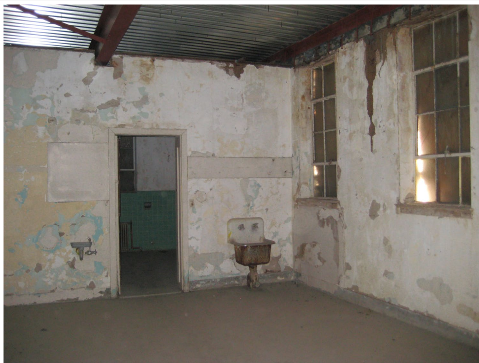
Elevation: Interior of secondary space Photographer: M. Schmitter
