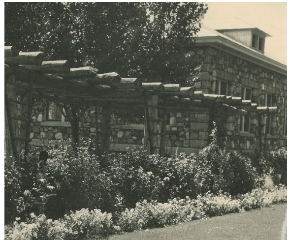
Stewart vernacular building with pergola covered walkway, ca. 1924, SISCC
