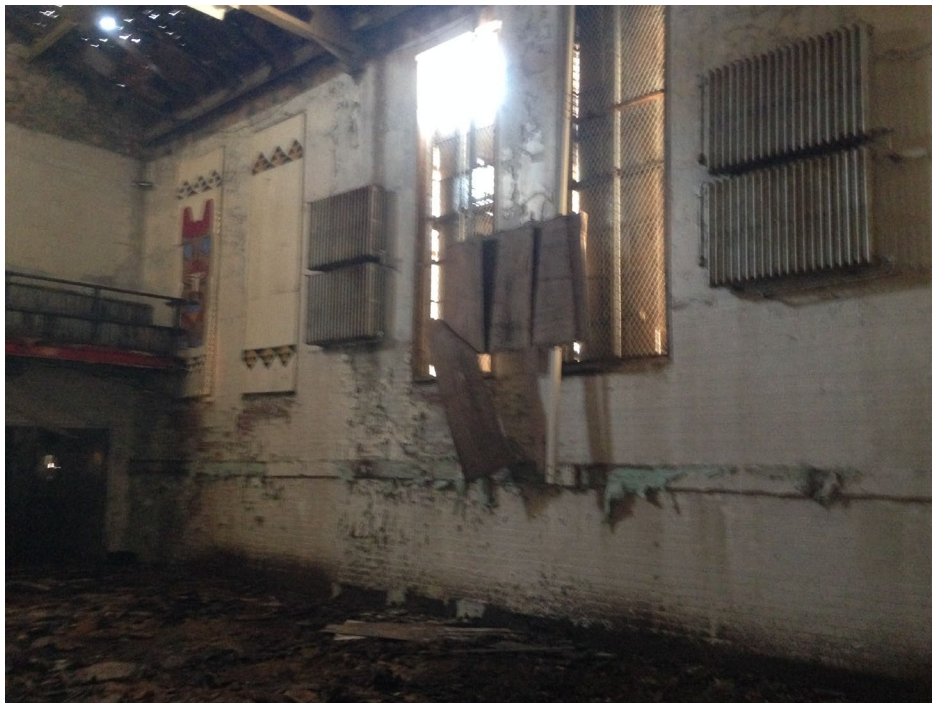
Elevation: Southeast corner, interior primary space Photographer: M. Schmitter
