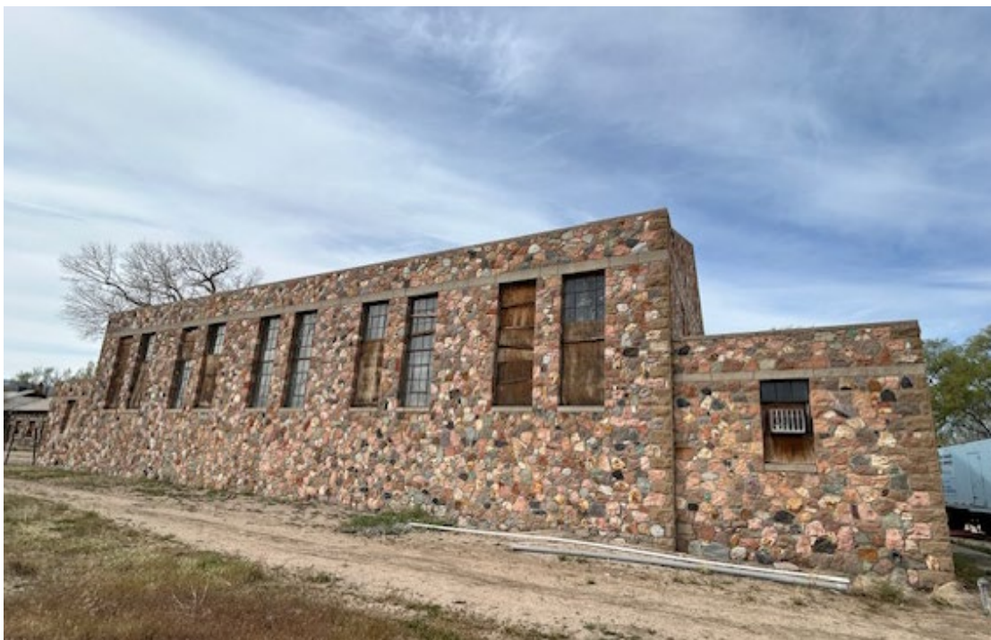
Elevation: South Photographer: M. Schmitter
