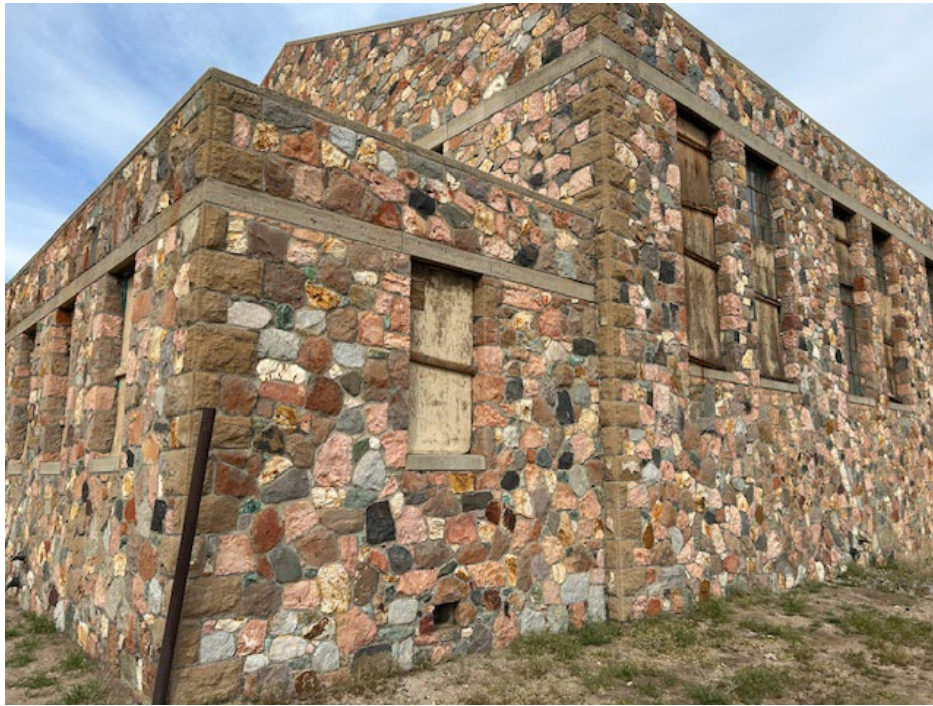
Elevation: South and partial west Photographer: M. Schmitter
