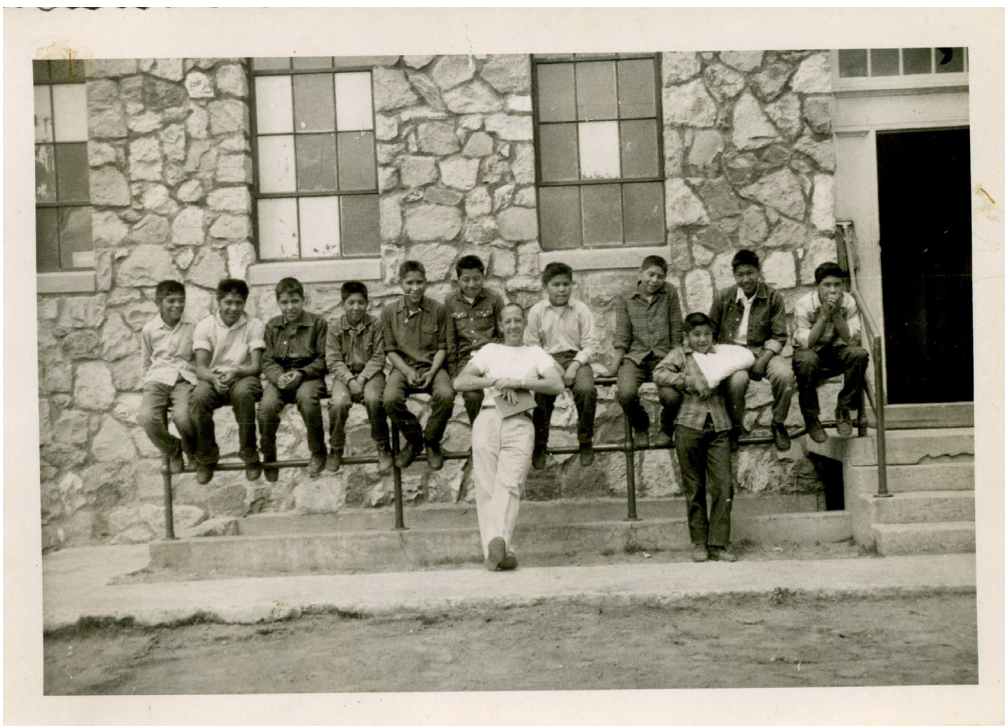
Elevation: East Close-up view of exterior stairs to partial basement, P.E. Class siting on metal railings Photographer: Howard Collett Collection at SISCC Date: 1953
