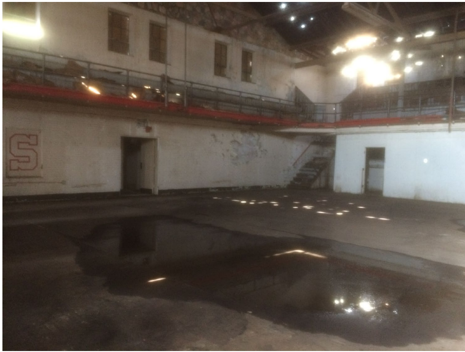
Elevation: Northwest corner, interior primary space
