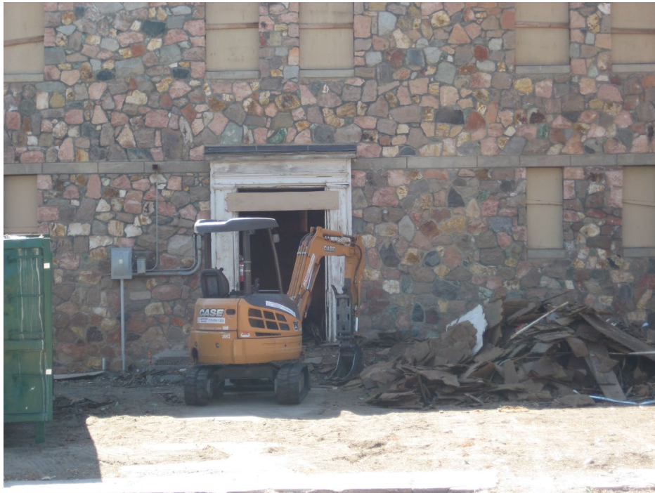
Elevation: North cleanup prior to roofing project
