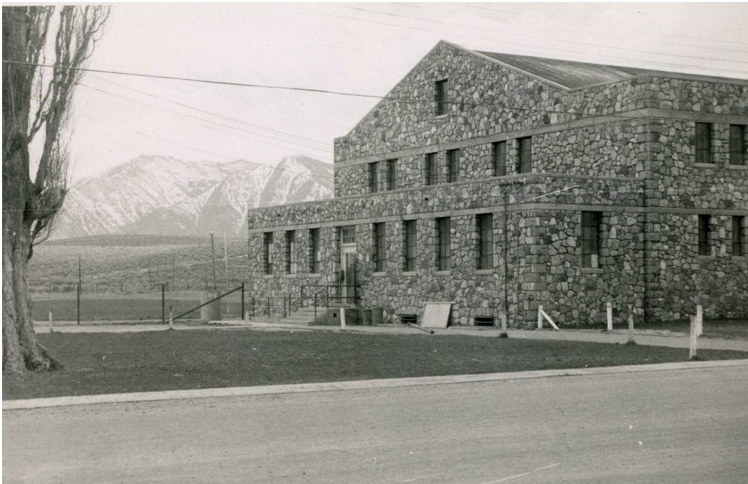
Elevation: East Direction facing: South Photographer: Howard Collett Collection, SISCC Date: ca. 1954
