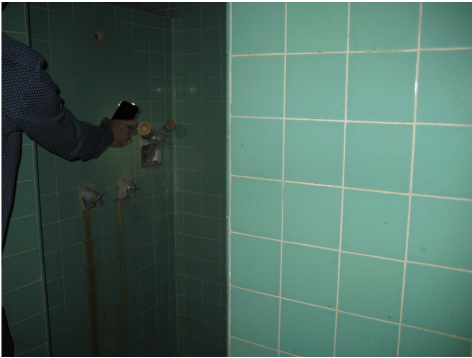
Elevation: Interior of secondary space Photographer: M. Schmitter
