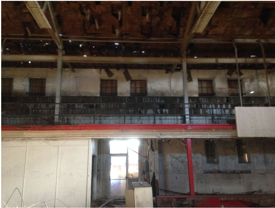
Elevation: Interior north elevation wall Photographer: M. Schmitter
