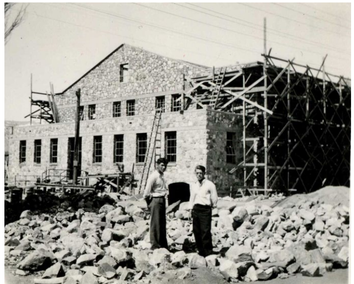
Construction of the gym is recorded in this historic photo from the Bob Wright collection (SISCC) dating to 1938. Note the piles of sand used to make the mortar and the stones for the walls.
