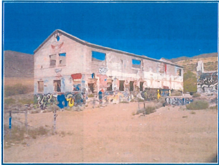
Figure 1-7 Building 6 – Precipitation and Refinery Building
