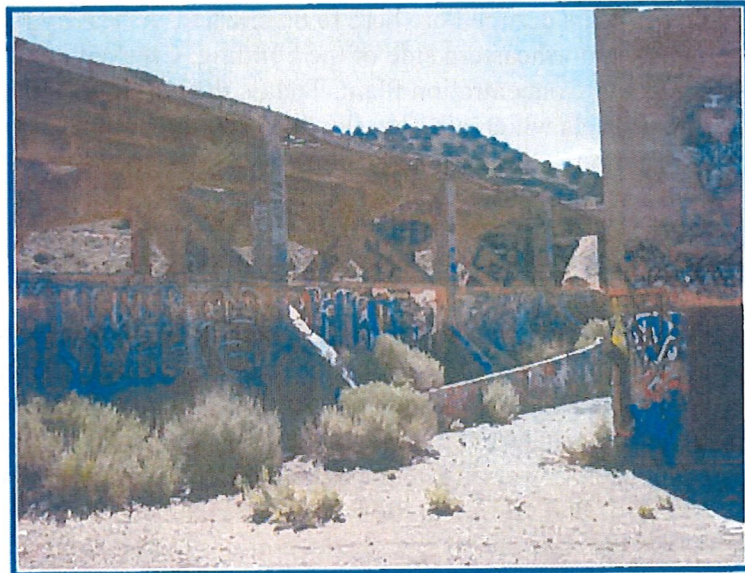
Figure 1-2 Building 1 – Ore Bin
