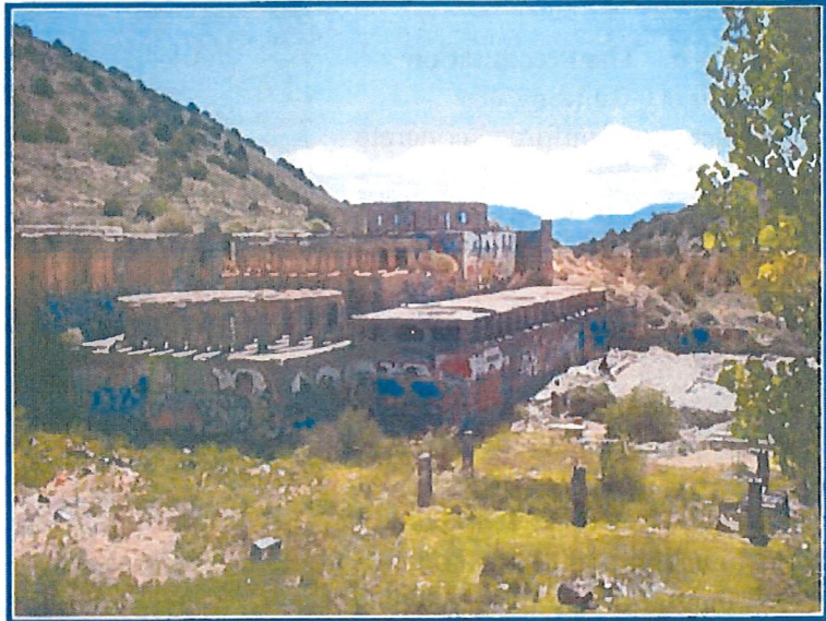
Figure 1-5 Building 4 – Cyanide Plant
