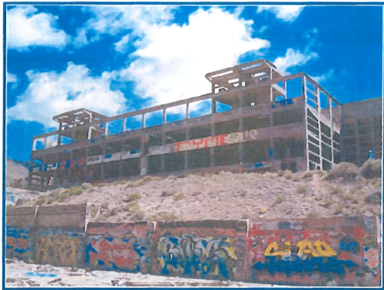
Figure 1-4 Building 3 – Fine Grinding and Concentration Plant
