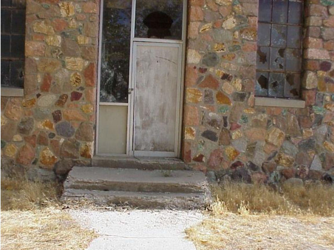
Figure 1: Front store front to be removed and replaced. The width once removed is 5'1".
