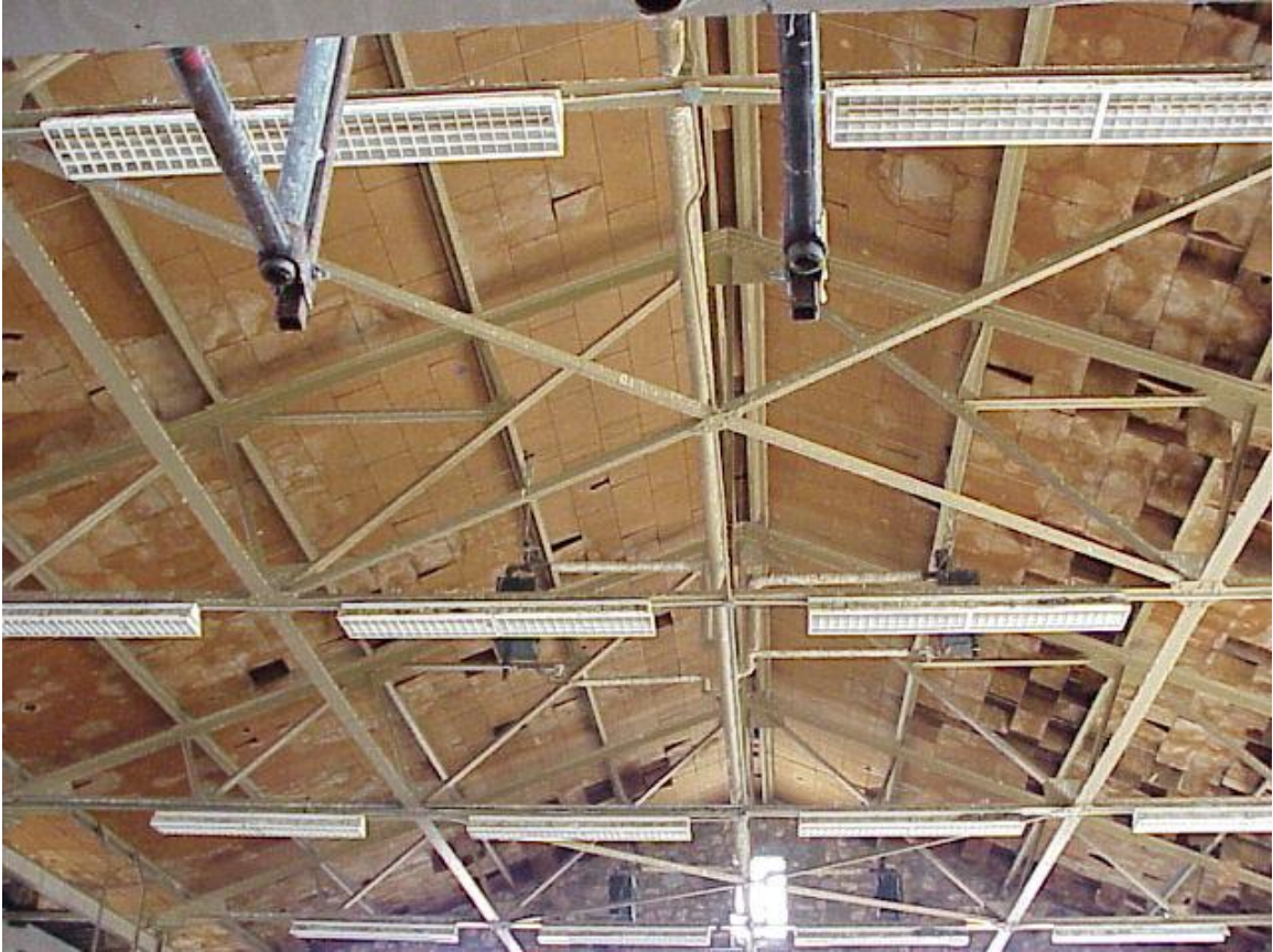
Figure 2: Ceiling tiles to be removed. This picture is 15 years old and 90% of the tiles have already fallen.
