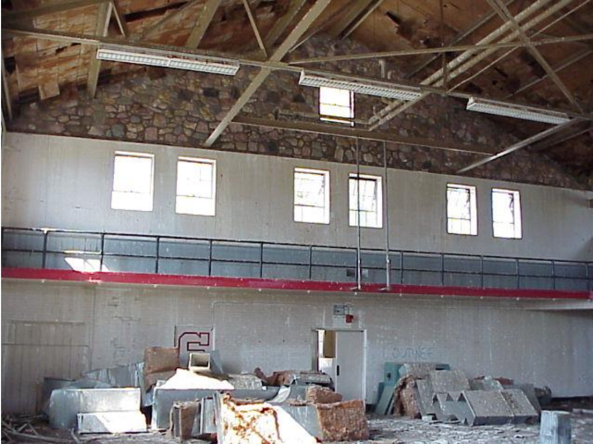
Figure 4: Miscellaneous debris. This is a 2001 picture, but the material is still in place covered with fallen ceiling tiles.
