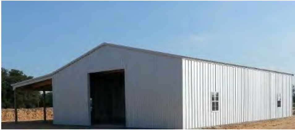
Example – showing vertical galvalume siding and vinyl windows. (The proposed garage will not have this shed-roofed side porch.)
