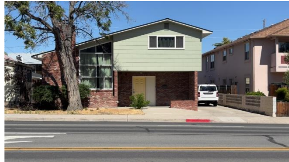
Figure 13: A Contemporary style home at 78 Keystone Avenue.
