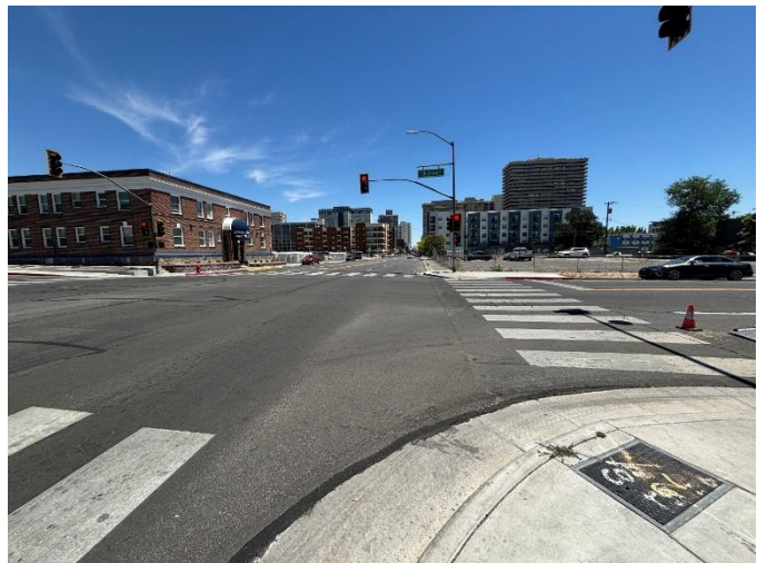
Figure 4: Facing east at the intersection of West Second and Ralston streets.
