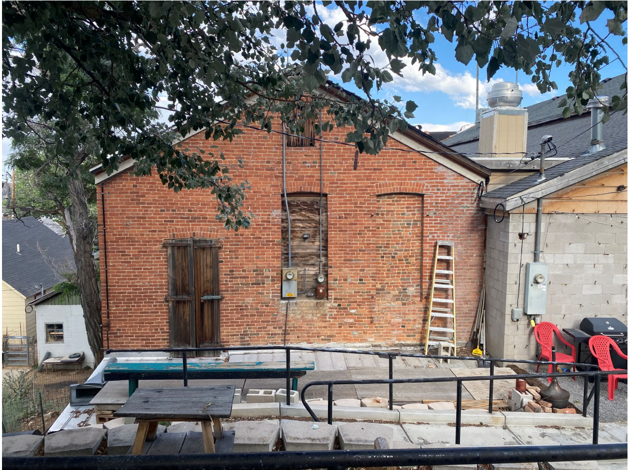
Photograph 17: Rear (west) elevation gable end looking east from the rear of the property. View shows brick masonry construction, gable end roof form, shuttered second-story doorway providing access to the upper level from the rear of the building, infilled opening with segmental brick arch, and utility service installations associated with the historic rear elevation. Photograph by Audie Robinson. Photographed July 14, 2026.
