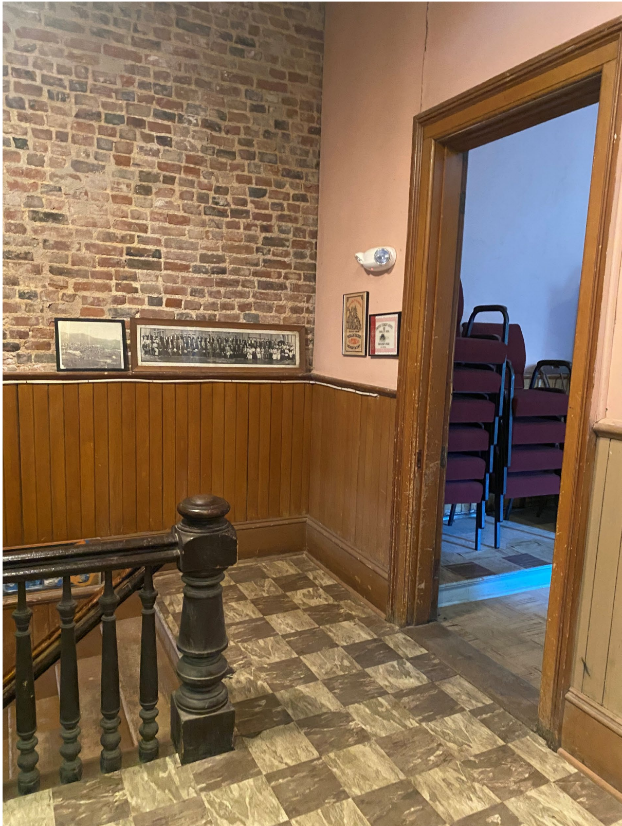
Photograph 5. Second-floor landing looking northeast. View shows original stair landing and balustrade, exposed brick masonry wall, vertical board wainscoting, plaster walls, and doorway opening into the adjacent meeting room. Photograph by Audie Robinson. Photographed July 14, 2026.
