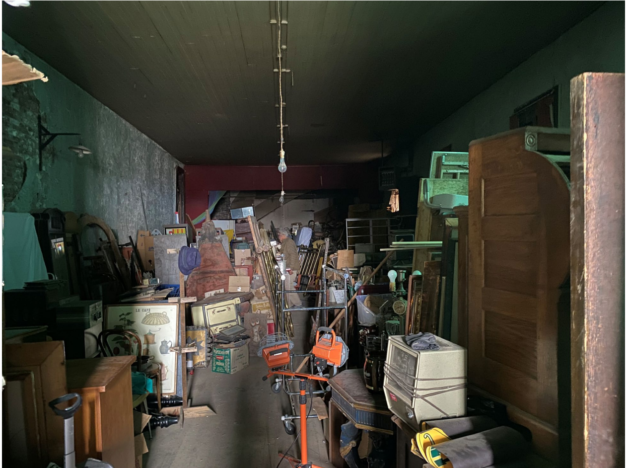
Photograph 2: First floor Assembly Hall looking west toward the stage. Room is currently leased for storage. View shows the open assembly space, tongue-and-groove ceiling, early electrical conduit and lighting, and surviving historic spatial organization. Photograph by Audie Robinson. Photographed October 18, 2025.
