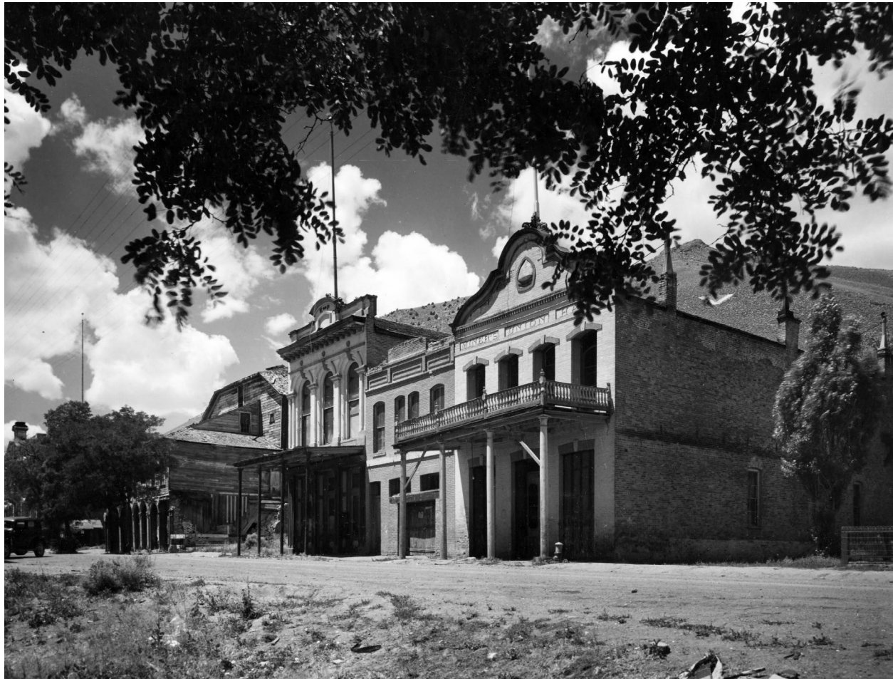
Figure 11. Miners' Union Hall, Virginia City, Nevada, north and east elevations, photographed by Josef Muench in the 1930s. Courtesy of the Utah State Historical Society.
