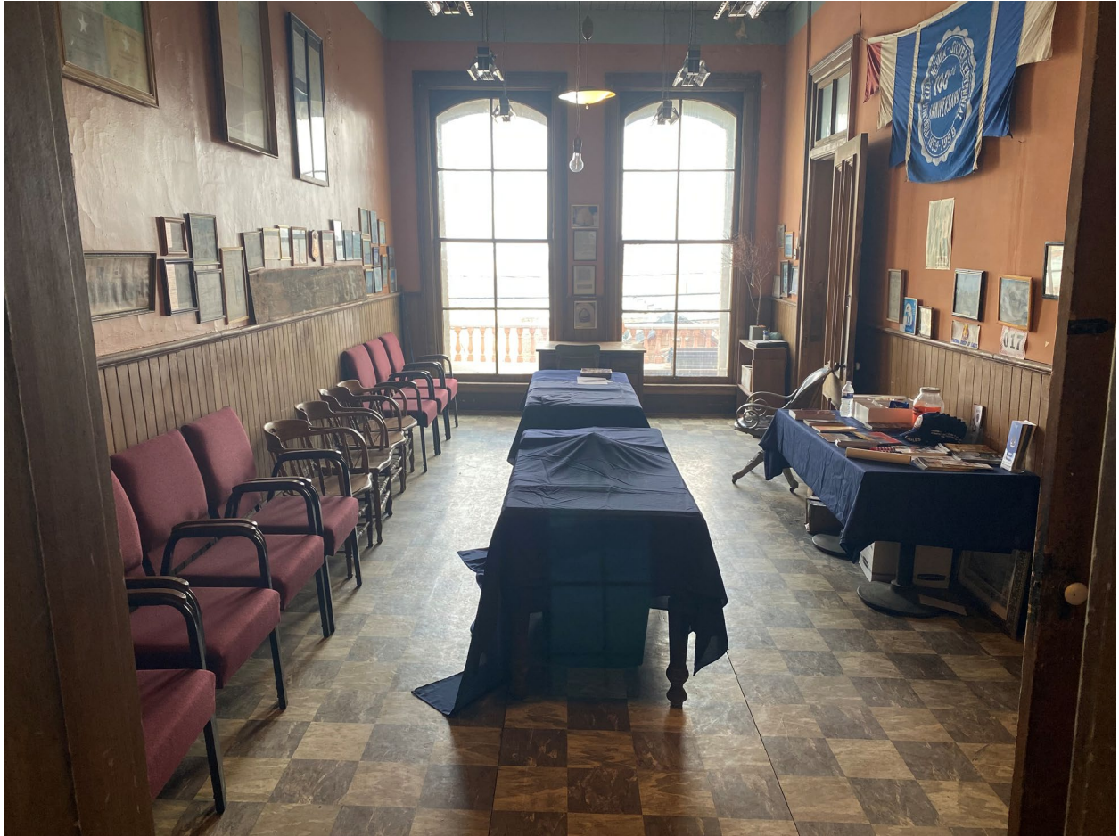
Photograph 8: Second-floor exhibit room looking east toward the balcony windows overlooking B Street. View shows wood wainscoting, plaster walls, wood flooring, historic window openings, and exhibit space adjacent to the Main Hall assembly room. Photograph by Audie Robinson. Photographed July 14, 2026.
