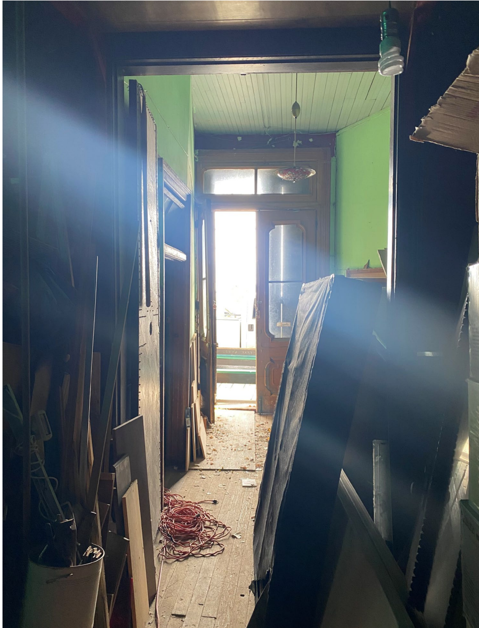
Photograph 3: First floor. Entrance vestibule looking east toward North B Street and the primary entrance. Note the historic entry doors, transom windows, wood flooring, and surviving millwork and trim. Photograph by Audie Robinson. Photographed October 18, 2025.
