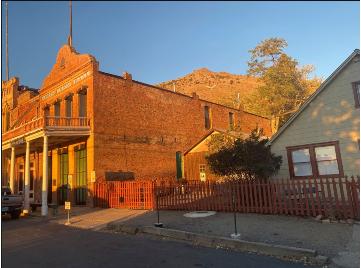
Photograph 16: North elevation of the Miners' Union Hall, looking southeast from the sloping ground north of the building. View shows the brick masonry construction, the relationship of the building to the surrounding topography, and the neighboring buildings along the north side of the property. Photograph by Audie Robinson, October 1, 2026.
