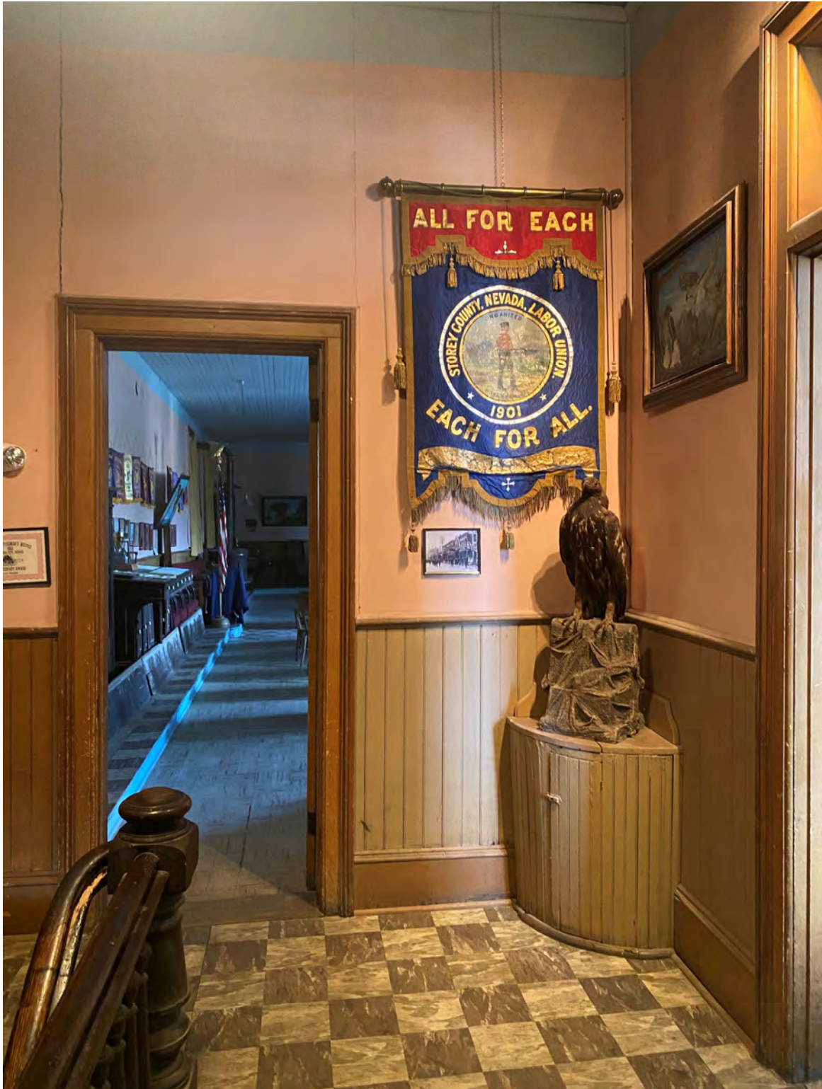
Photograph 6. Second-floor entry hall looking west into the Main Hall. View shows wood wainscoting, plaster walls, transomed doorway opening, and circulation between the stair landing and Main Hall assembly space. Photograph by Audie Robinson. Photographed July 14, 2026.
