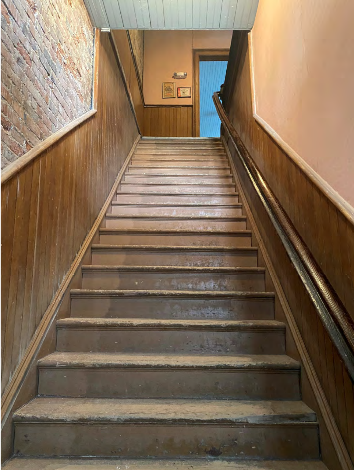
Photograph 4. First-floor main stair looking north toward the second-floor landing. View shows original wood stair assembly with wood treads and risers, wood handrail, vertical board wainscoting, plaster walls, exposed brick masonry wall, and tongue-and-groove ceiling above the landing. Photograph by Audie Robinson. Photographed July 14, 2026.
