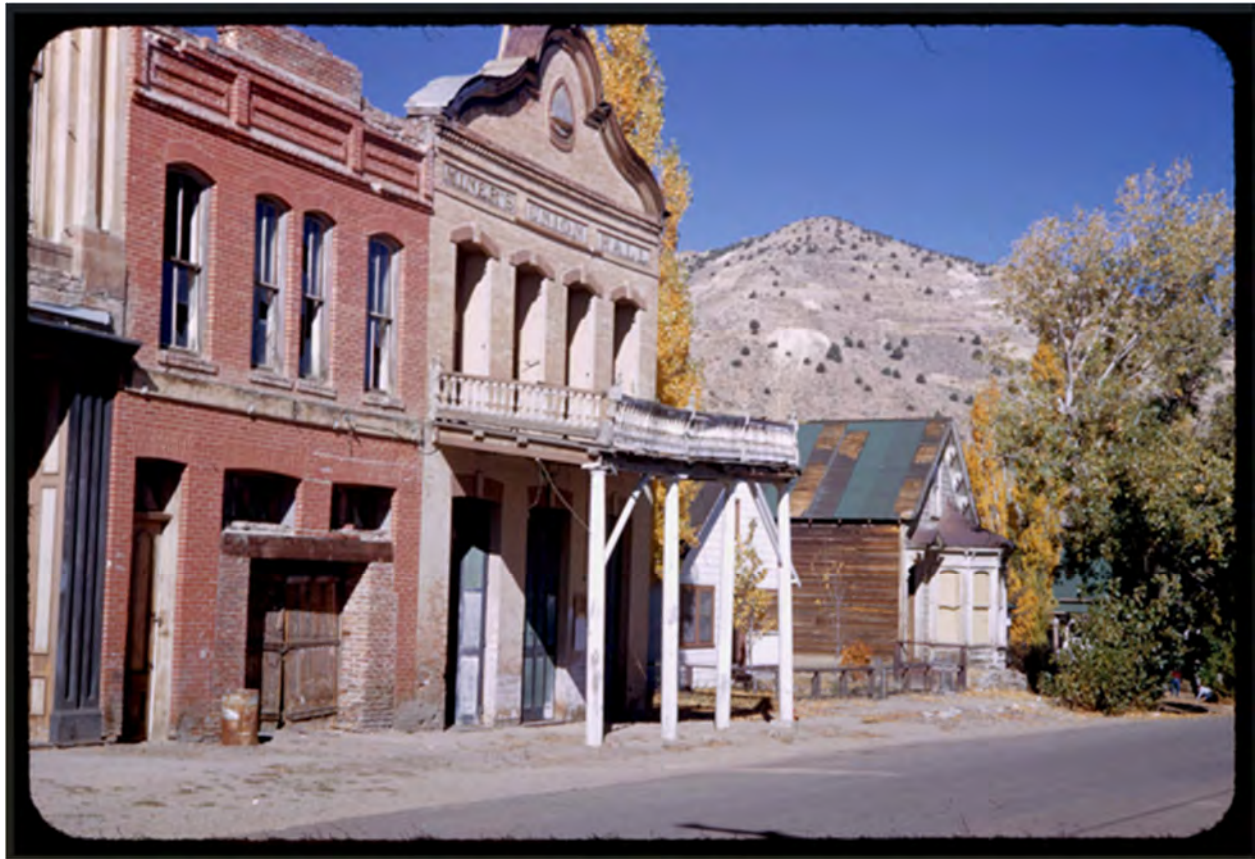
Figure 12. Miners' Union Hall, Virginia City, Nevada, north and east elevations, photographed in 1952 by Charles Cushman. Courtesy Indiana University
