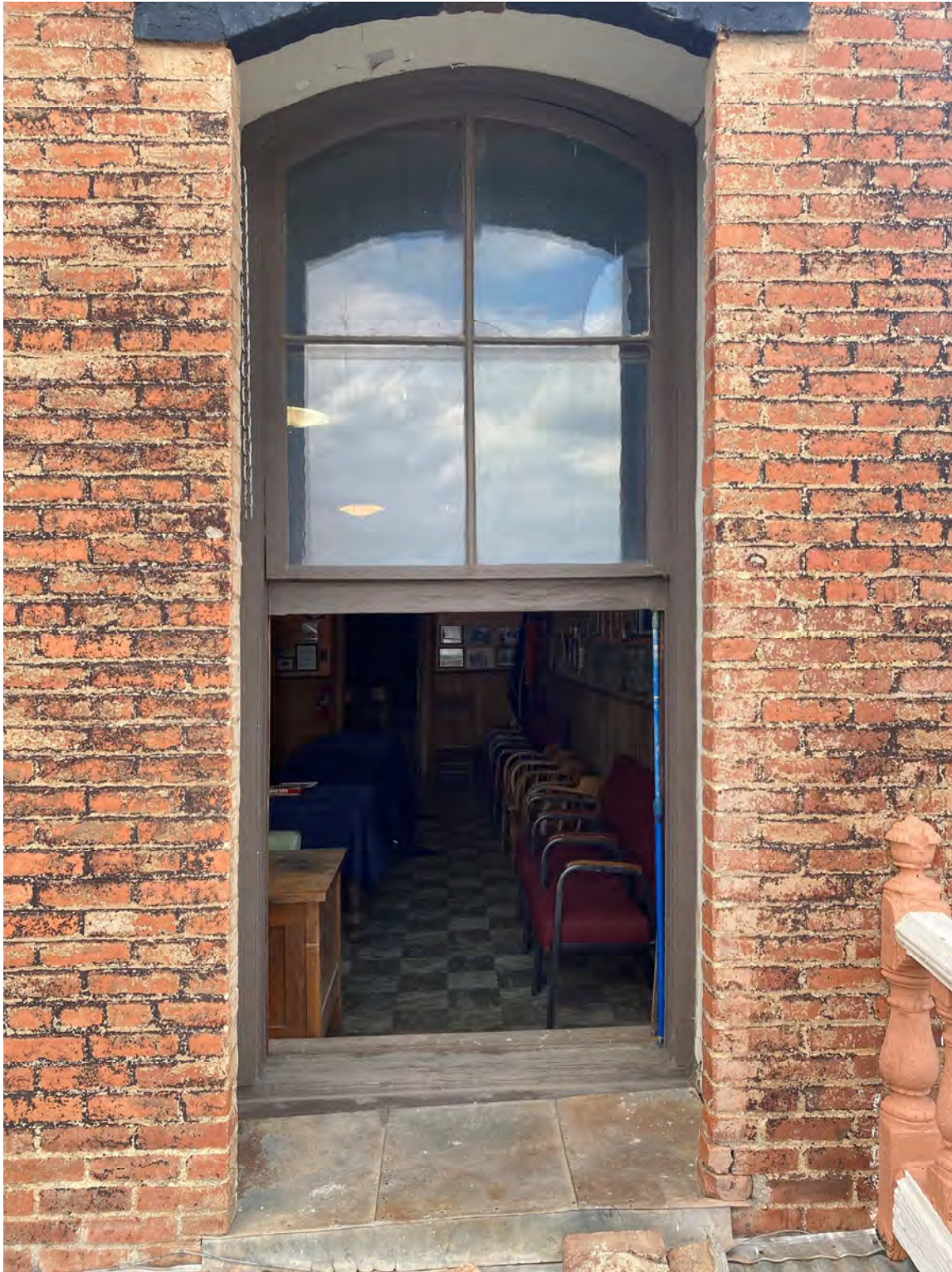
Photograph 9. Second-floor front elevation window looking west into the second-floor exhibit room from the exterior balcony. View shows the segmental arched masonry opening, wood window frame and sash, and relationship between the exterior balcony and second-floor exhibit room. Photograph by Audie Robinson. Photographed July 14, 2026.
