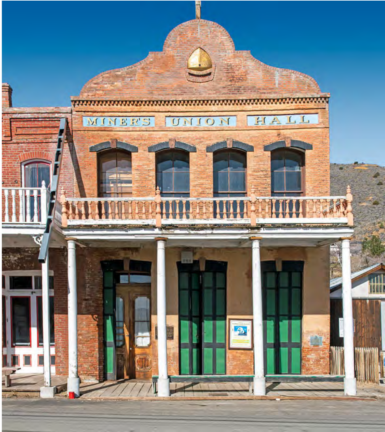
Photograph 1. Primary east facade looking west from North B Street. View shows the two-story brick institutional building with curvilinear parapet, painted "MINERS UNION HALL" sign panel, four segmental-arched, two-part commercial second-story window openings, full-width second-story balcony with turned balustrade, one-story porch supported by wood columns, and storefront openings at street level. Photograph by Audie Robinson. Photographed October 18, 2025.
