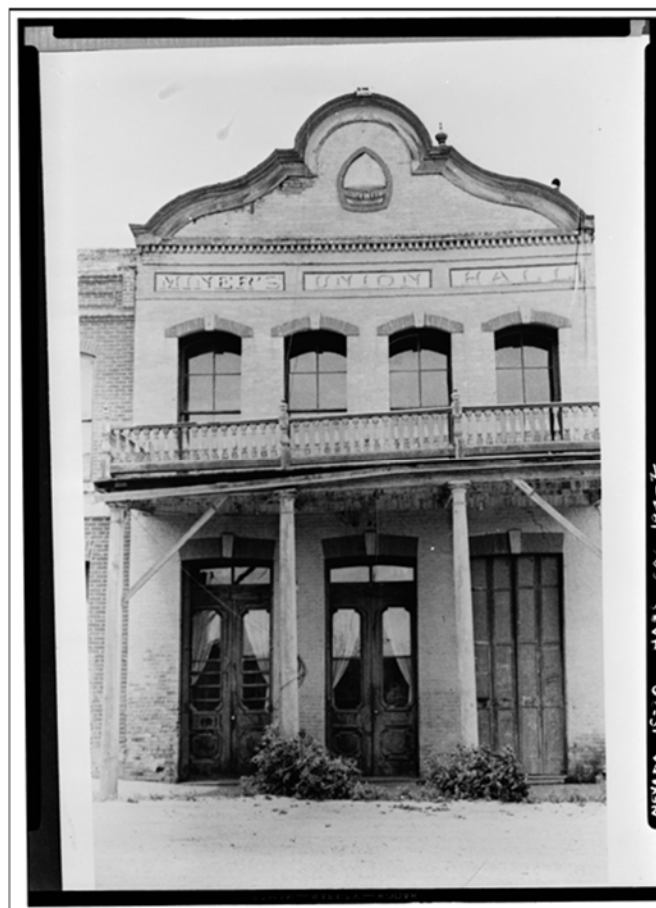
Figure 10. Miners' Union Hall, Virginia City, Nevada, east elevations, photographed in 1940 by Robert W. Kerrigan. Courtesy of the Library of Congress.
