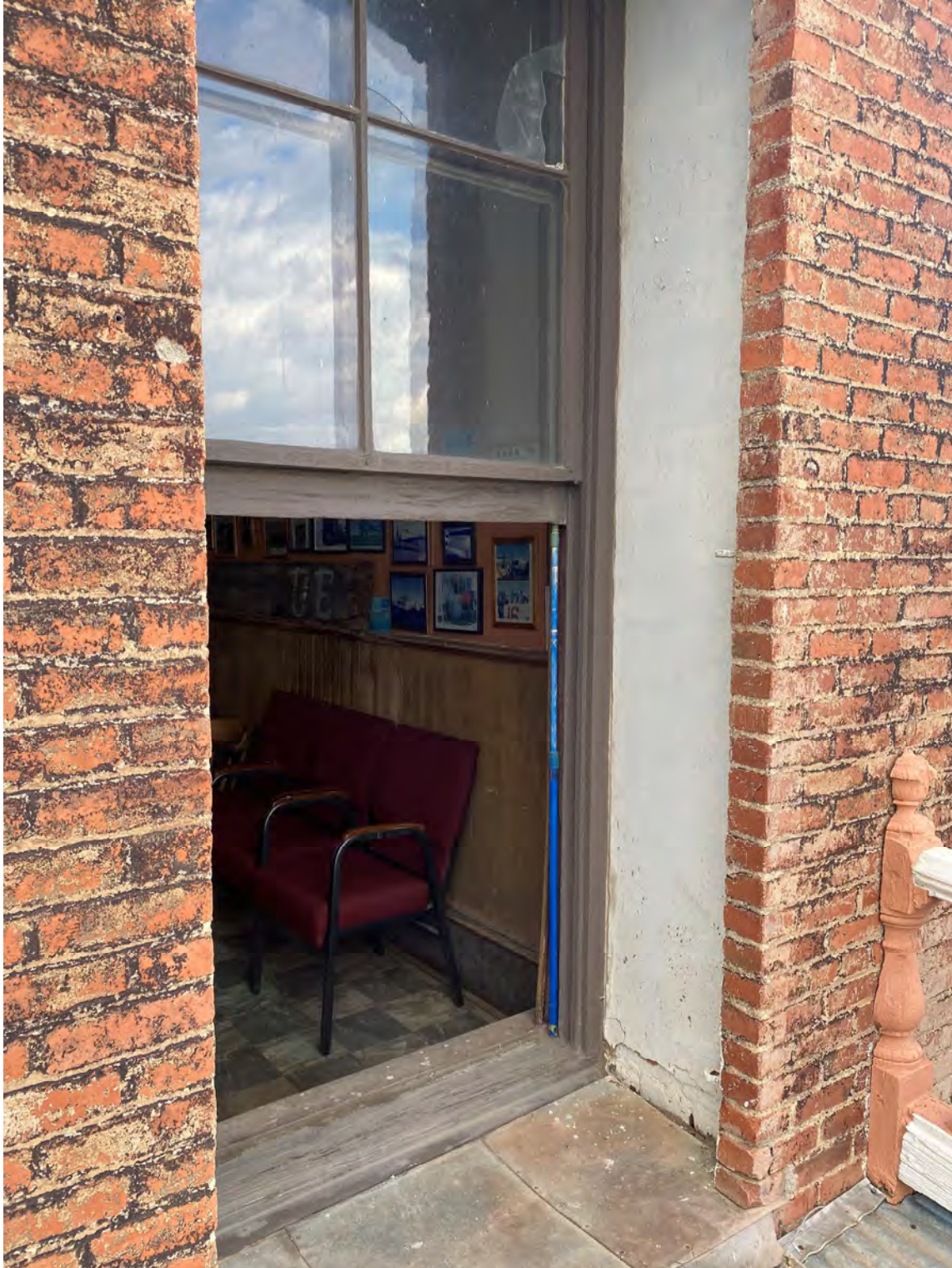
Photograph 10. Oblique view of the north second-floor front elevation window looking northwest from the exterior balcony. View shows the relationship between the exterior balcony, masonry wall, wood window frame and sash, and second-floor exhibit room. Photograph by Audie Robinson. Photographed July 14, 2026.
