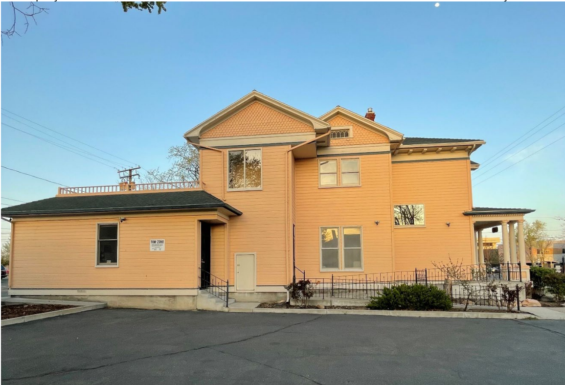
Photo 2 of 6: West elevation facing east. The home's two-story Queen Anne massing is still evident. The 1980s single-story addition for office space is at the far left.
