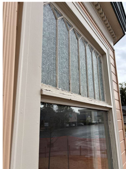
Figure 2: Special window in first-floor bay with textured glass upper sash. Photo credit: Melissa Hafey 10/02/2025.
