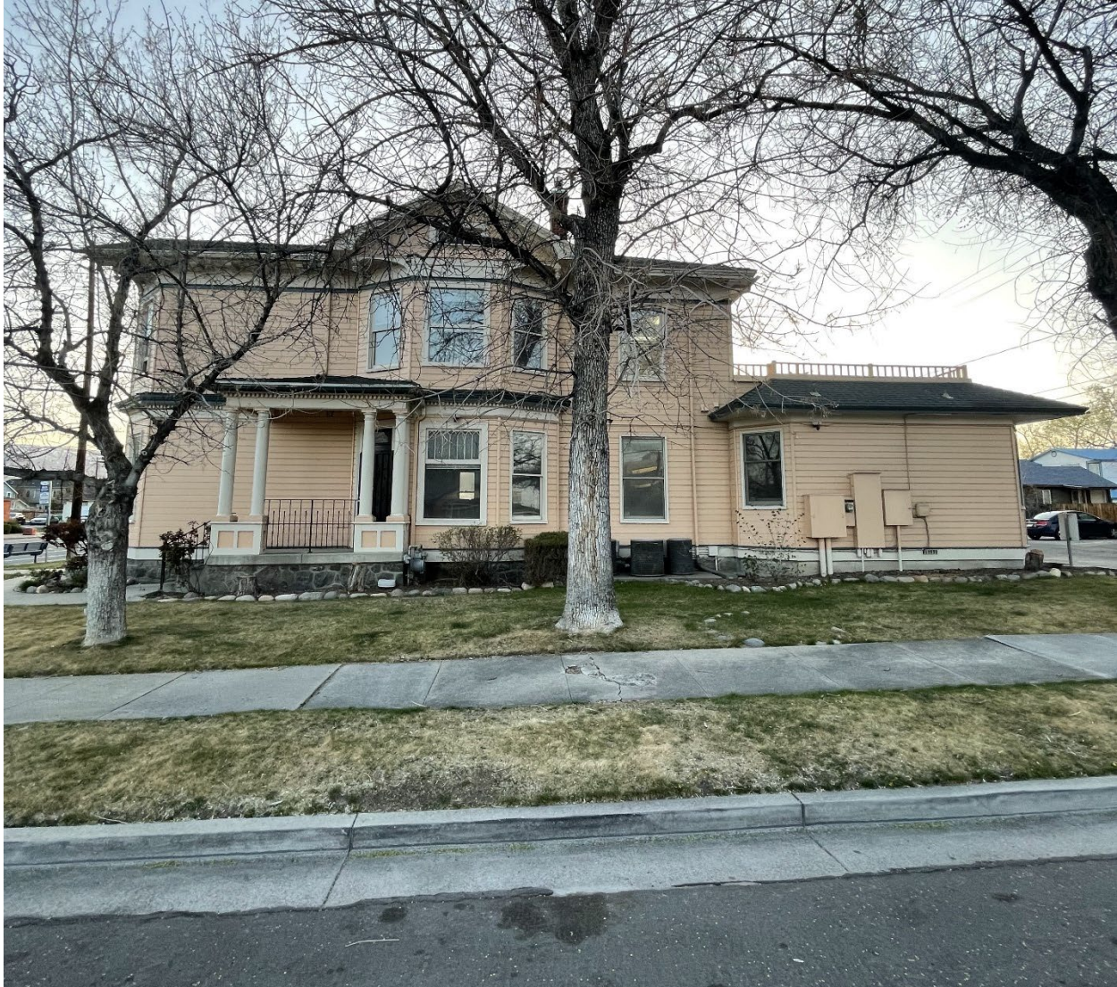
Photo 3 of 6: East elevation facing west. The home's original two-story Queen Anne massing has been preserved. The one-story addition is to the right.
