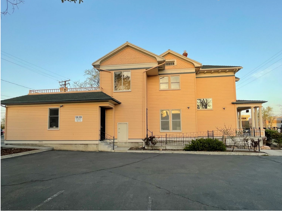
Photo 2 of 4: West elevation facing east. The home's two-story Queen Anne massing is still evident. The 1980s single-story addition for office space is at the far left.
