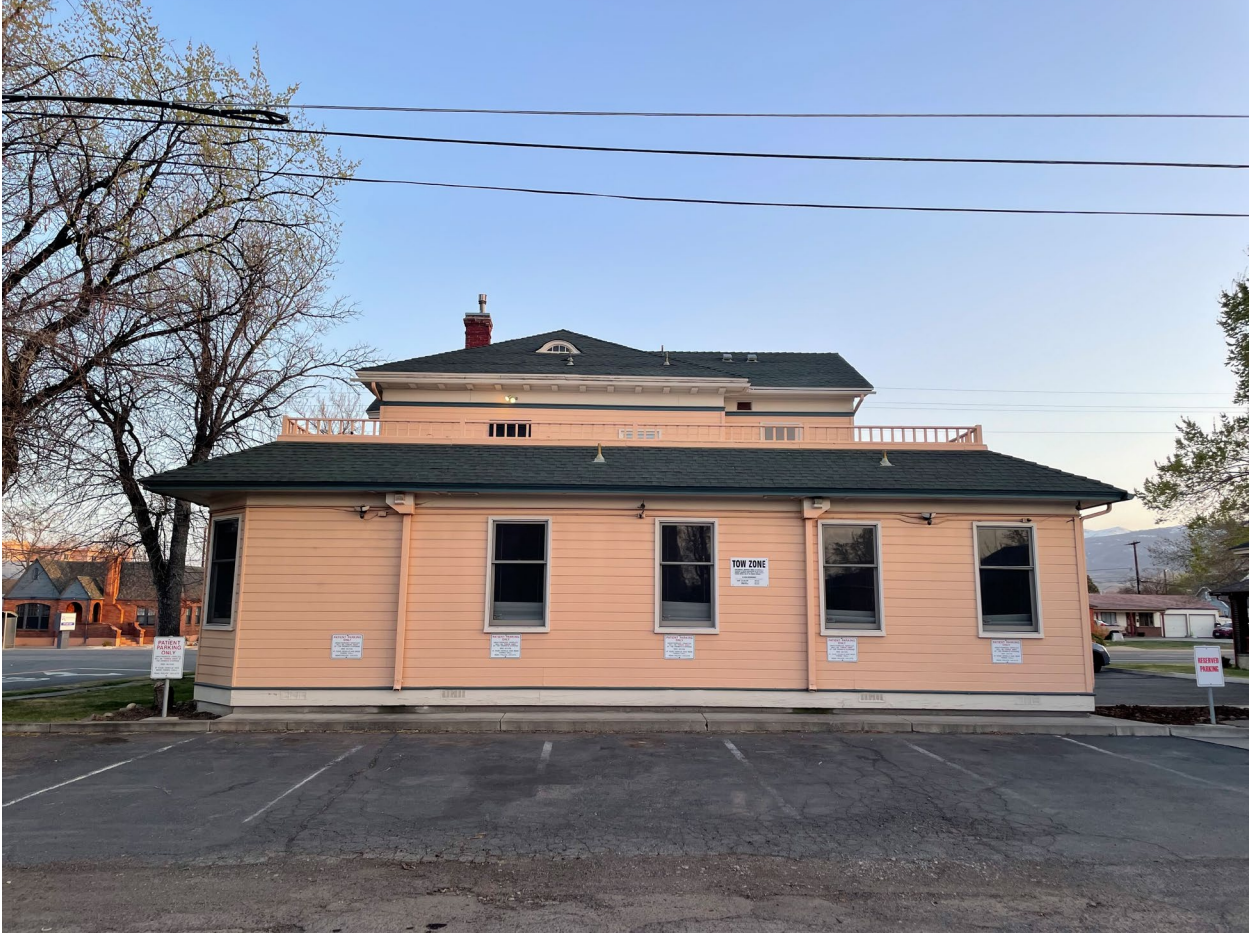
Photo 4 of 4: Rear elevation facing south. The 1980s first-floor addition is in the foreground, while the original home's second floor and eyebrow window are still visible.
