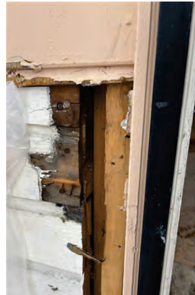
Figure 7: Original shiplap cladding under a newer layer of siding. Photo credit: Melissa Hafey 10/02/2025.
