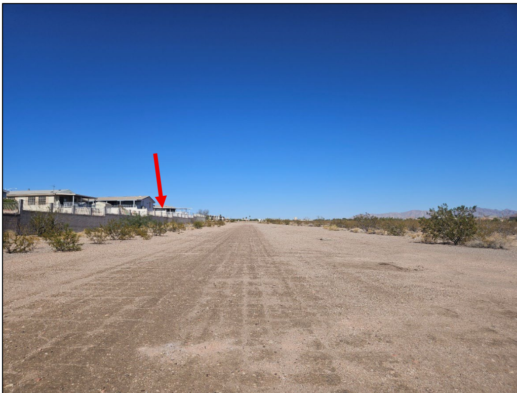
Photograph 7: (NV_Clark_Boulder City Navy Hangar_0007) Overview of Runway 3/21 from northeast of Aspen Drive, facing northwest. Navy Hangar is located on the north of the runway (not visible), depicted by the red arrow.
