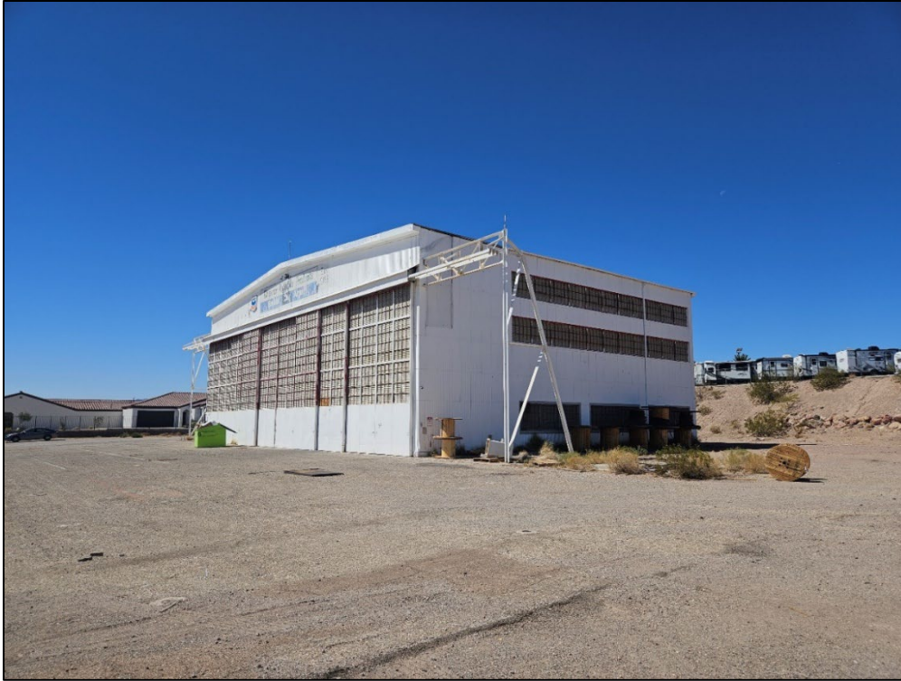
Photograph 2: (NV_Clark_Boulder City Navy Hangar_0002) North and primary facades, facing east. Compare to north historic photograph in Figure 7.
