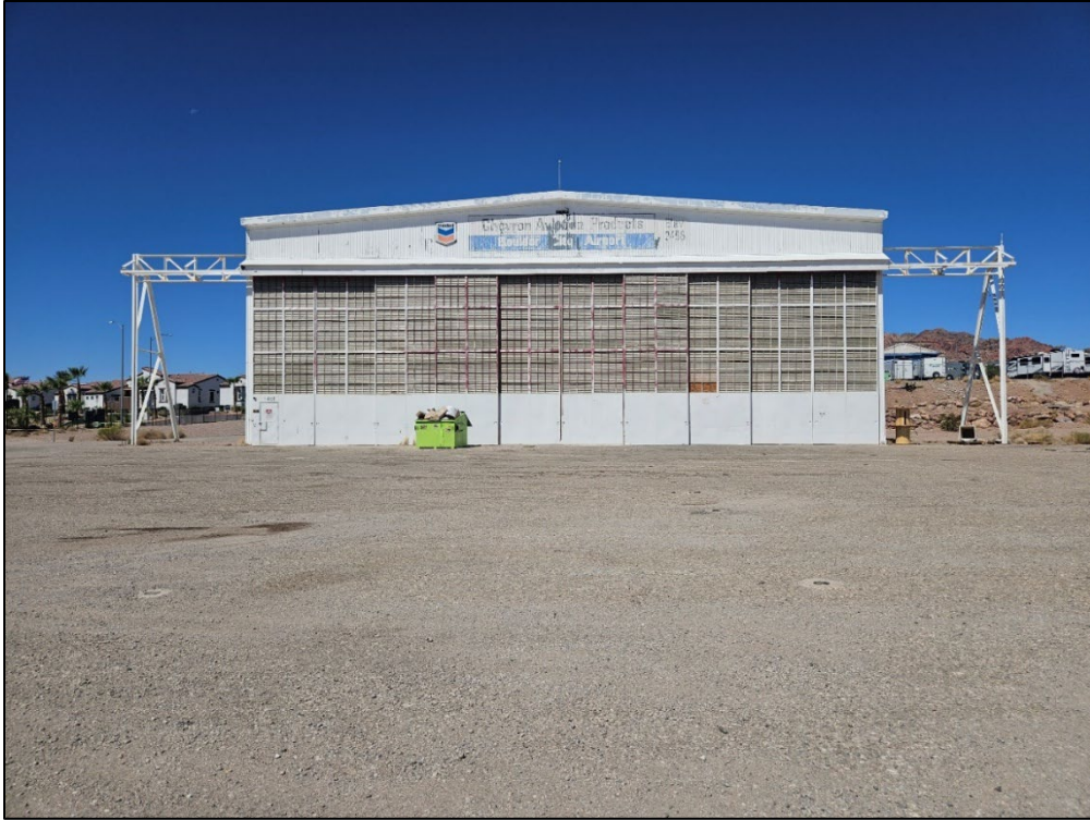
Photograph 1: (NV_Clark_Boulder City Navy Hangar_0001) Primary façade of Navy hangar, facing northwest.
