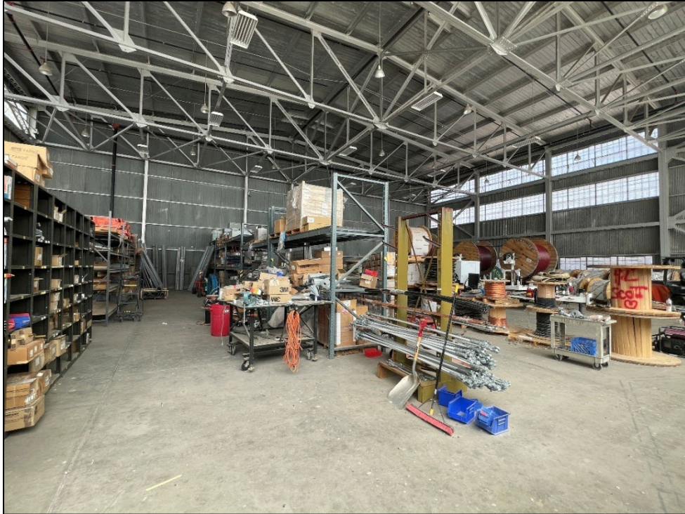
Photograph 5. (NV_Clark_Boulder City Navy Hangar_0005) Interior of Navy Hangar, facing north.
