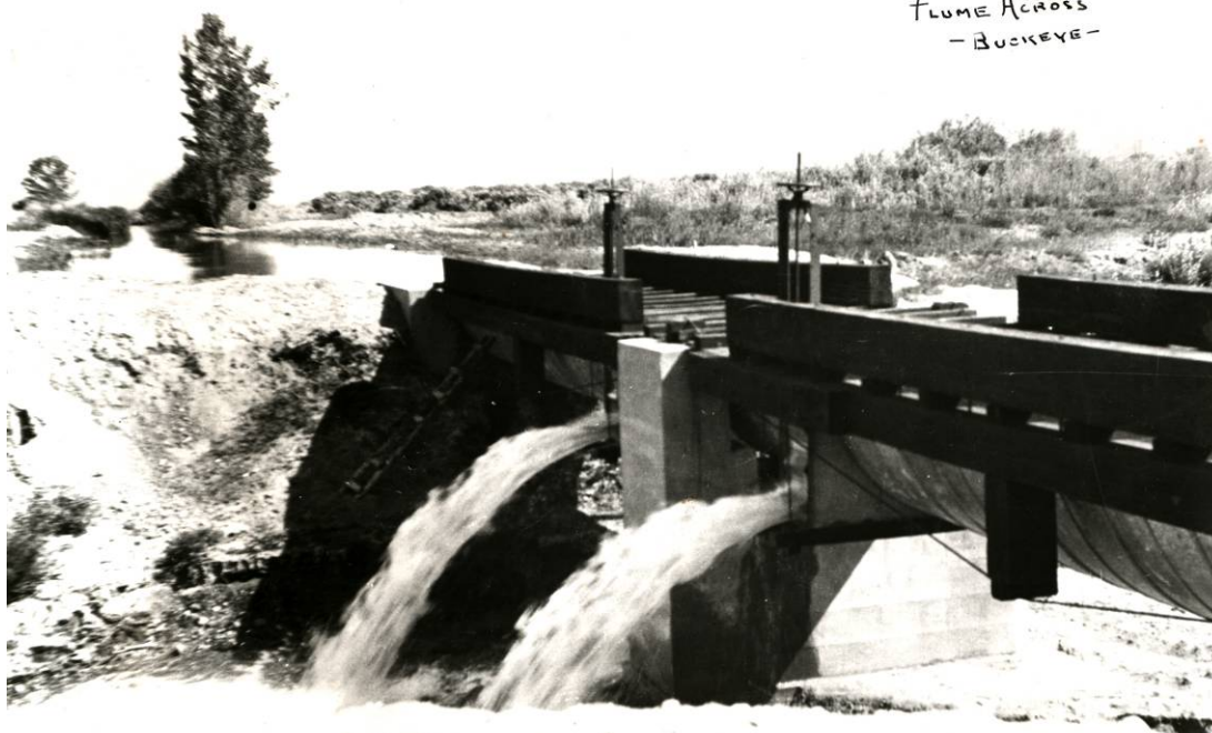
Ditch flume over Buckeye Creek in Carson Valley. The flume allows appropriated water from the ditch to flow over the bed of Buckeye Creek, keeping the two waterways separate. This flume is likely for either the Allerman or Lower Old Virginia Canal. No date. Courtesy of Douglas County Historical Society.
