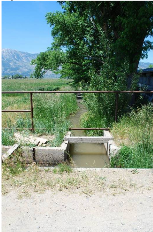
A diversion box and culvert (left) and distribution ditch (right) on the Stodieck ranches near Waterloo, Nevada SHPO, June 7, 2016.
