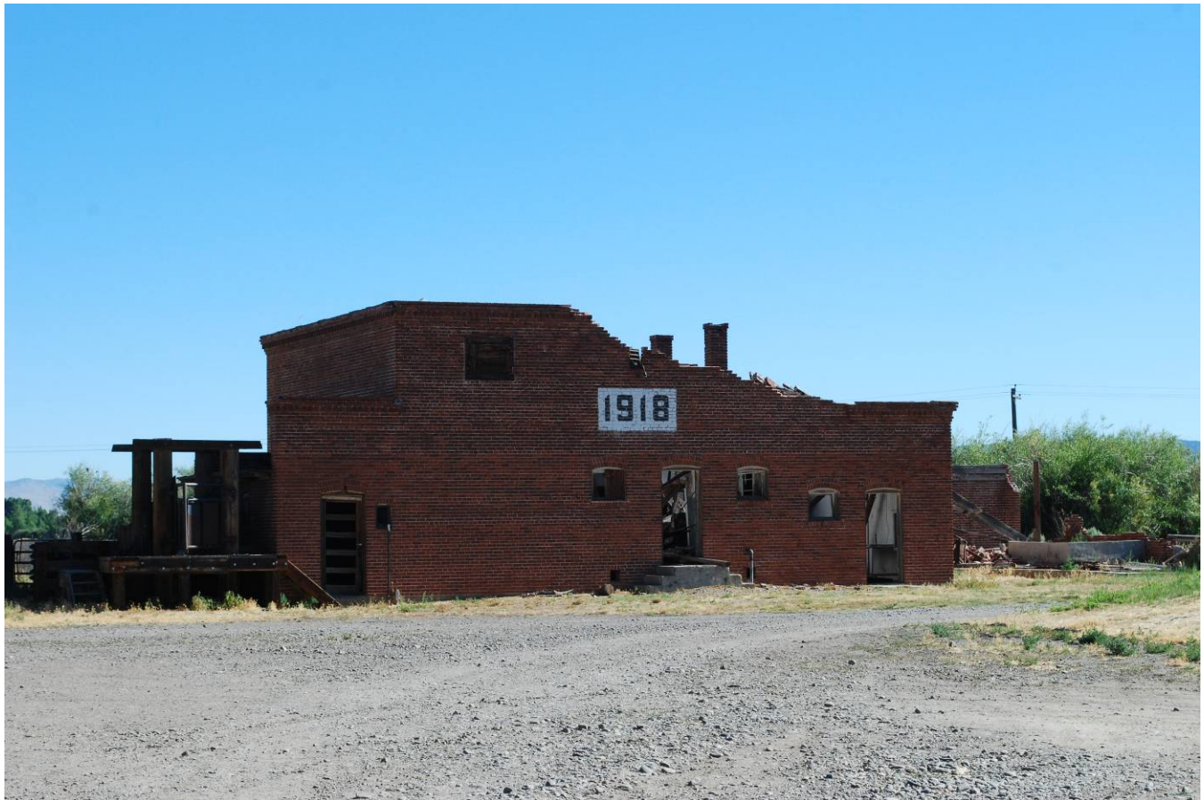
Slaughterhouse at the Dangberg Home Ranch. Built between 1915 and 1916, this was possibly the largest such facility in the region. The roof was damaged prior to 1980 but has not been repaired, leading to the current deterioration. Nevada SHPO, July 22, 2016.
