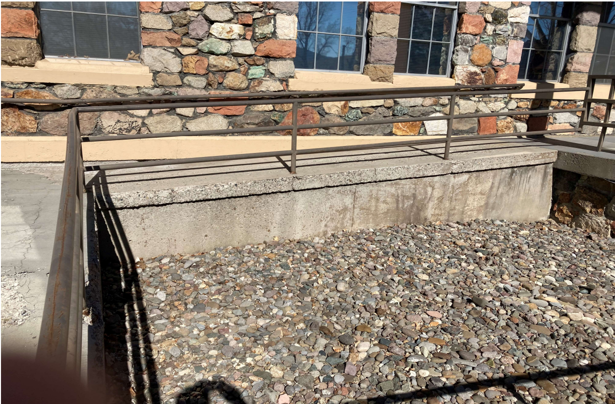
East Ramp Upper Level
