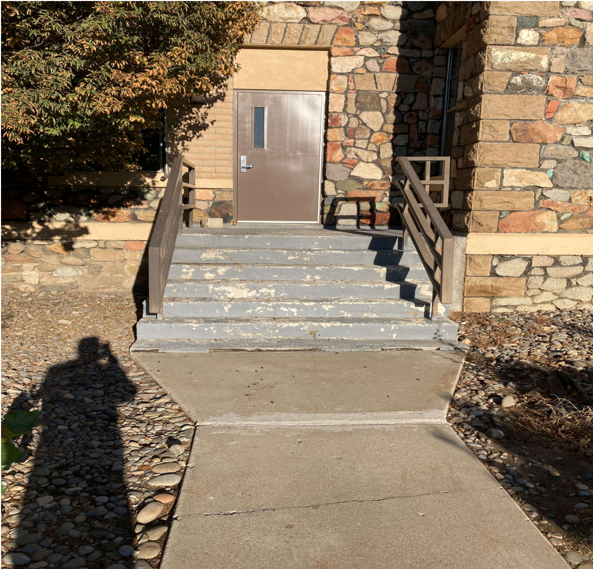
Northeast Building Entrance Stairs
