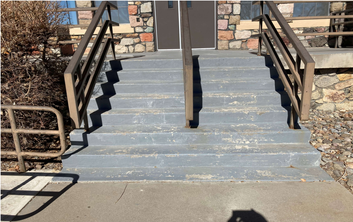
East Building Main Entrance Stairs
