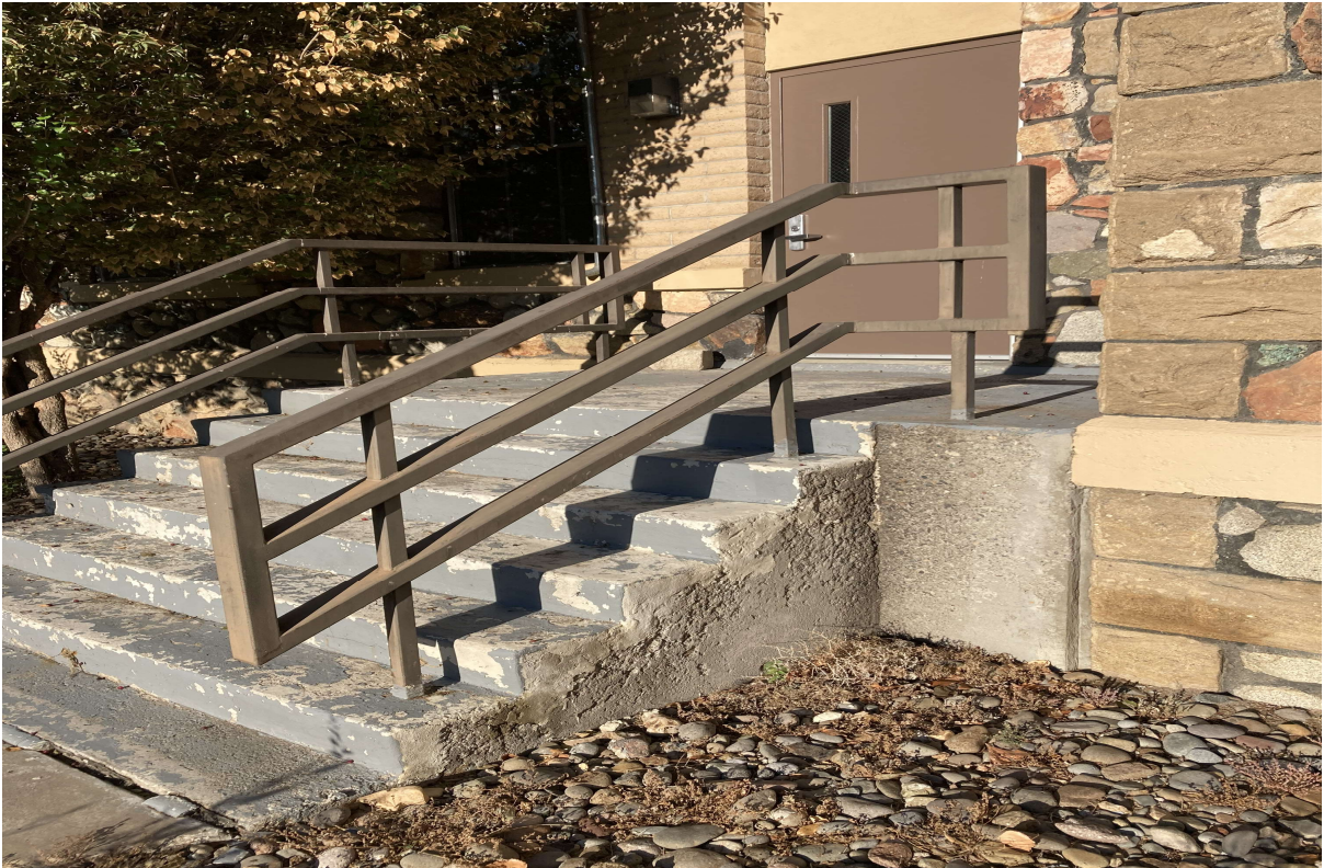
Southeast Building Entrance Stairs
