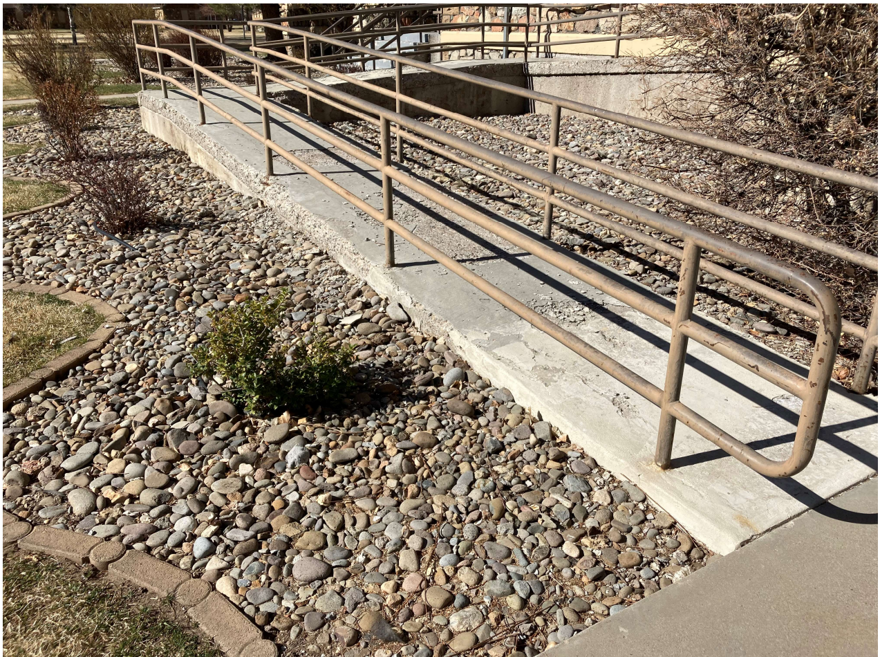
East Ramp Lower Level
