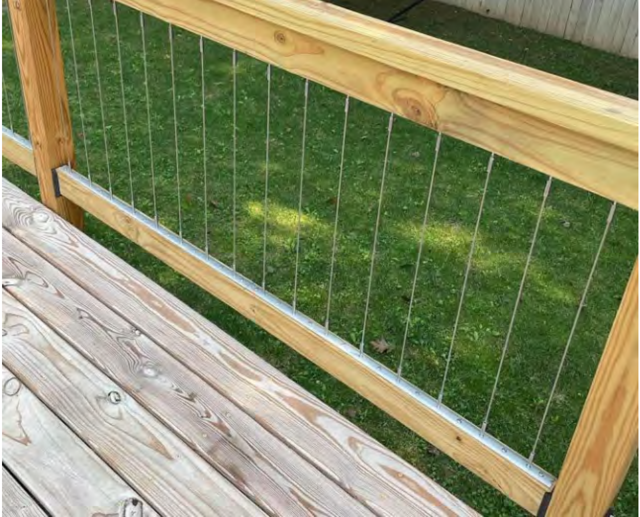
The type of thin cable to be installed between each baluster
