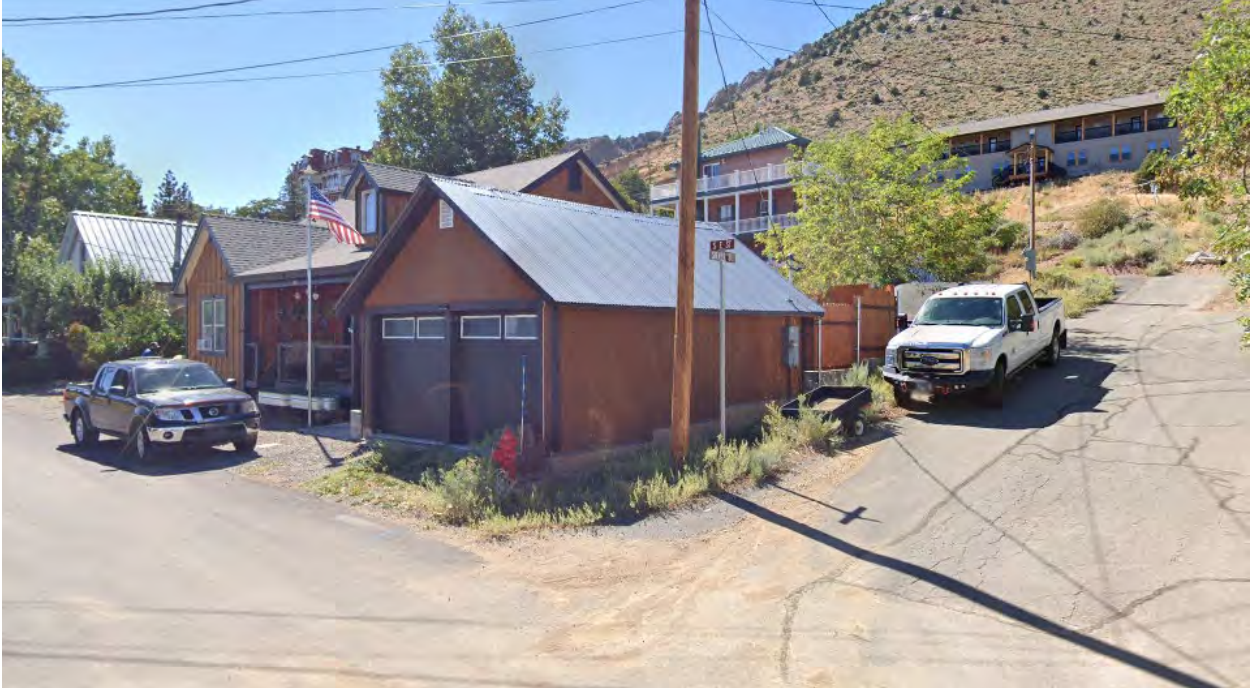
View from E Street
