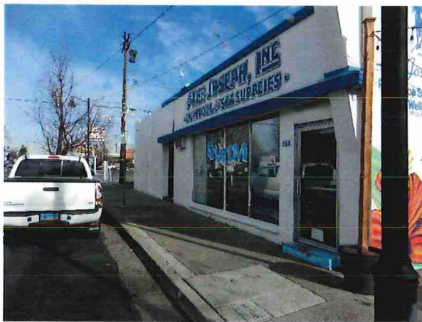
Photo 3: Lee Joseph, Inc. 864 S Wells Ave
