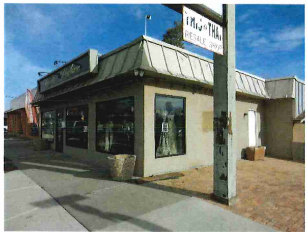
Photo 8: Party Palace, 1090 S Wells Ave
