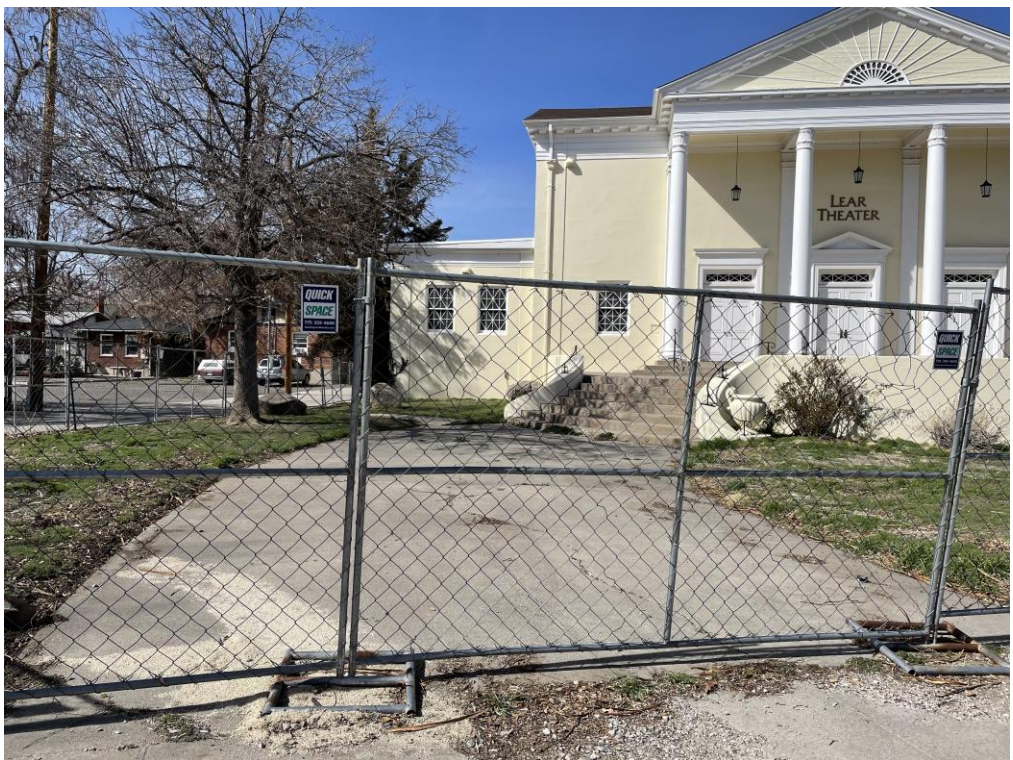
Front (south) facade, left sidewalk and stairs up to main entrance.
