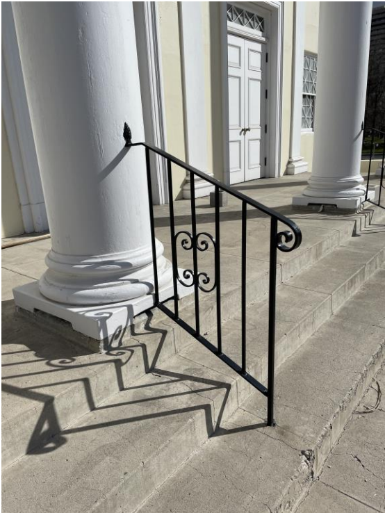
View of existing railings on south facade, main entrance.
