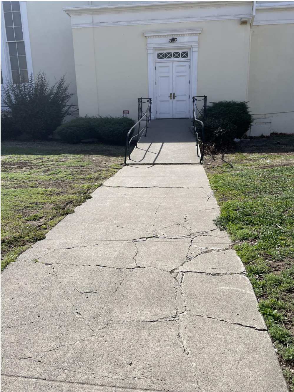
East facade with existing ramp and entrance.
