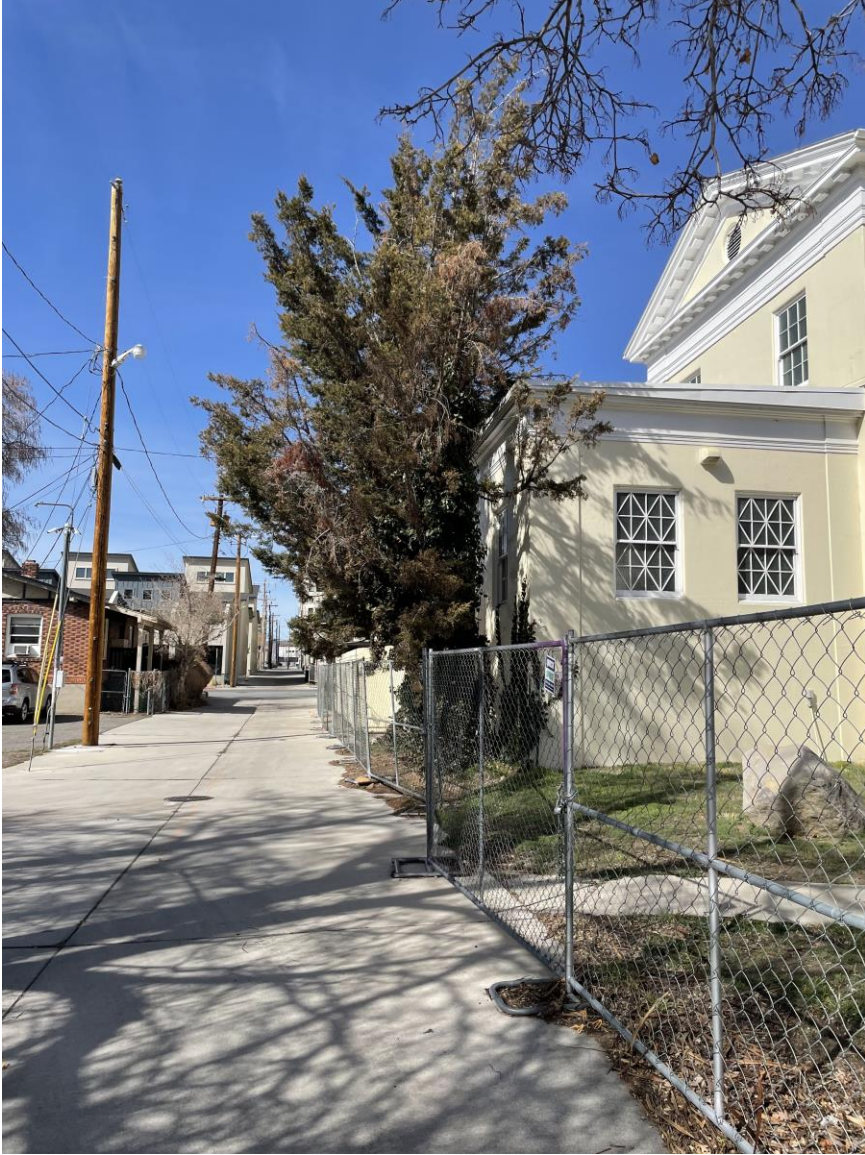
View of west facade, facing north.
