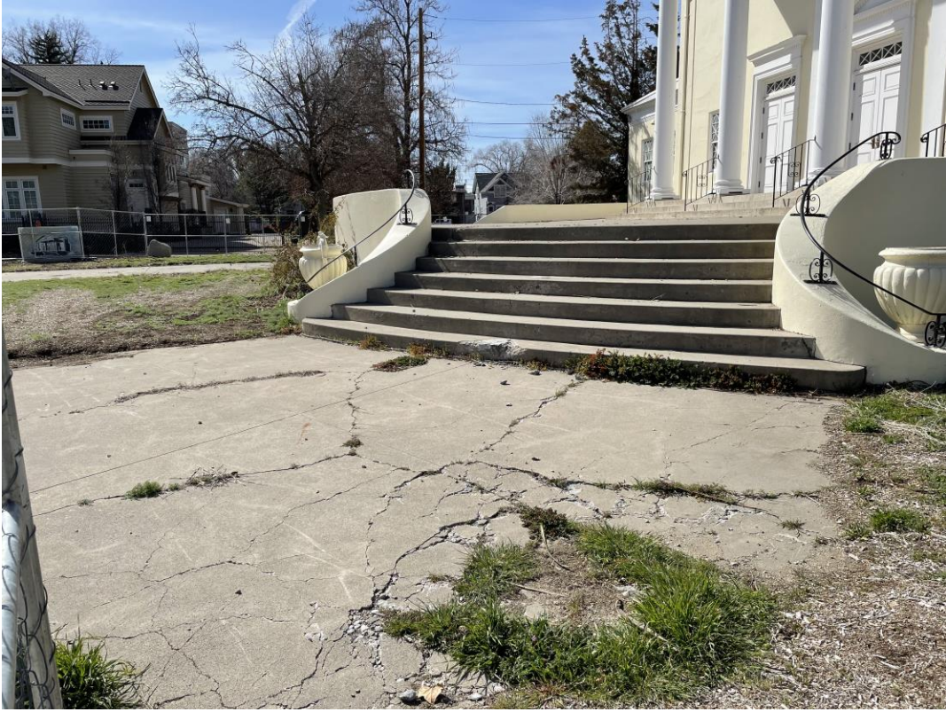
Detailed view of eastern staircase and sidewalk on south facade.
