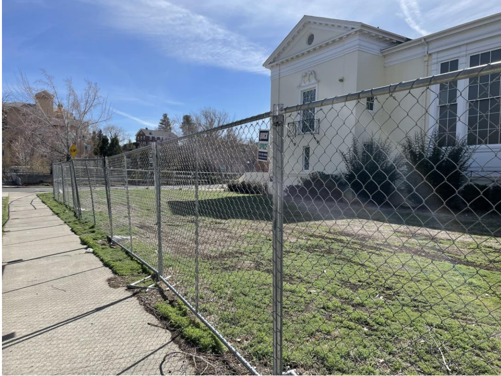
East facade, looking southwest.
