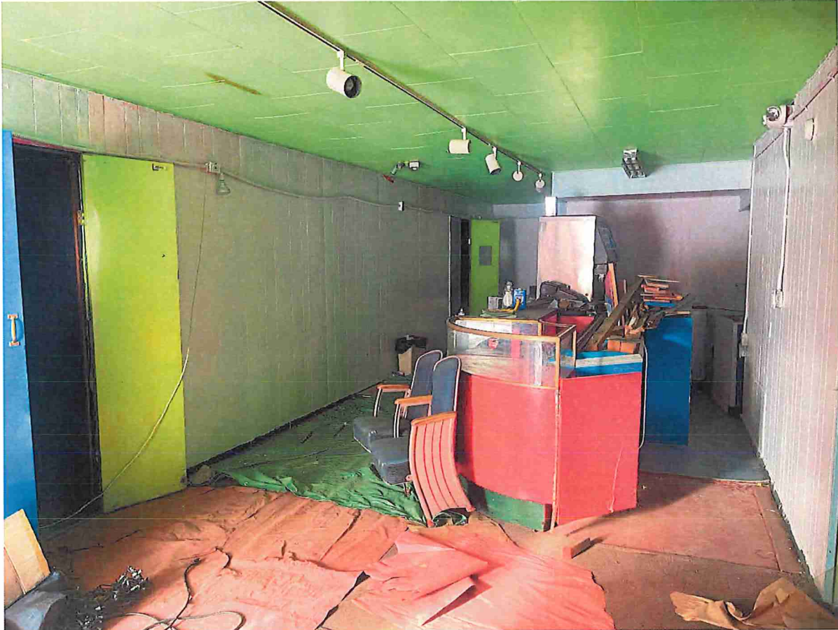
Lobby with rehabilitation in progress Kansas Bowling, 2023
