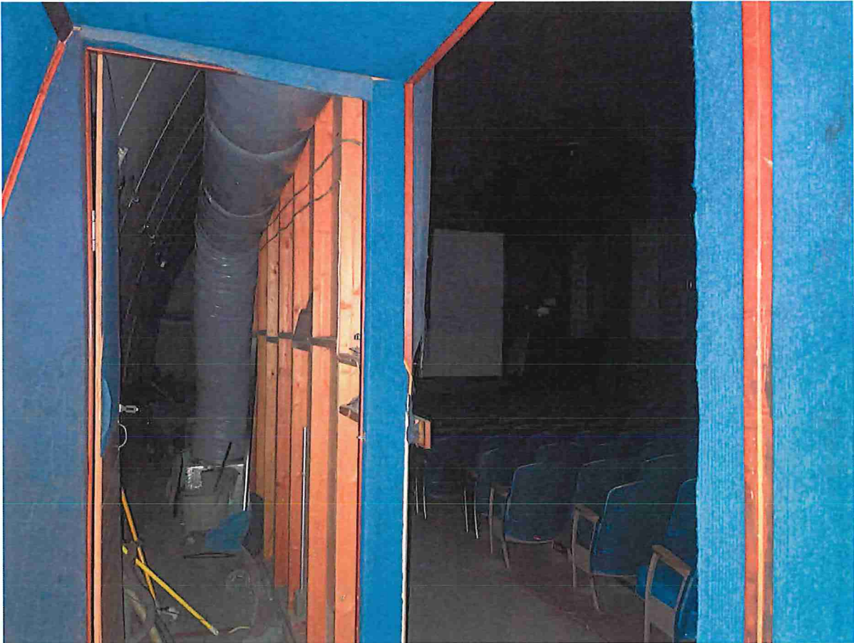
Theatre entrance and view of original curved exterior wall and 1960s interior wall Kansas Bowling, 2023
