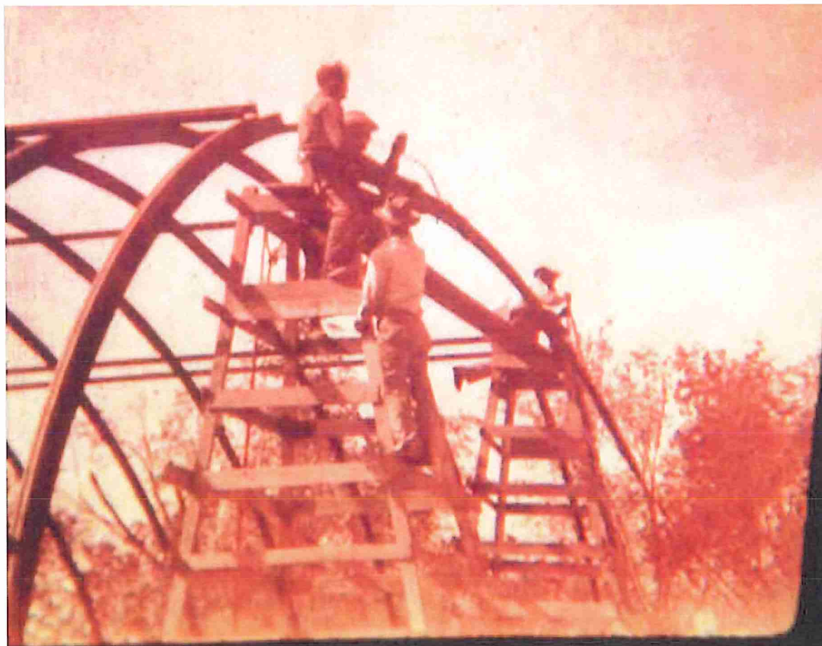
Theatre under construction in 1946 Photographer unknown, 1946 Image courtesy of Harold W. Fuller
