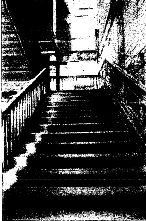
Image 44: Level 2 to Level 3 Stairwell view west up stairs
