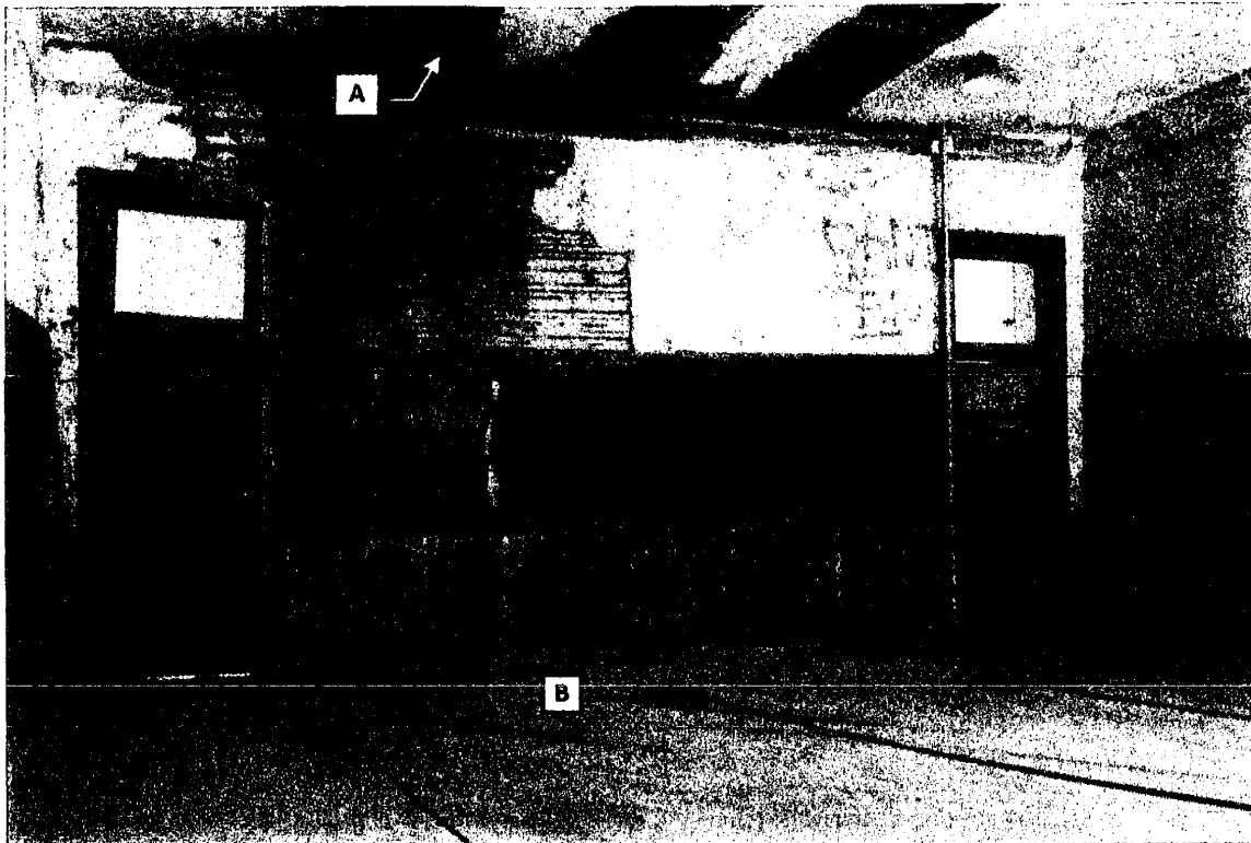
Image 54: Room 9 view north. (A) Lath and plaster are missing from ceiling, (B) Cable tie-downs
