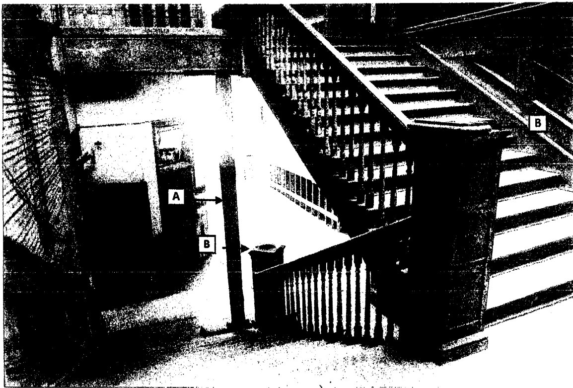
Image 45: Level 2 to Level 3 Stairwell view southeast. (A) Shoring pier per 2008 structural retrofit, (B) Missing finial.
