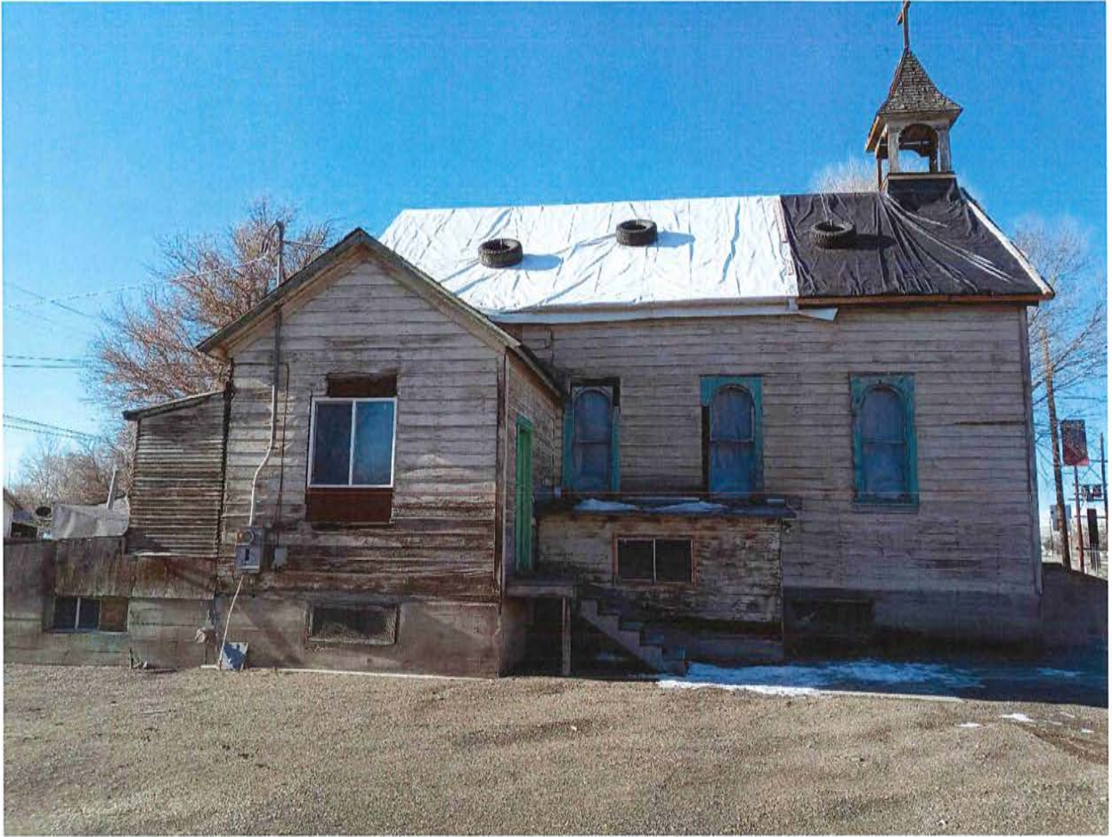
Side of Building Facing East
