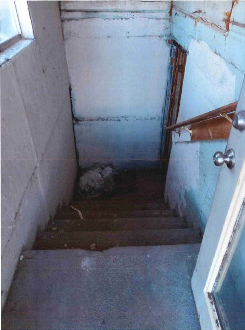
Stairs to Basement
