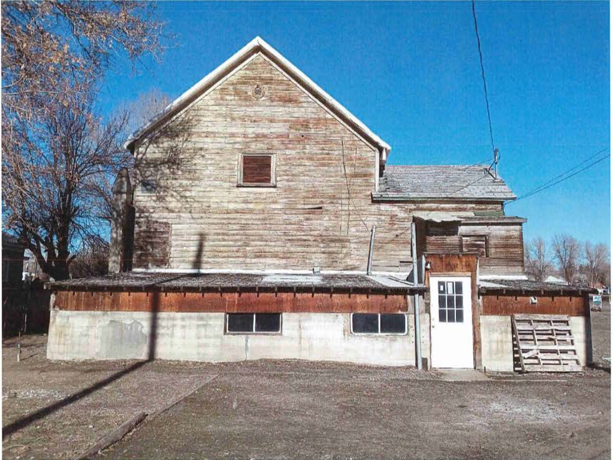
Rear of Building Facing South
