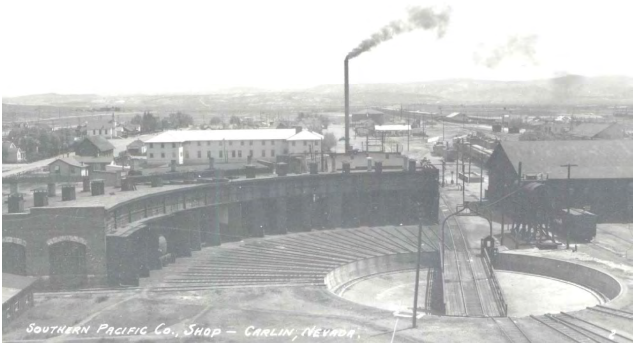
Southern Pacific Co., Shop — Carlin, Nevada. Carlin's 16-stall Roundhouse and Turntable. Circa 1940s, provided by Carlin Historical Society. Photographer Unknown.
