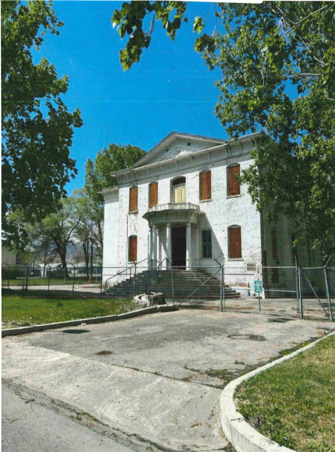
Southwest view from the street
