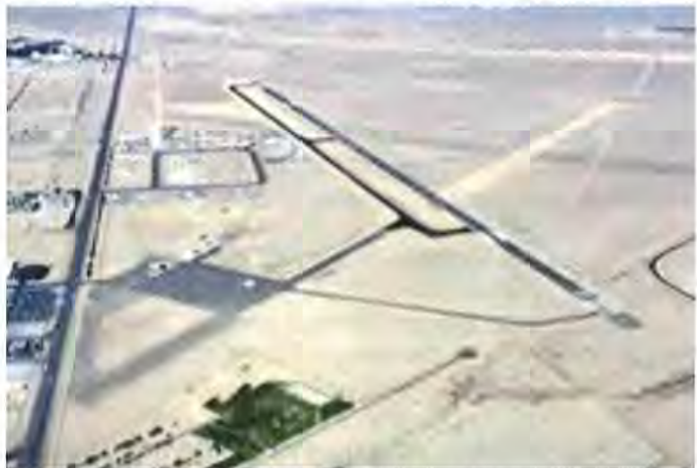
(Photo by Roger Kubeck) Hawthorne Airport
