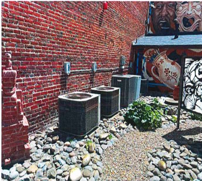
Brewery Annex Rooftop Condensers
