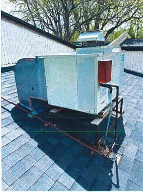
Brewery Office Pkg Unit west annex south view
