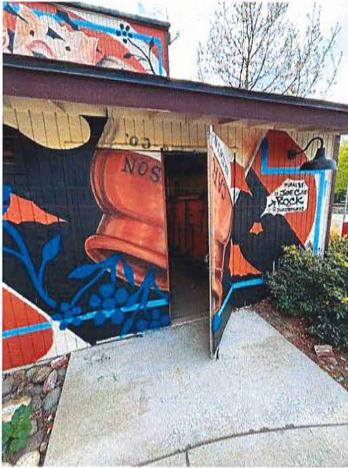
Brewery Annex Double Door Exterior south view
