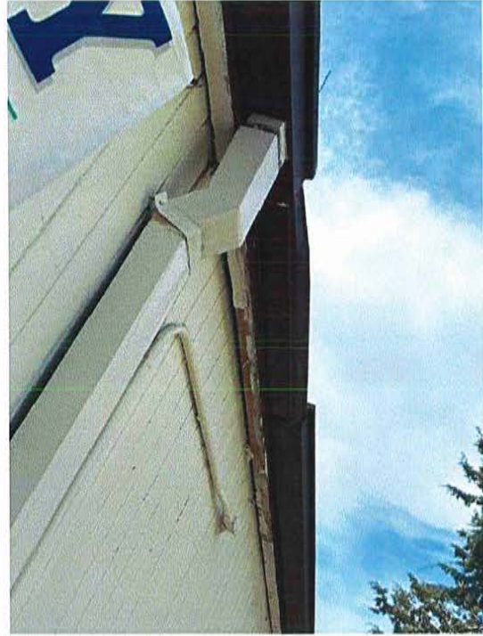
Gutter Downspout at NAA Gallery N. Side Annex
