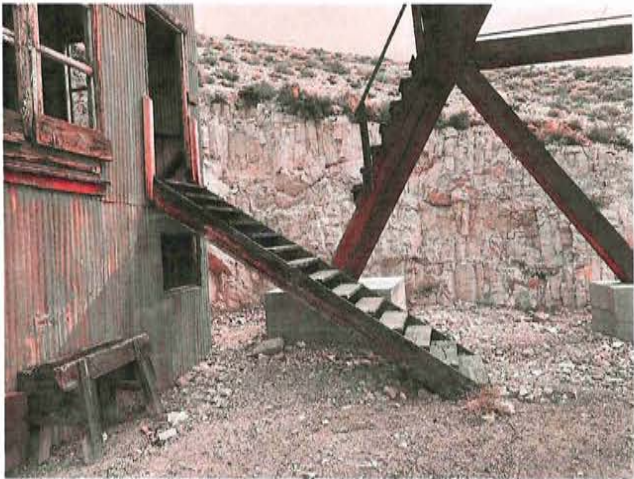
Hoist House facing east showing staircase
