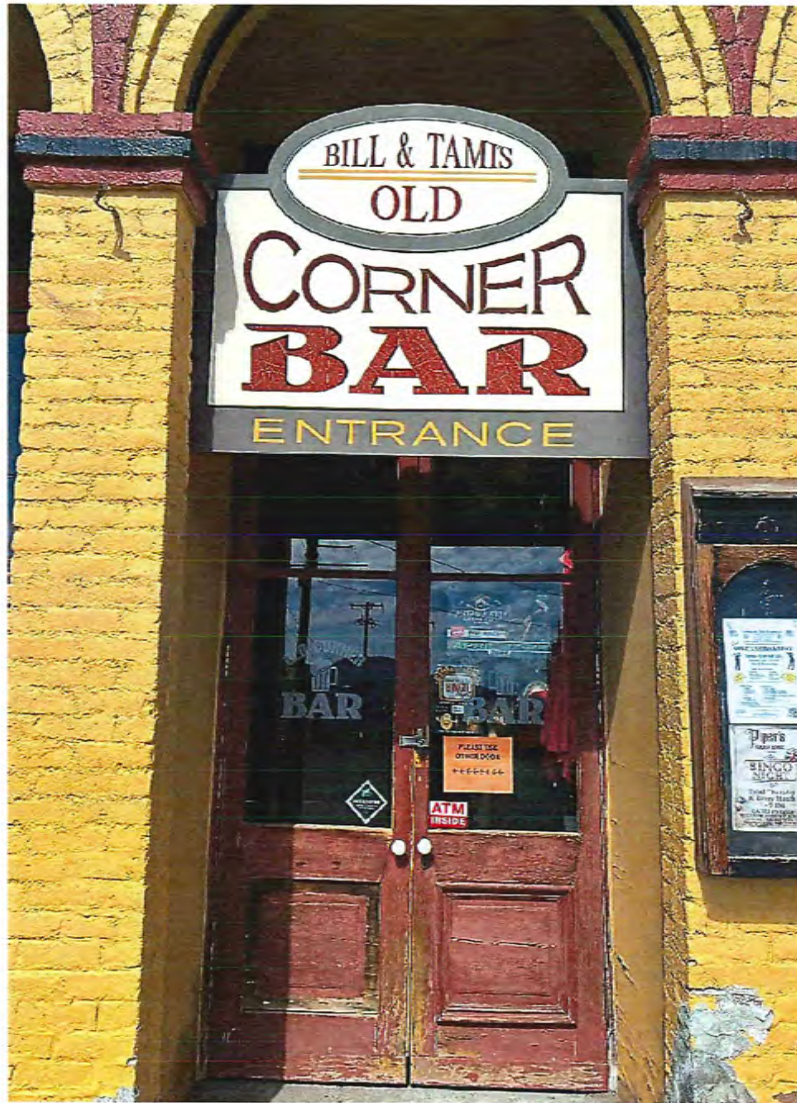
Photo 7: East elevation – 6 of 12 doors to be restored
