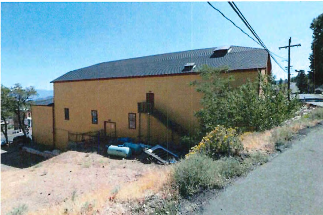
Photo 19 View looking south from A Street. Roof hatch visible lower left, smoke vent upper right
