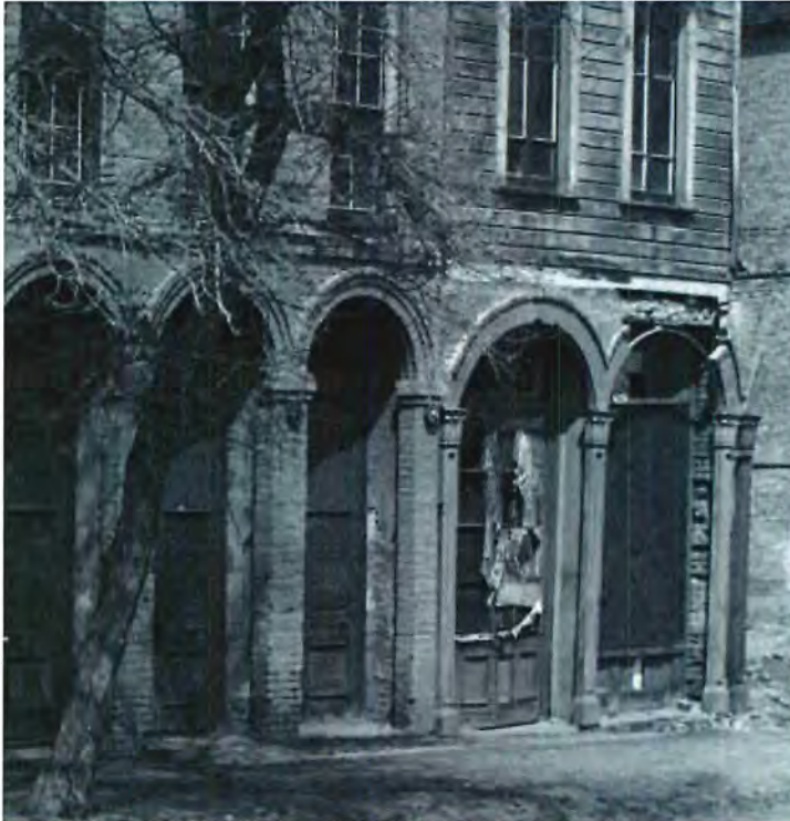
Photo 26 Four cast iron piers visible in photo to right. Pier at north end appears to support adjoining building which has been demolished
