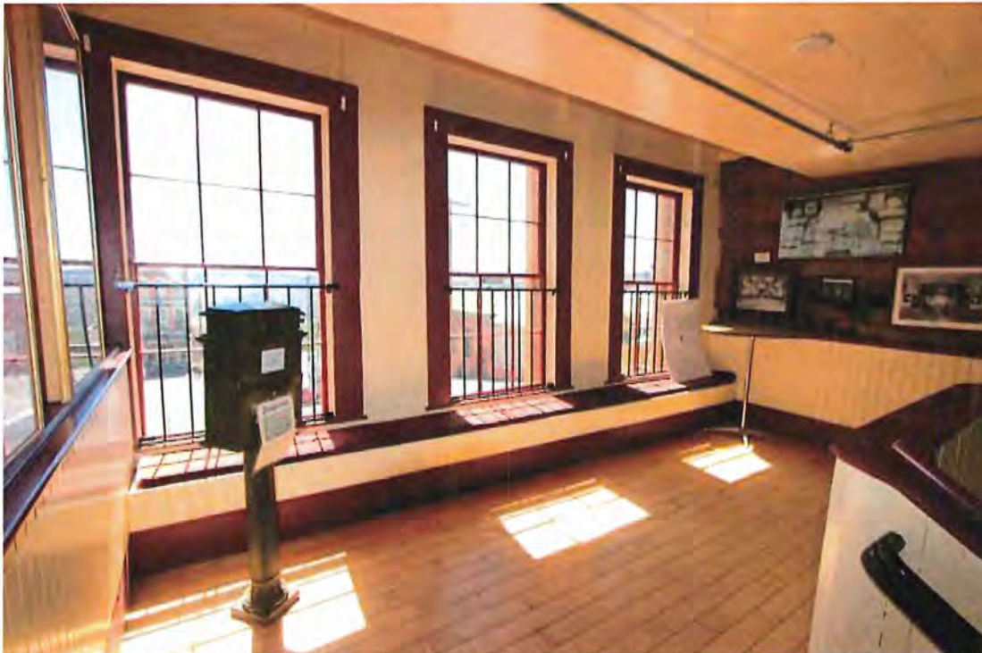
Photo 39 Looking east at auditorium lobby landing. Grills were added for fall protection. Salvaged lumber exposed above wainscot.
