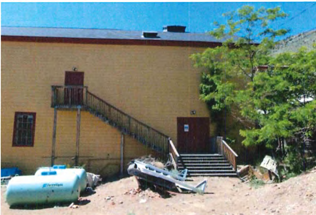
Photo 29 New exit at north balcony and stage left with staircase and landing constructed 1999
