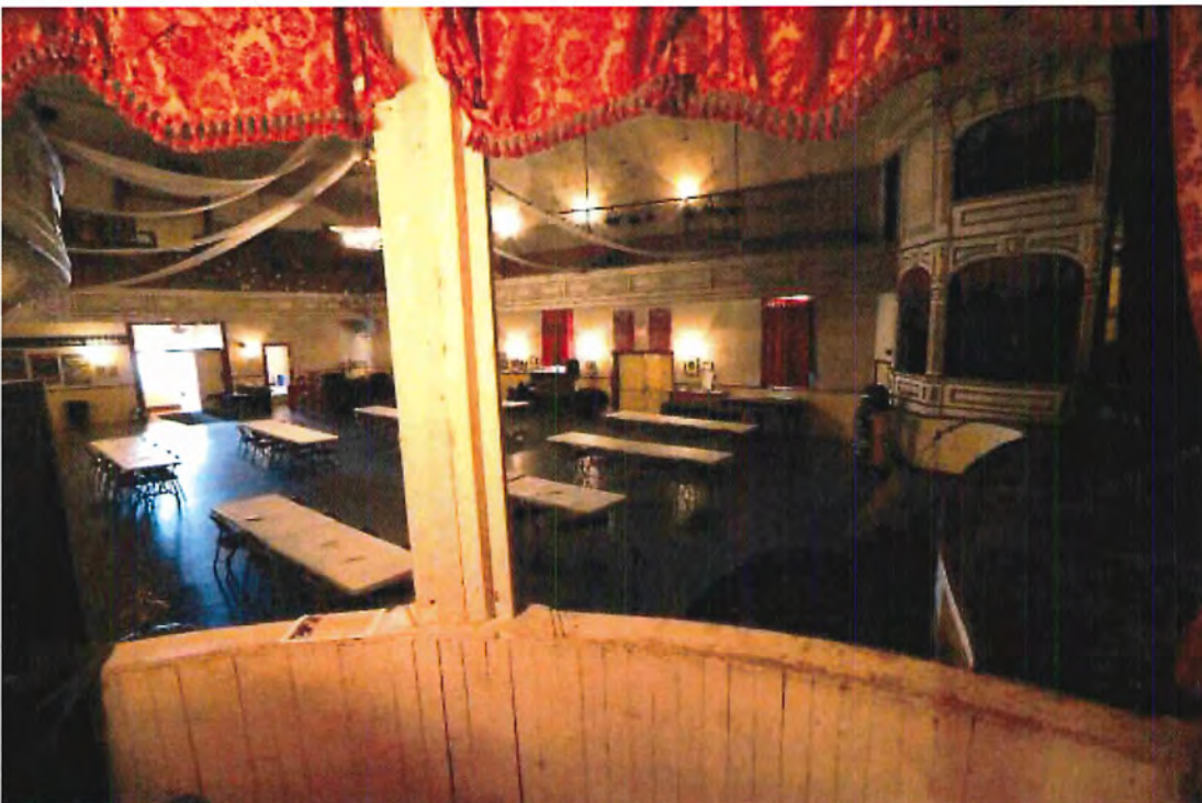
Photo 52 View of stage and auditorium chamber from lower opera box at stage left. Existing wood elements in fair condition.
