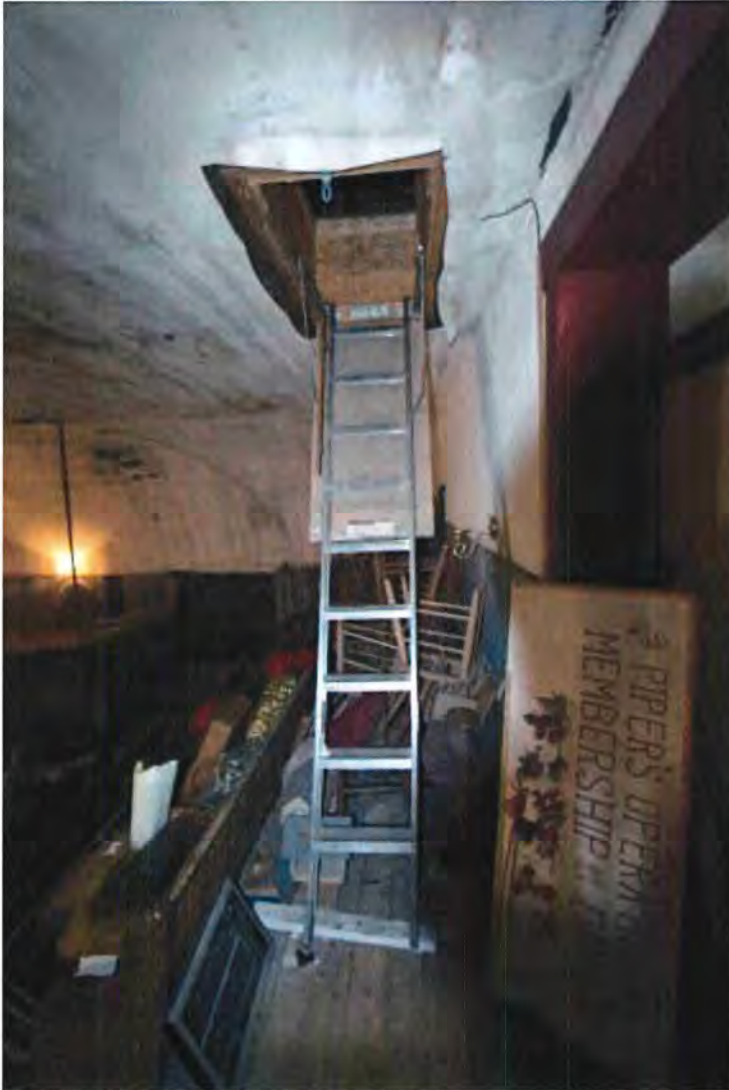
Photo 66 Attic access via pull down ladder
