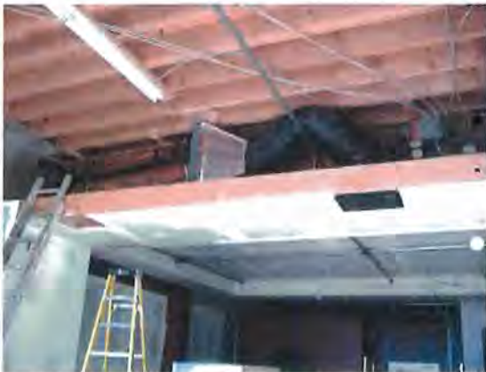
Photo 7 Heater above Old Corner Bar ceiling
