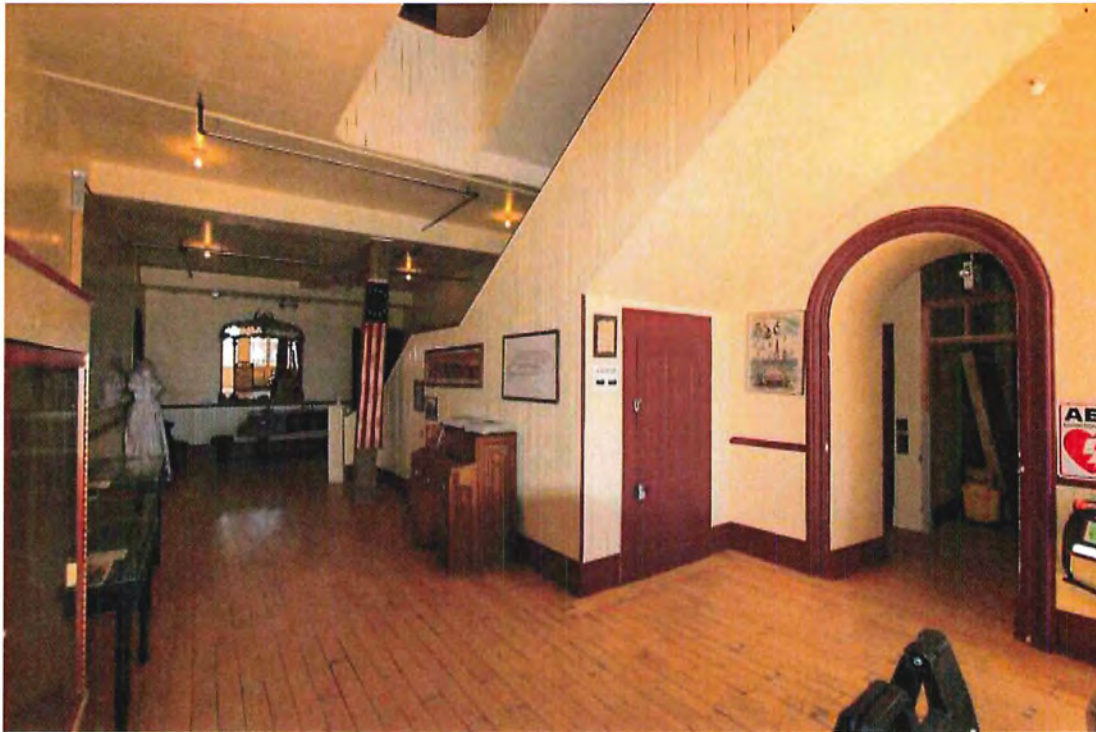
Photo 33 B Street lobby looking west. Walls are plastered and painted with bead board wainscoting and cap. Wood ceiling with soffits to hide piping. Wood column in middle of photo leaning. Stairs complete. New maple flooring over hydronic heating tubes. New director's office visible through archway.
