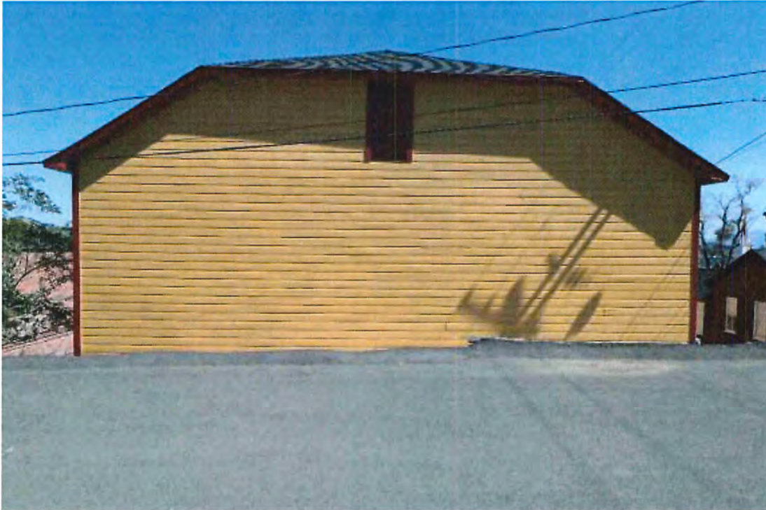
Photo 25 West elevation from A Street looking east. Door above stage provides additional attic access. Siding was replaced over new plywood sheathing.
