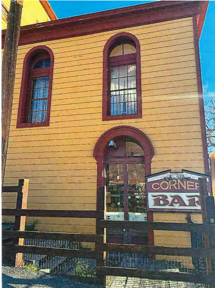
Photo 17: Overview of two south wall windows over Corner Bar
