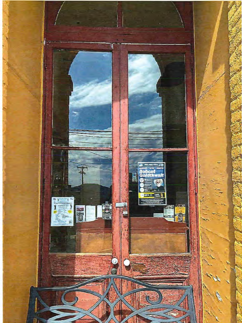
Photo 8: East elevation – 8 of 12 doors to be restored
