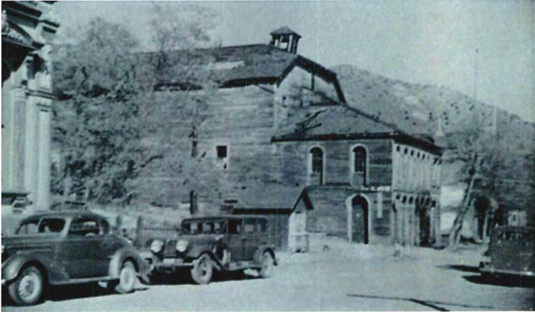
Photo 18 Hip roof ventilator, circa 1939
