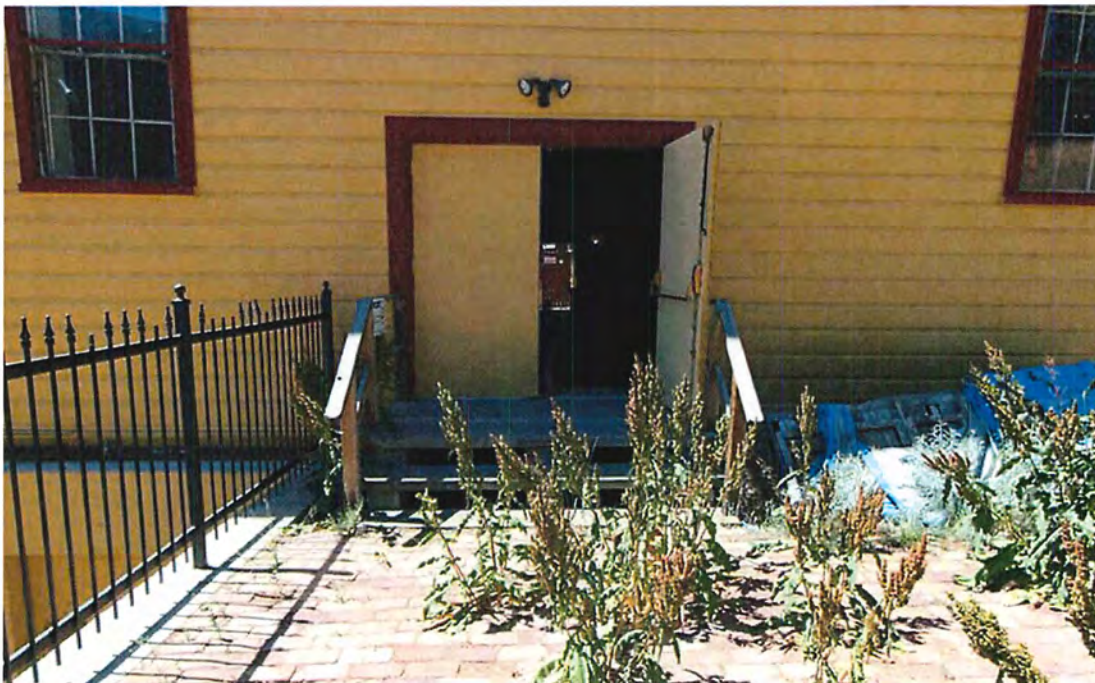
Photo 54 North exit from auditorium
