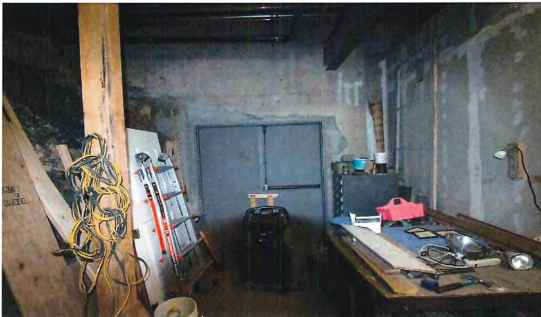
Photo 38 View of double egress doors looking north. Note blocked exit. New partition wall will align with the footing supporting the column.
