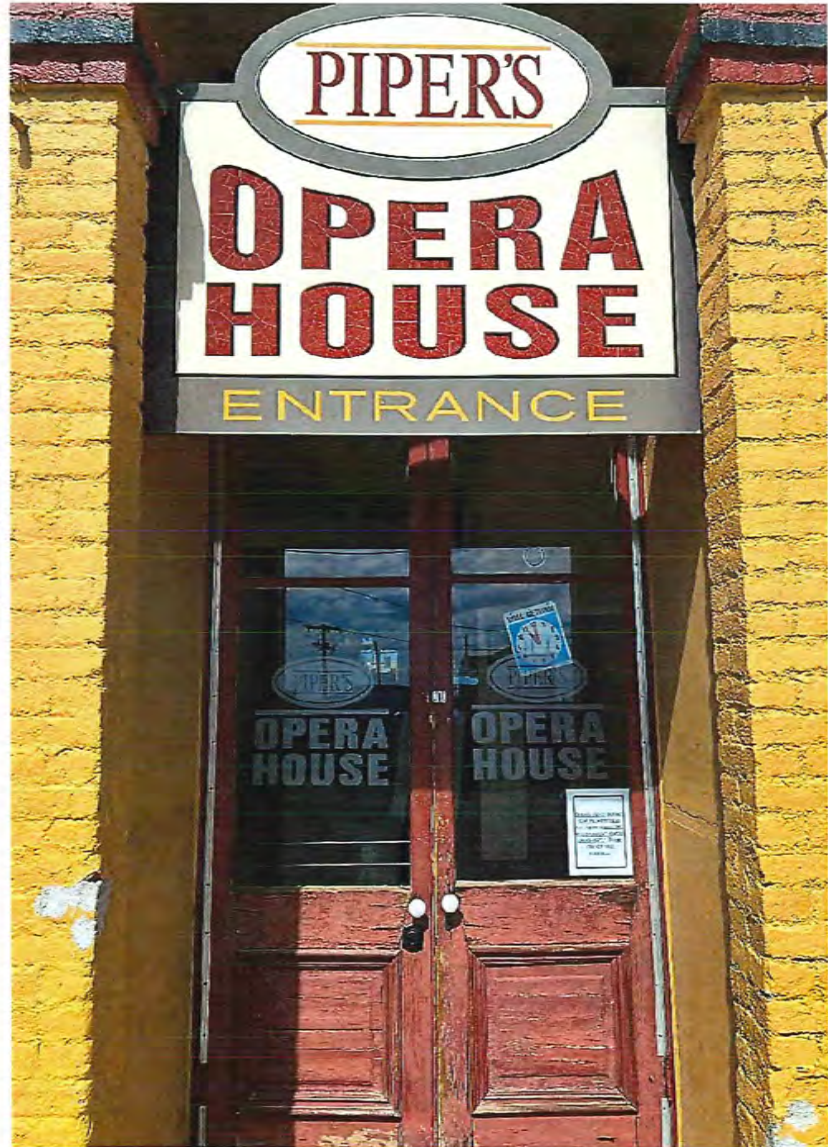
Photo 10: East elevation – 10 of 12 doors to be restored
