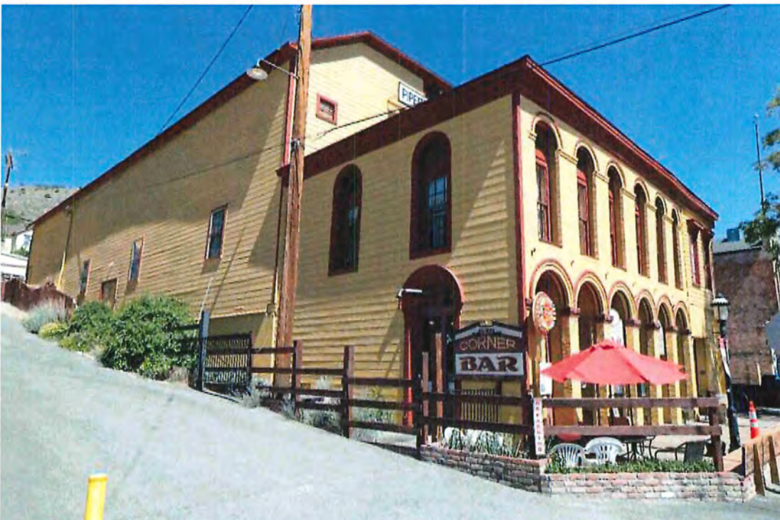
Photo 21 View looking northwest from B Street. Shiplap siding covering brick on south elevation of 1863 building. Flue coming out of arched window vents pellet stove used to heat Old Corner Bar. Seven doors with archways and eight second level windows (facing south and east) were refurbished in 2003. Note high window facing east in upper balcony.
