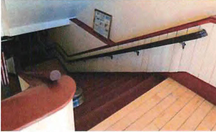
Photo 59 Existing stairs complete with handrails on both sides of stairs; half-round bannister cap, bead board wainscoting, and vinyl treads and risers
