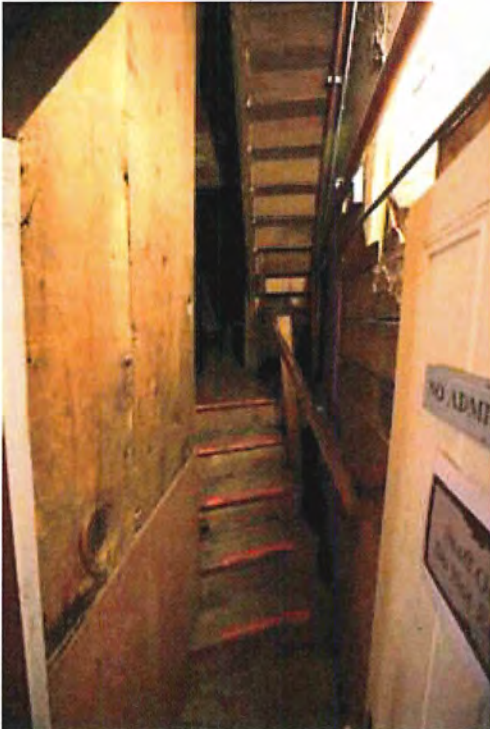
Photo 51 Stairs to opera boxes at stage left
