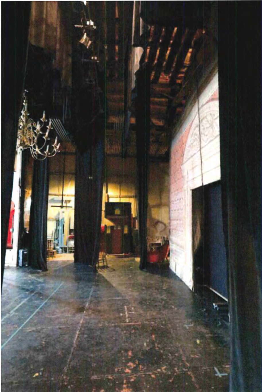
Photo 58 View from stage left looking south. Note light through floor boards of loft area in attic above stage.
