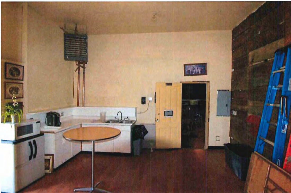
Photo 43 View of existing kitchenette looking west. Auditorium visible through open doorway. Exposed wall sheathed in salvaged lumber shown on right side of photo should be protected in place and left exposed for interpretation or covered with fabric and new wall paper attached. Electrical subpanel to right of doorway. Fan coil unit for heating in kitchenette and adjoining Bridal Room. New flooring overlaid on existing wood floors
