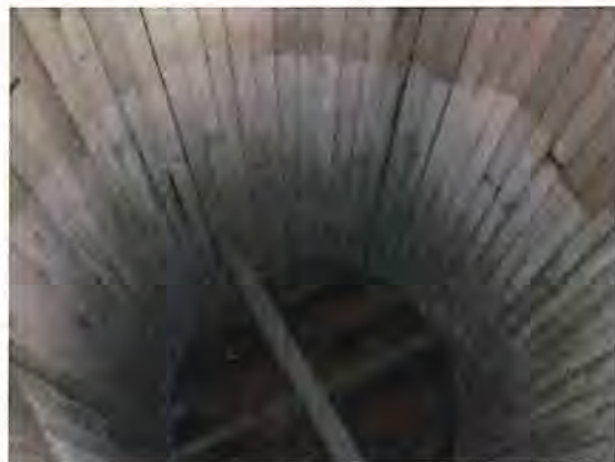
Photo 5 Existing Ventilation Shaft from Auditorium
