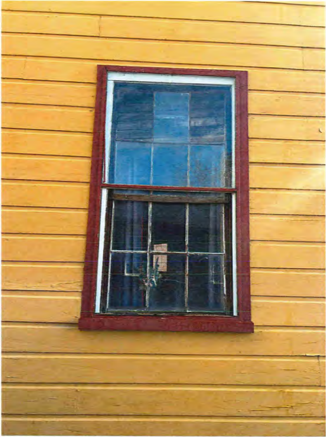
Photo 14: Window 1 of 5 (windows are presented here from the west to east)
