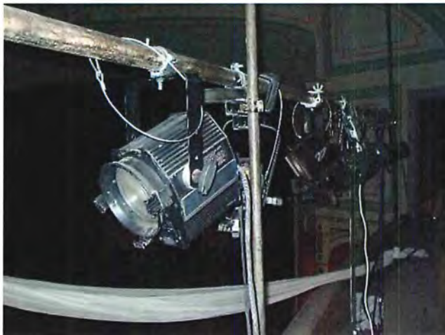
Photo 16 Balcony stage lights and pipe rigging
