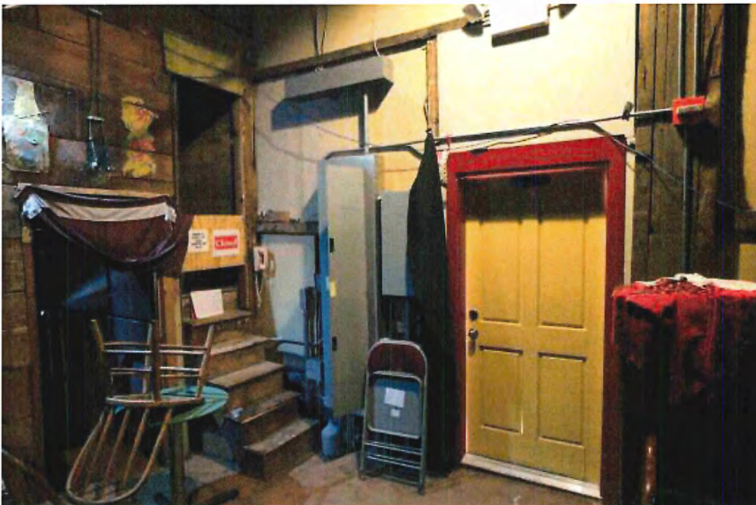
Photo 57 view from stage right. Stairs on right go up to balcony, stairs to left go down to auditorium. Stage exit door facing south. Note electrical panels to left of door.
