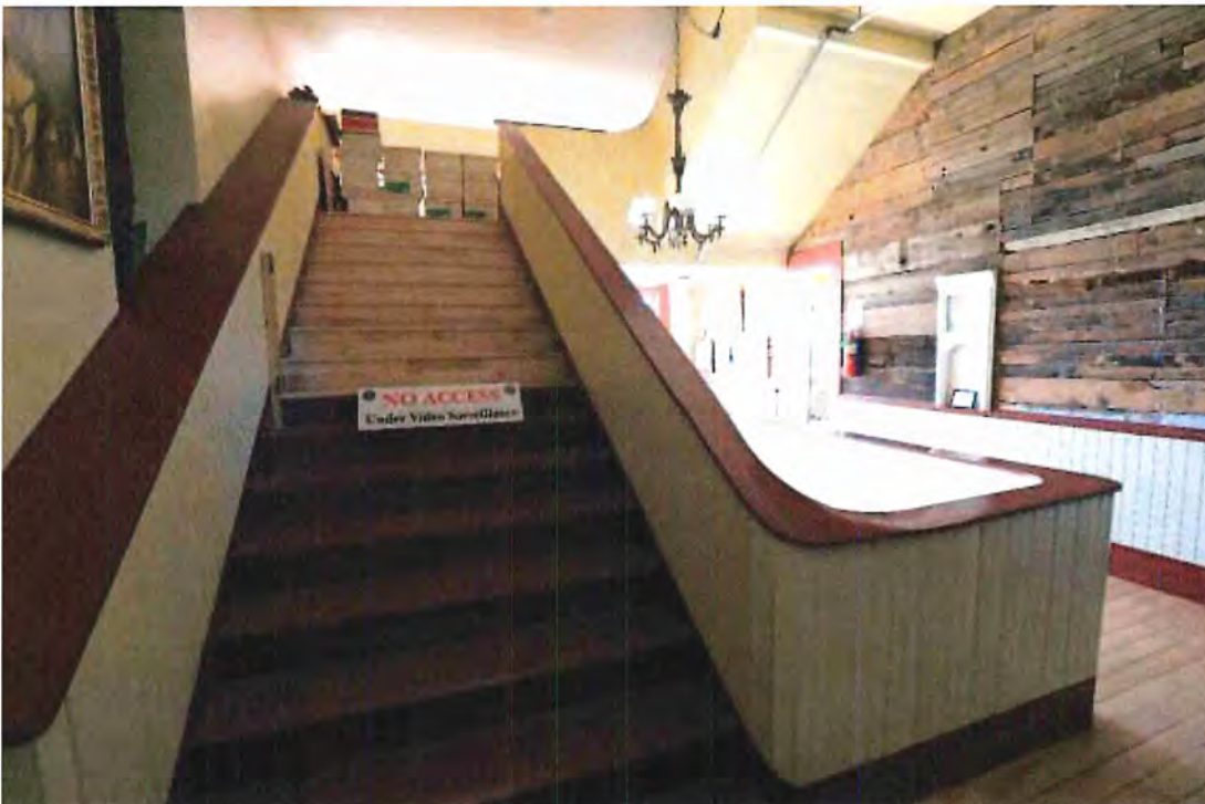
Photo 60 View looking east of partially completed stairs to balcony level.
