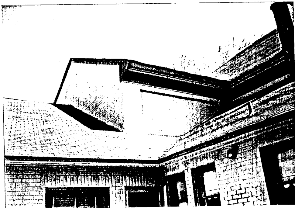
Photo 8. Photograph of the roof where several additional join. Areas such as this require special structural ties to distribute loads around it.
