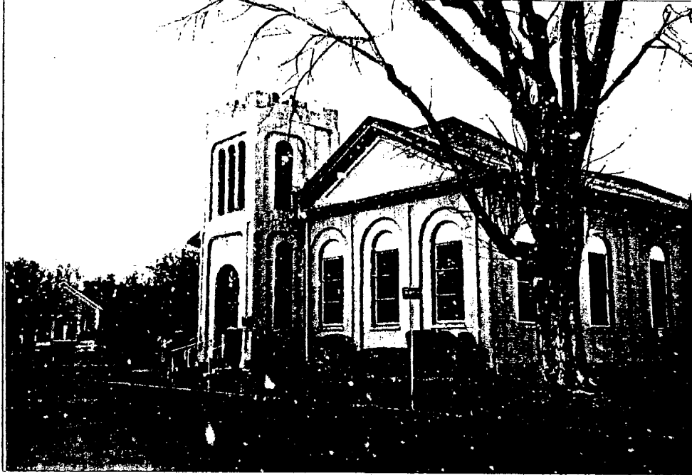
Photo 1. Front, east, elevation showing original church and tower.
