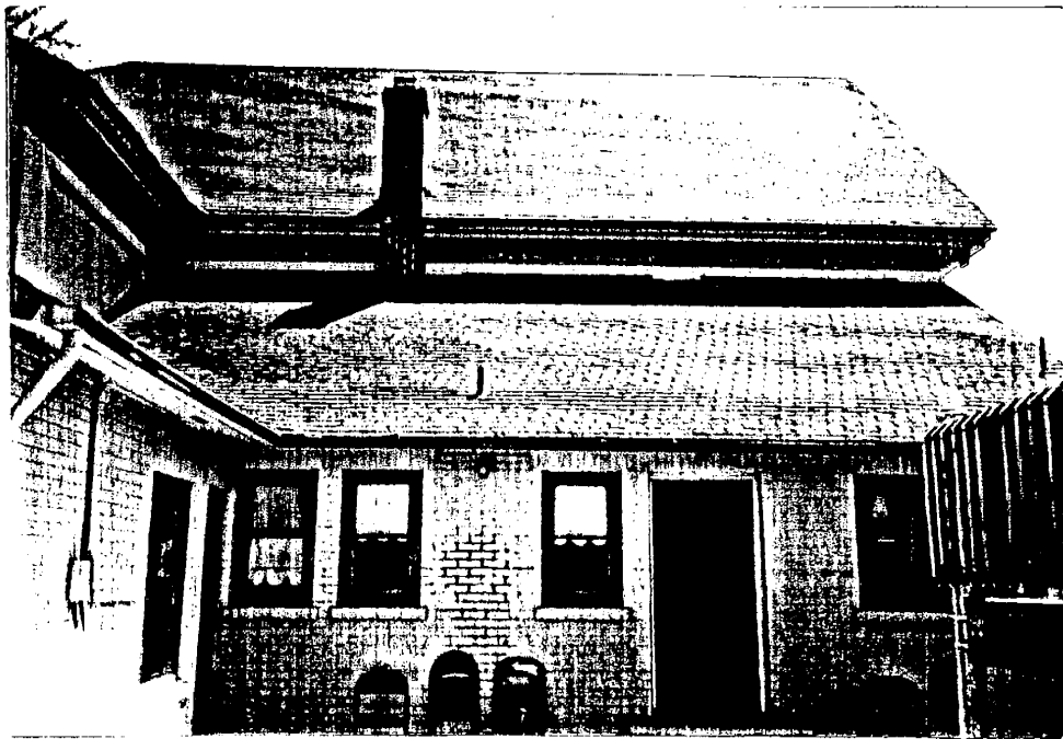
Photo 6. West elevations showing additions. The walls of these additions will require further investigation.
