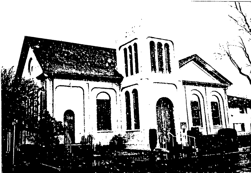
Photo 2. East and south elevations, front of church. The gable ends at the south and east are visible. These are some of the tall walls that will require bracing.
