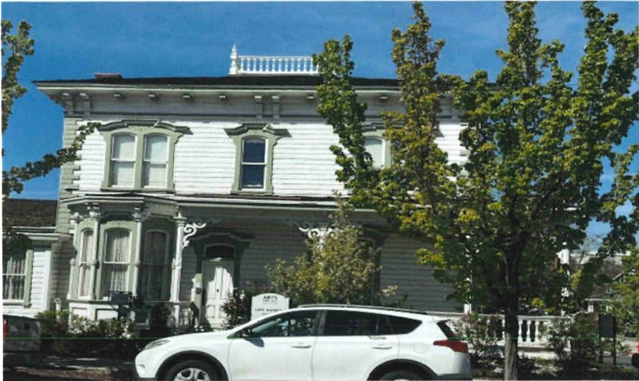
2) Eastern Elevation of the Lake Mansion
