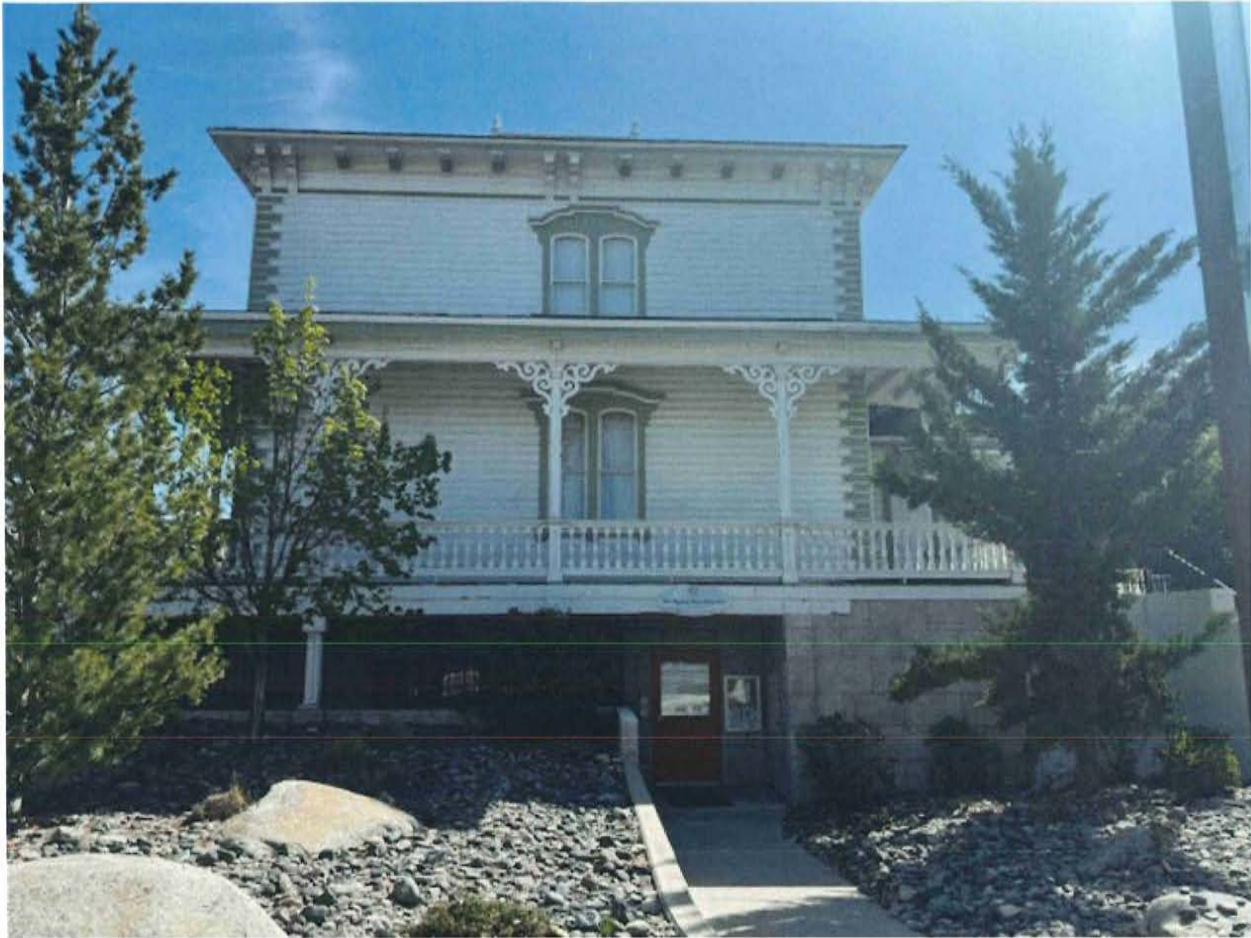
4) Western Elevation of the Lake Mansion
