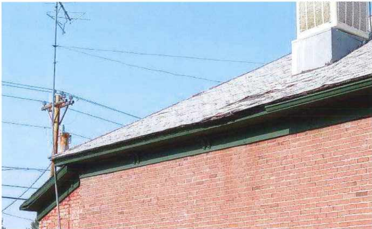
West Side of Building Looking North (Missing Gutter)
