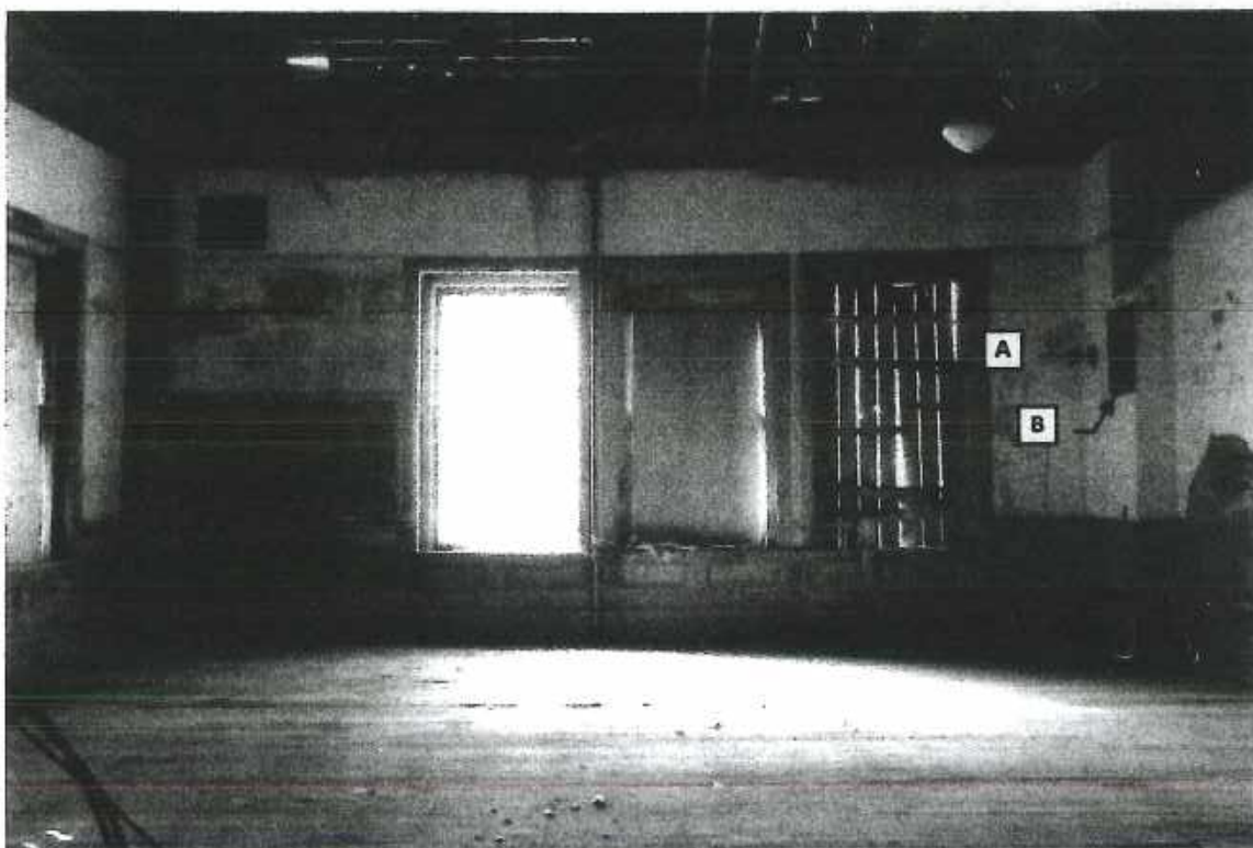
Image 94: Room 17 view west. (A) Flue opening in wall for non-extant wood burning stove, (B) Heating Vent.
