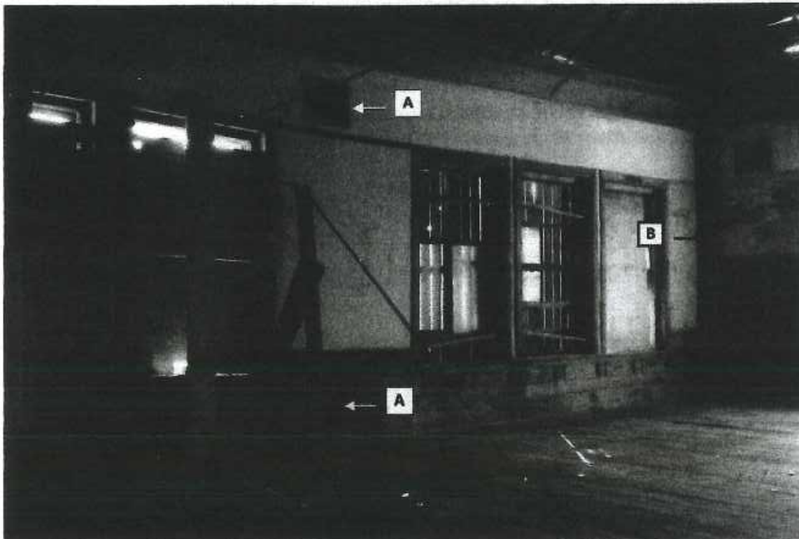
Image 93: Room 17 view southwest. (A) Upper and Lower Fresh Air Gravity Vents. (B) Wainscot-sided pipe chase.
