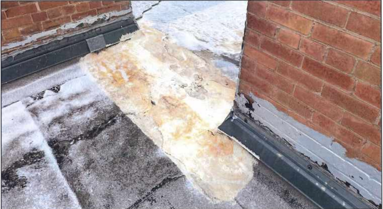
Photo 11 – This view shows one of the temporary patches that we have made to stop a leak.
