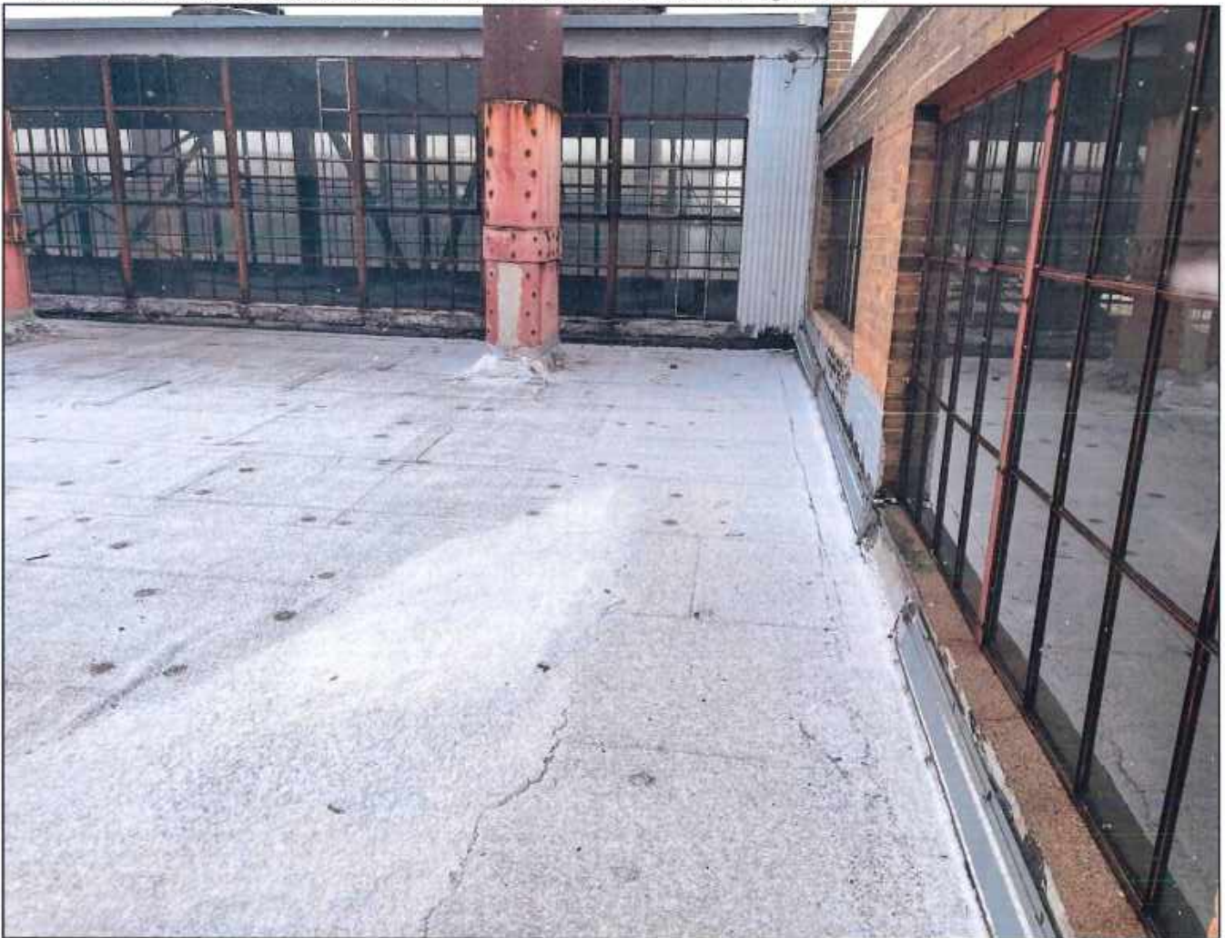
Photo 4 – This is the engine house roof showing the skylight windows and one of the smoke jacks.
