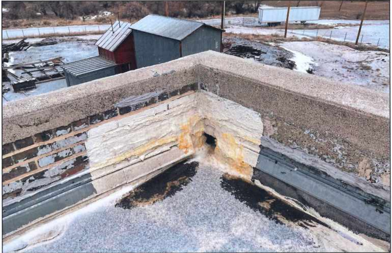
Photo 7 – This is the engine house roof showing one of the roof drains. We have made temporary repairs here. A previous CCA grant paid for repairs to this wall. The repairs were needed because the water had infiltrated the brick wall and caused damage because of the freeze thaw cycle.
