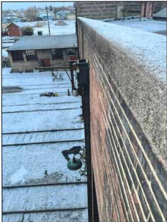
Photo 8 - This is the east wall of the engine house showing one of the roof drains. The drains are made out of copper sheets. They drain into a storm sewer that has failed on the east side of the engine house. The storm sewer goes under the six engine house tracks and it has collapsed.
