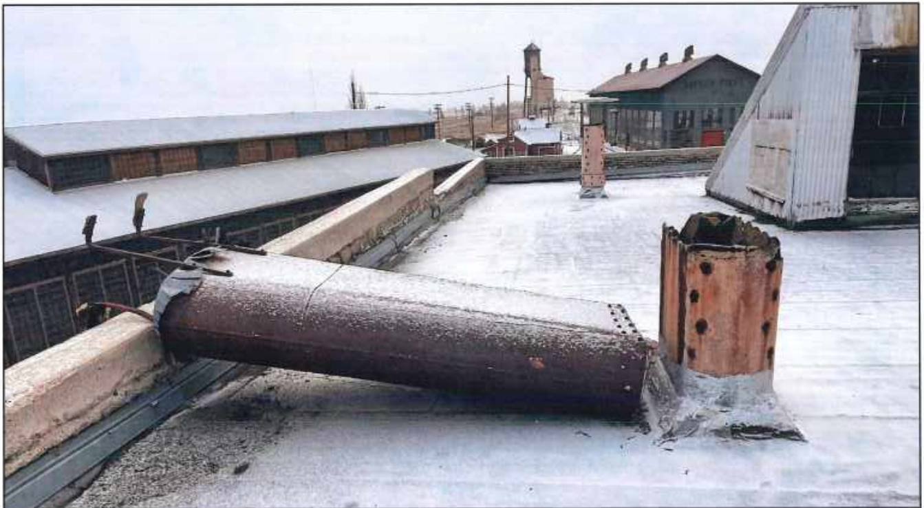
Photo 10 – This view shows that one of the smoke jacks has completely failed and needs to be repaired.
