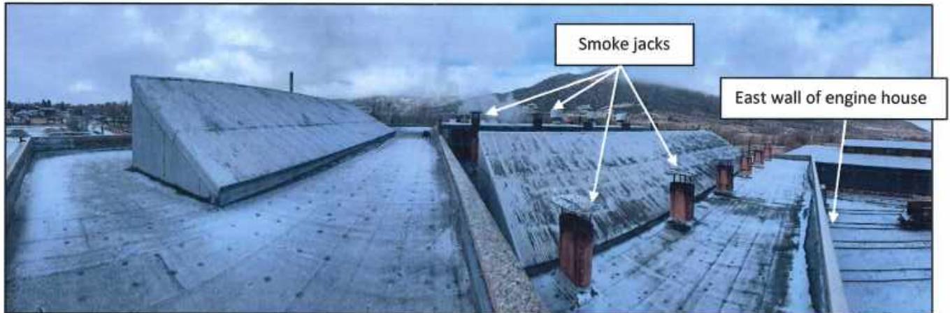
Photo 3 – This is a panoramic view of the roof structure looking west and north. Going from left to right is the machine shop roof. The structure in the foreground is one of the window structures. Going through the center of the photo is one of the parapet walls separating one of the levels. Going further to the right is engine house roof. Twelve of the smoke jacks are visible and one has smoke coming out of it.
