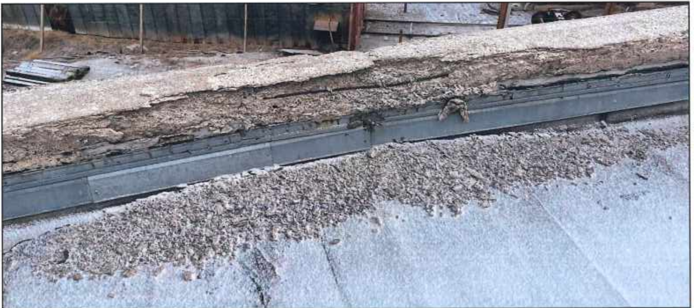
Photo 6 – This is one of the crumbling parapet walls.
