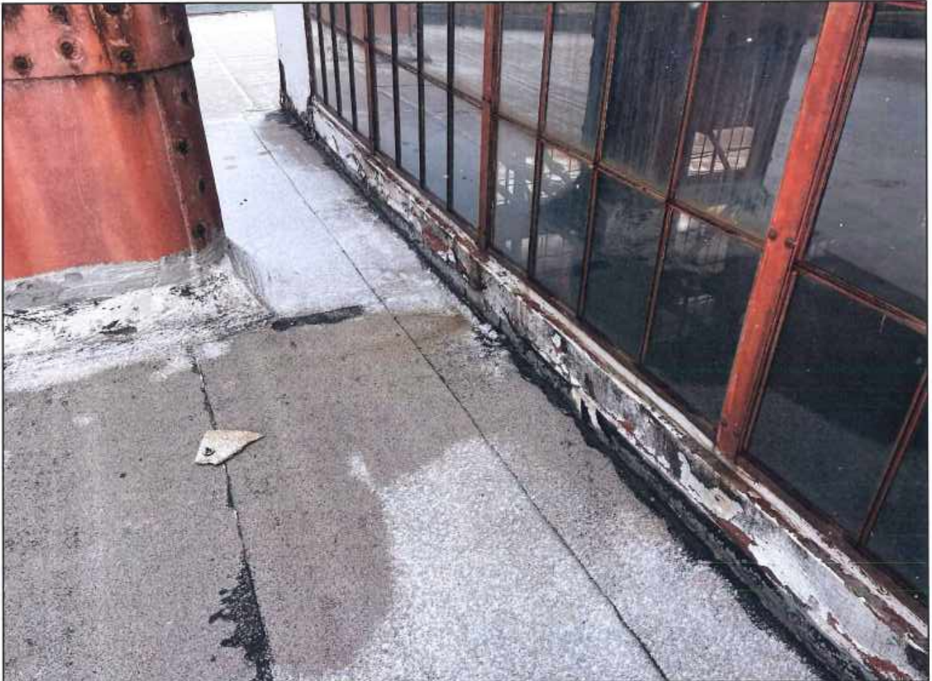
Photo 5 – Another view of the engine house roof showing the skylight windows and one of the smoke jacks.
