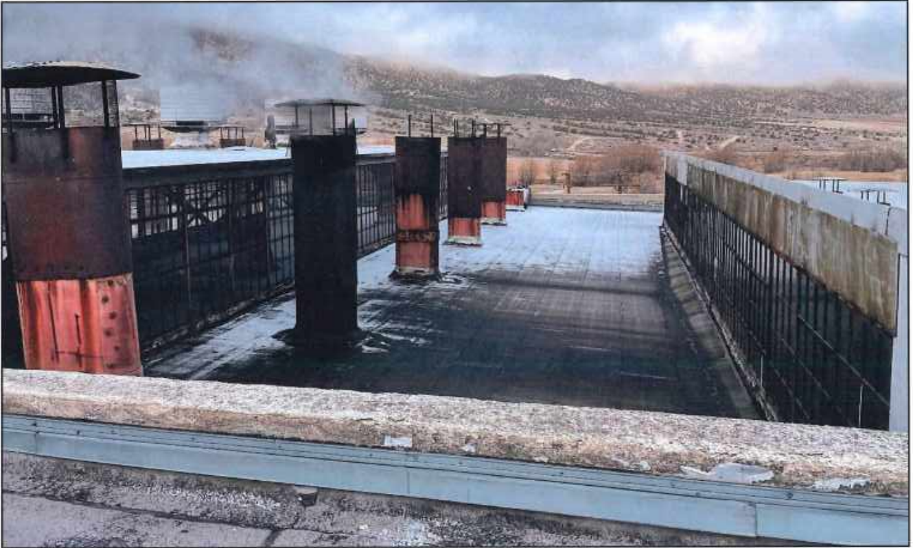
Photo 9 – This view is looking north from the machine shop roof to the engine house roof, two of the smoke jacks are missing the covers.
