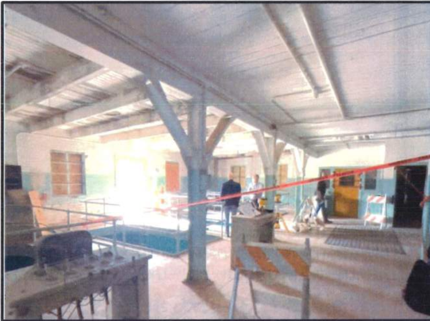
Figure 20 – Underside of Second Floor Framing and Steel Frame Supporting South End of Second Floor
