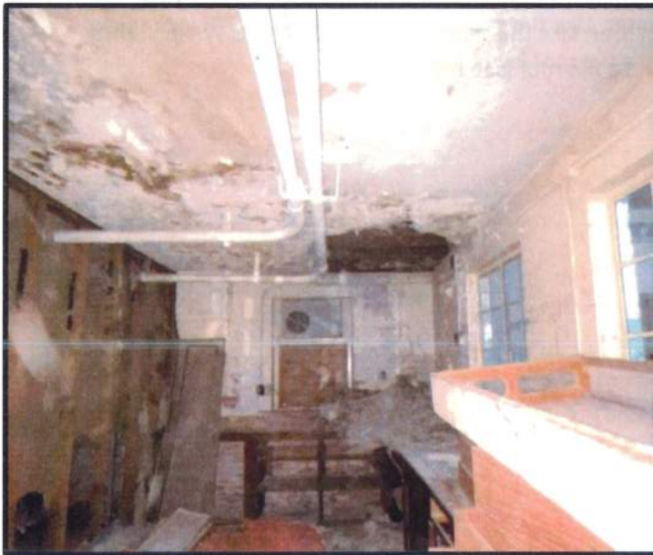
Figure 27 – Plaster Ceiling Failure at NW Addition
