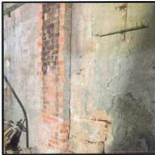
Figure 32 – One Wythe of Old Chimney Still Remains
