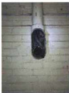
Photo 1 - Interior Service Entrance Conduit and Cut Conductors
