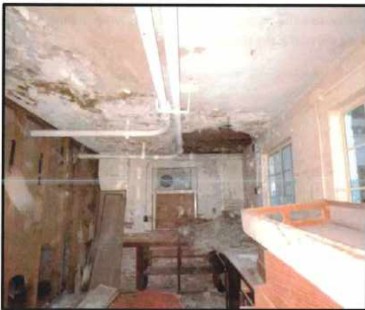
Figure 27 – Plaster Ceiling Failure at NW Addition
