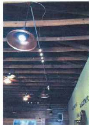
[40] Not Recommended: Removing a finished ceiling and leaving the structure exposed in a historic retail space does not meet the Standards for Rehabilitation.
