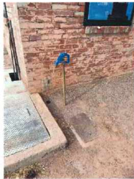
Photo 4 - Existing Water Meter & Yard Hydrant
