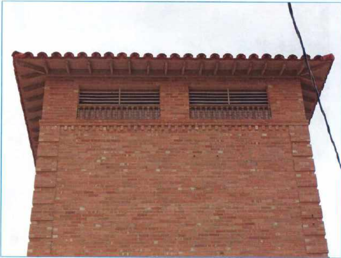
Photograph 8. Copper louvered vents with turned wood balustrades on all four sides of the tower, and brick quoins, are significant features of the Plant.
