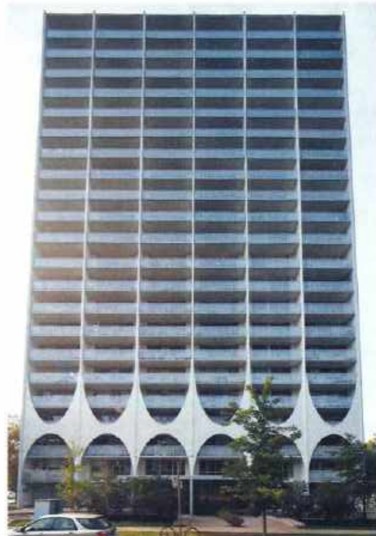
[59] (a-b) The decorative concrete balcony railings on this 1960s building did not meet life-safety code requirements. They were replaced with new glass railings with a fritted glass pattern matching the original design—a creative solution that satisfies codes, while preserving the historic appearance of the building when viewed from the street (c-d). Photos: (a, b, d) ERA Architects, Inc.; (c) Nathan Cypris, photographer.
