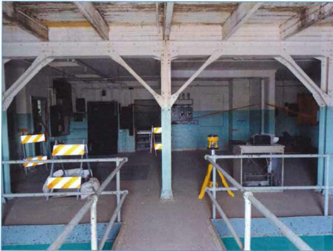
Photograph 11. Interior of Operating Floor showing structural steel beams and columns with rivets, facing northeast. The columns and beams are considered character-defining features.
