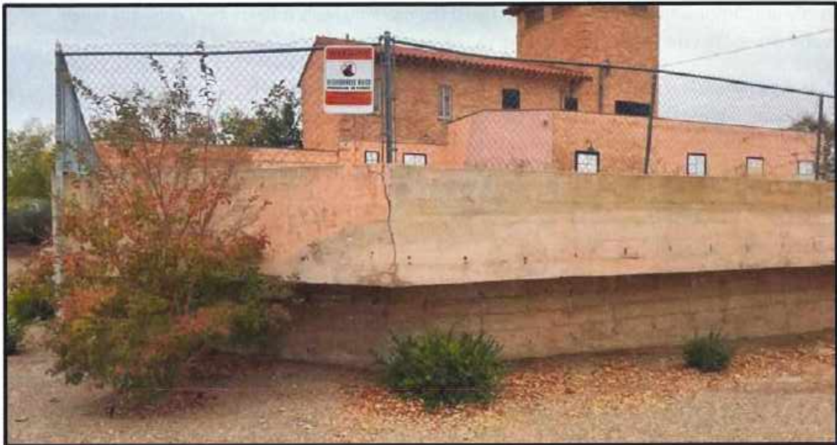
Figure 31 – Crack at Clarifier Tank Retaining Wall
