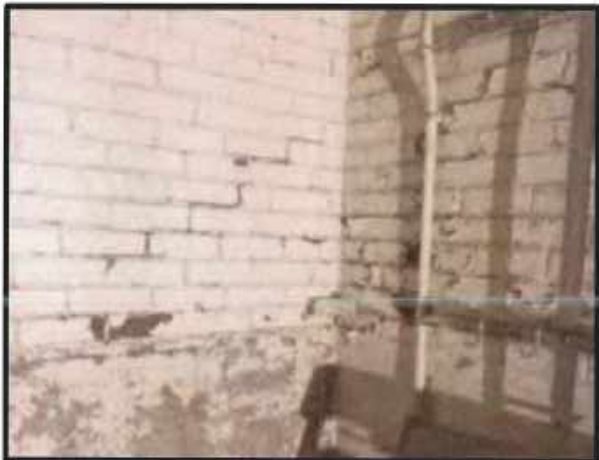
Figure 13 – Step Cracking at South Corner of Unloading Shed
