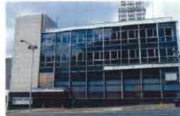
[31 a-c] (a) The rehabilitation of the First Federal Savings and Loan Association building in Birmingham, AL, constructed in 1961, required replacing the deteriorated historic curtain wall system because the framing and the fasteners holding the spandrel glass and the windows had failed. (b) Comparative drawings show that the differences between the replacement system, which incorporated new insulated glass to meet wind-load requirements, and the original system are minimal. (c) The replacement system, shown after completion of the project, has not altered the historic character of the building.
