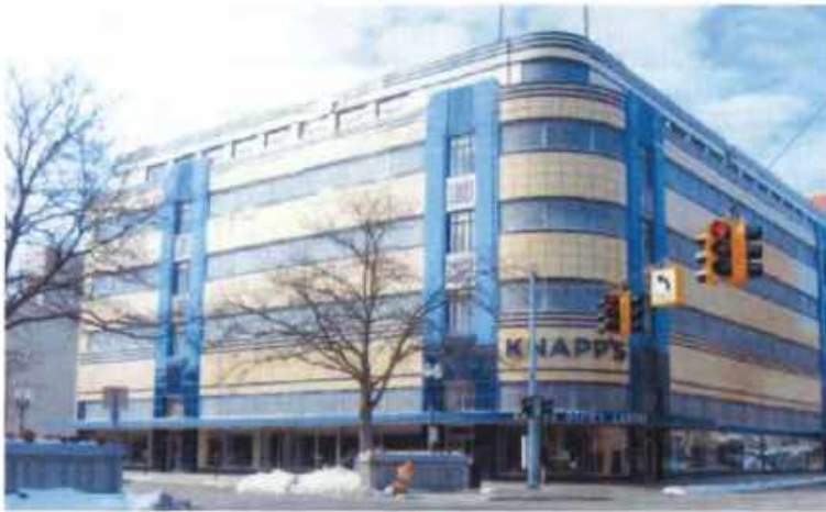
[7] (a) J.W. Knapp's Department Store, built 1937-38, in Lansing, MI, was constructed with a proprietary material named "Maul Macotta" made of enameled steel and cast-in-place concrete panels. Prior to its rehabilitation, a building inspection revealed that, due to a flaw in the original design and construction, the material was deteriorated beyond repair. The architects for the rehabilitation project devised a replacement system (b) consisting of enameled aluminum panels that matched the original colors (c). Photos and drawing (a-b): Quinn Evans Architects; Photo (c): James Haeffner Photography.
