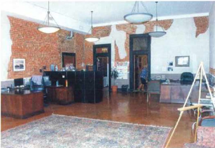
[41] Not Recommended: Leaving fragments of deteriorated or "scabbed" plaster is not a compatible treatment for either finished or unfinished interior spaces.
