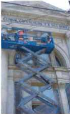
[1] An alkaline-based product is appropriate for use to clean historic marble because it will not damage the marble, which is acid sensitive.
