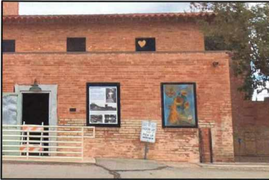
Figure 29 – Mortar Loss Due to Rising Damp
