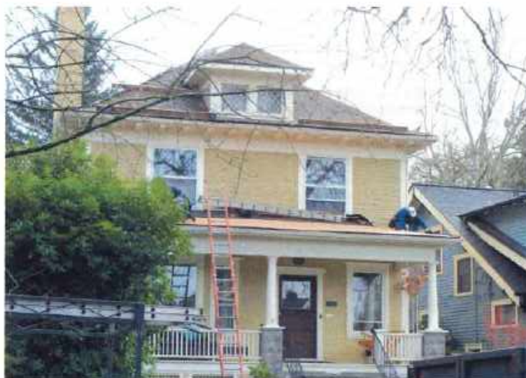
[6] The deteriorated asphalt shingles of this porch roof are being replaced in kind with matching shingles.
