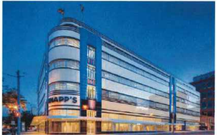
[7] (a) J.W. Knapp's Department Store, built 1937-38, in Lansing, MI, was constructed with a proprietary material named "Maul Macotta" made of enameled steel and cast-in-place concrete panels. Prior to its rehabilitation, a building inspection revealed that, due to a flaw in the original design and construction, the material was deteriorated beyond repair. The architects for the rehabilitation project devised a replacement system (b) consisting of enameled aluminum panels that matched the original colors (c). Photos and drawing (a-b): Quinn Evans Architects; Photo (c): James Haeffner Photography.
