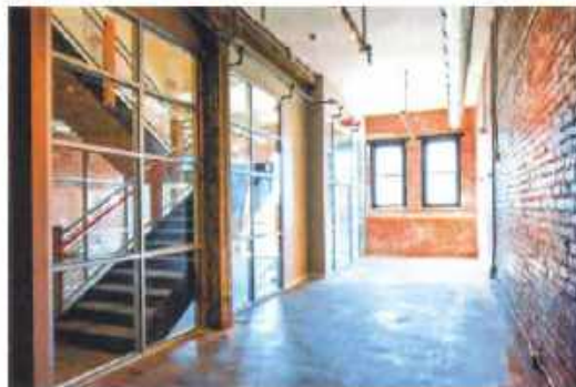
[38] The rehabilitation project retained the industrial character of this historic factory building, which included installation of a fire-rated, clear glass enclosure that allows the stairway, an important interior feature, to remain visible.
