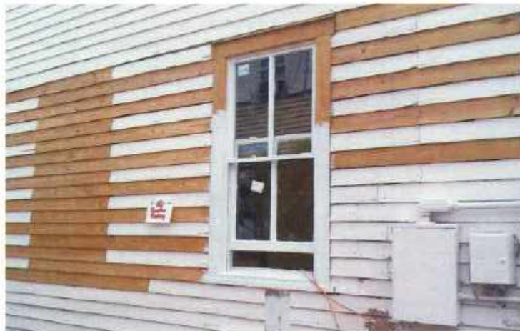
(B) Rotted clapboards have been replaced selectively with new wood siding to match the originals.
