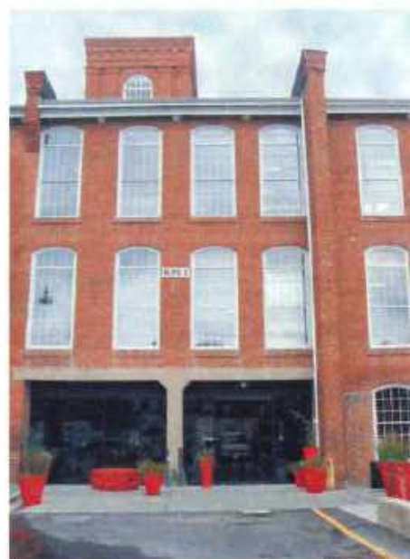
(25) The new (left) designs for the garage door openings in this commercial building (a) converted for restaurant use and in this mill building (b) rehabilitated for residential use are compatible with the historic character of the buildings.
