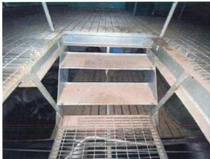
Figure 3: Open grate floor and stairs
