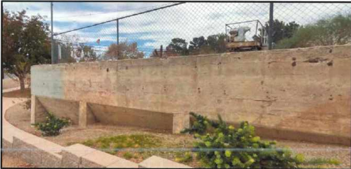
Figure 30 – Concrete Damage at Top of Walls
