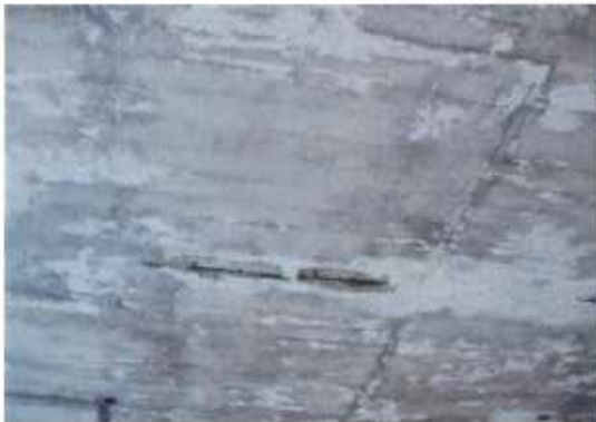
[5] Rebar in the reinforced concrete ceiling have rusted, causing the concrete to spall. The rebar must be cleaned of rust before the concrete can be patched.
