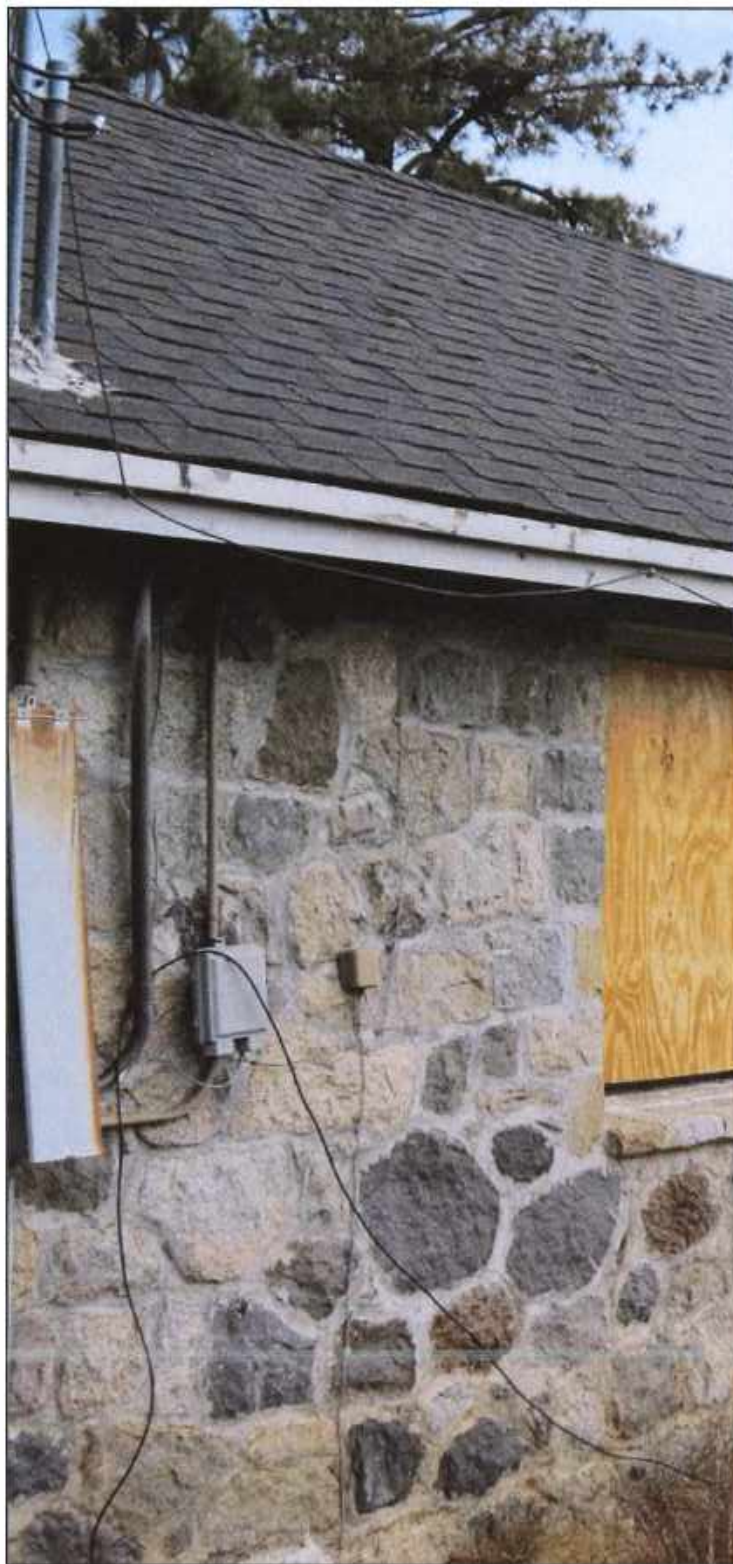
Figure 10 In several areas, cement has been used to repair the mortar joints. The example shown here is on the south elevation next to the bank of four windows (facing northeast).
