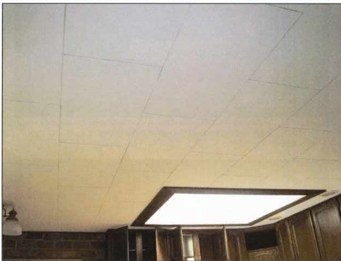
Figure 24 The interior of the school room was modified with a drop ceiling and a skylight over the kitchen.
