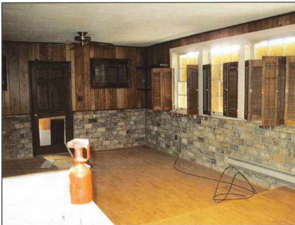
Figure 18 The interior of the school room (facing southeast). The original bank of windows remains, but the interior walls have been covered in artificial brick and wood paneling.
