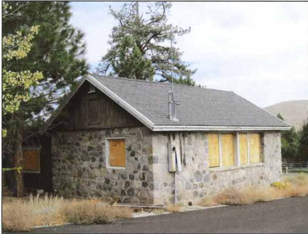
Figure 13 The main source of light for the school room was the bank of four windows on the south elevation. In keeping with the school standards of the day, the light from the windows shone on the students' left (facing northwest).
