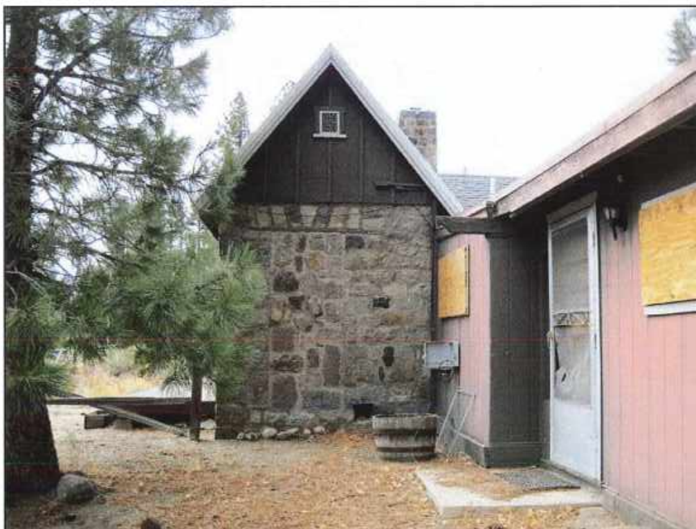
Figure 12 The north elevation of the wing showing the door filled in with local field stone. The front elevation of the c. 1980s addition is on the right (facing south).
