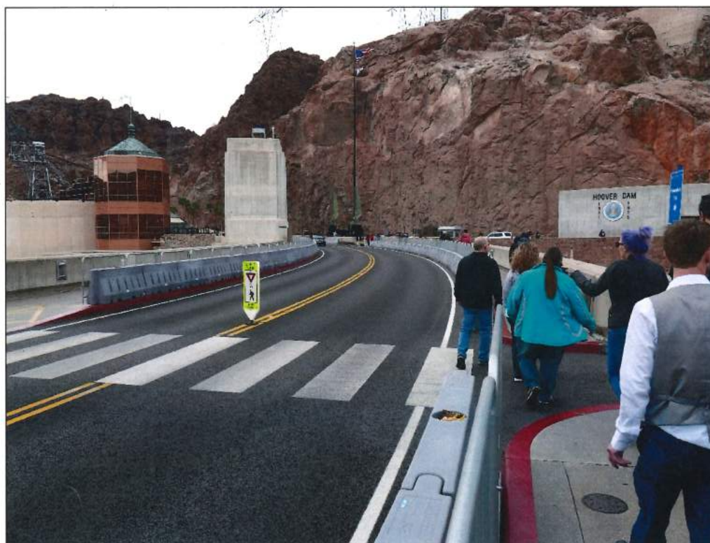
Figure A.5. Currently installed Jersey barriers, fencing, and crosswalk at Hoover Dam.
