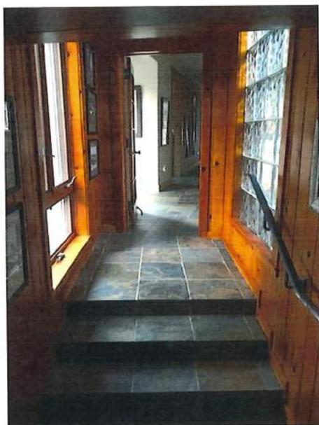
*Connector Interior. Glass Block and Ceiling Leaking. Window unit on left has failed.*
