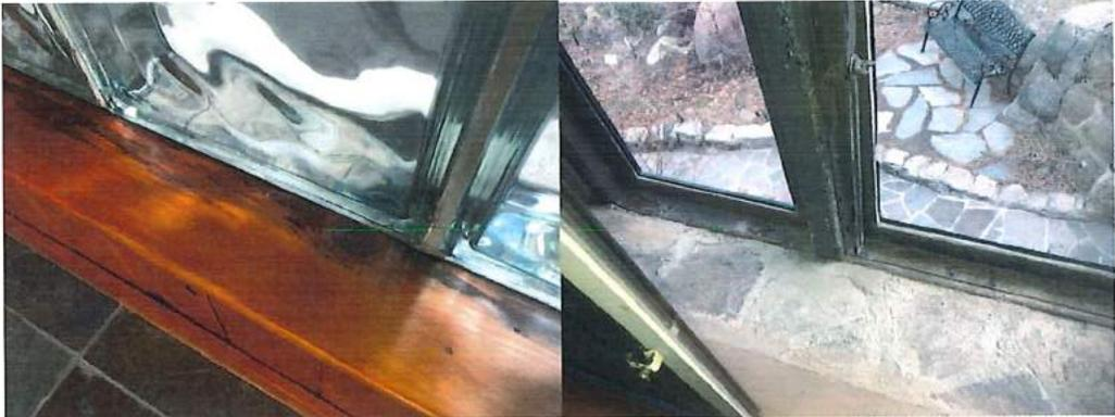
*Water seepage under 1930s glass window block onto sills.*
