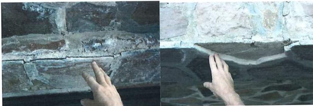
*Failing masonry on underside of upper balcony due to water penetration.*
