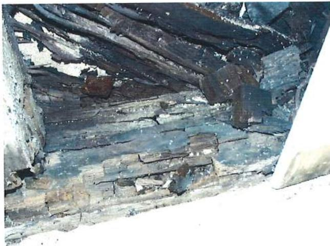
*Opening-up the space beneath the leaking Old Lodge Door units reveals extent of damage.*
