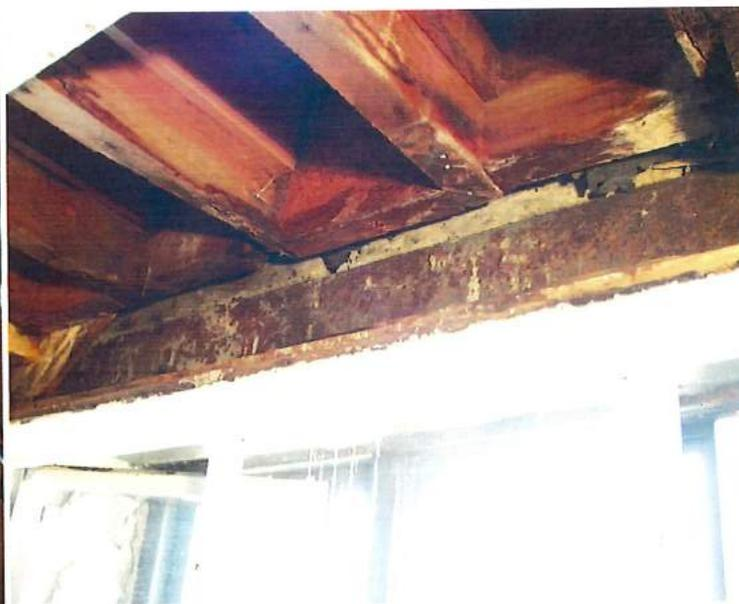
*Opening up the spaces below reveals extent of water damage, including rot.*
