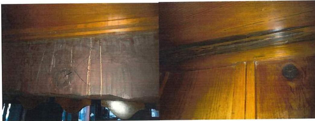
*Water Passes Through Balcony Stone to Interior Spaces, below. Mold and Mildew is forming, not to mention what we will find in spaces behind the wall and ceiling boards.*
