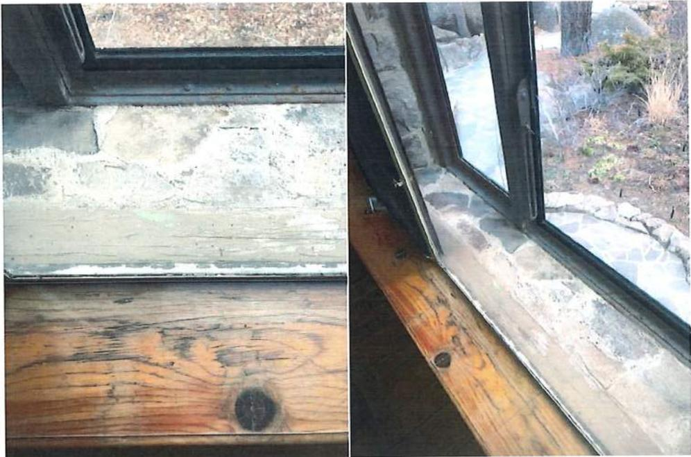
*Close-up Detail of Air-Gap Area. Note grout will require replacement.*
