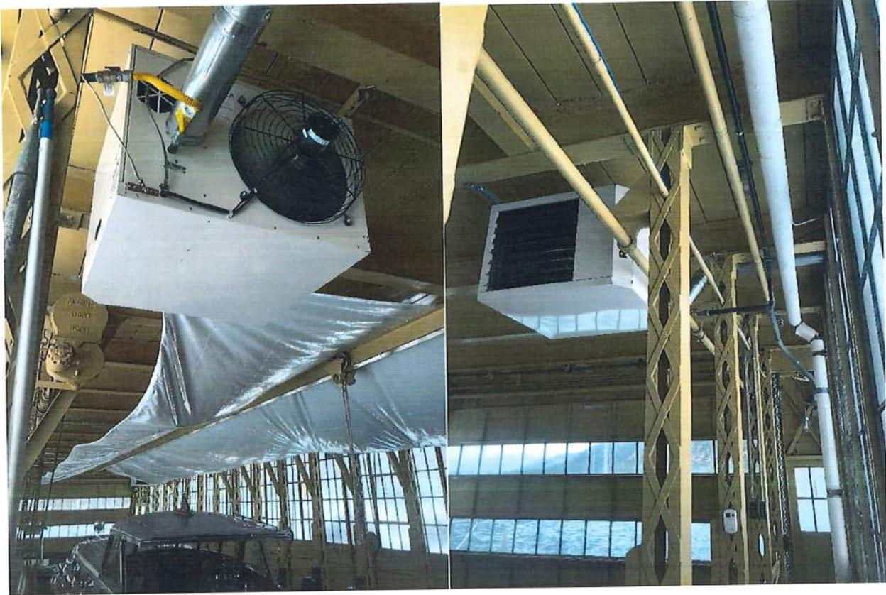
***Plimpton Installed Dual State-of-the-Art Reznor Units with new electrical, gas supply, and venting, while Nevada 36 Companies Inc. supplied material and installed hangars, conduit, and control circuits.***
