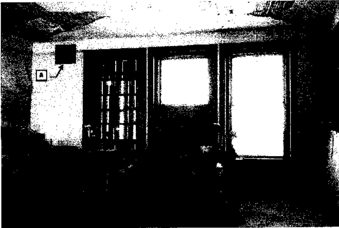
Image 51: Room 8 view north. (A) North wall upper fresh air gravity vent.
