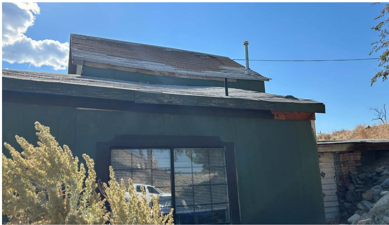
STRUCTURAL ROOF FAILURES
