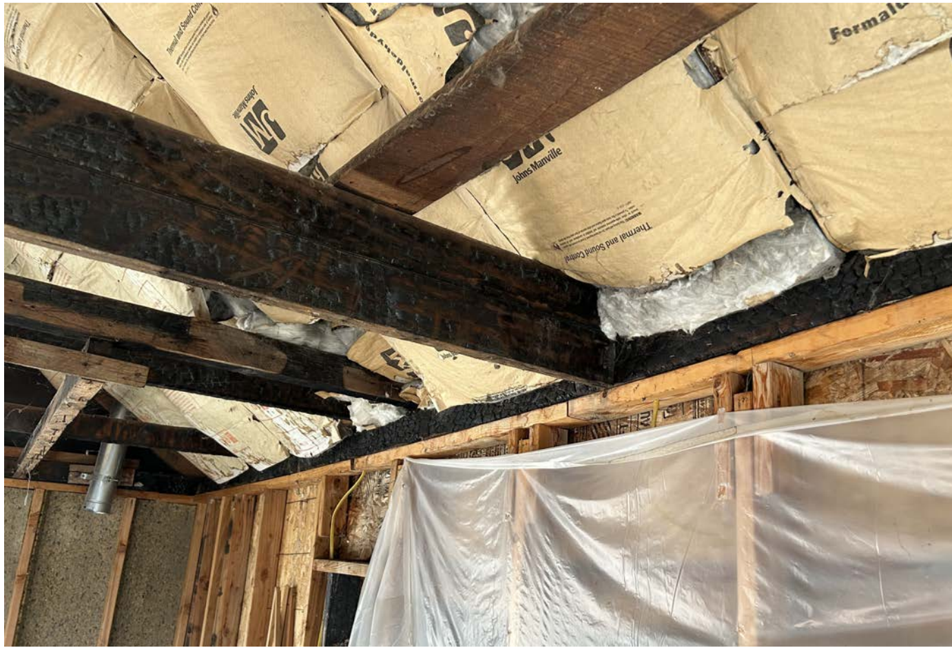
EXISTING FIRE DAMAGE @ ROOF STRUCTURE
