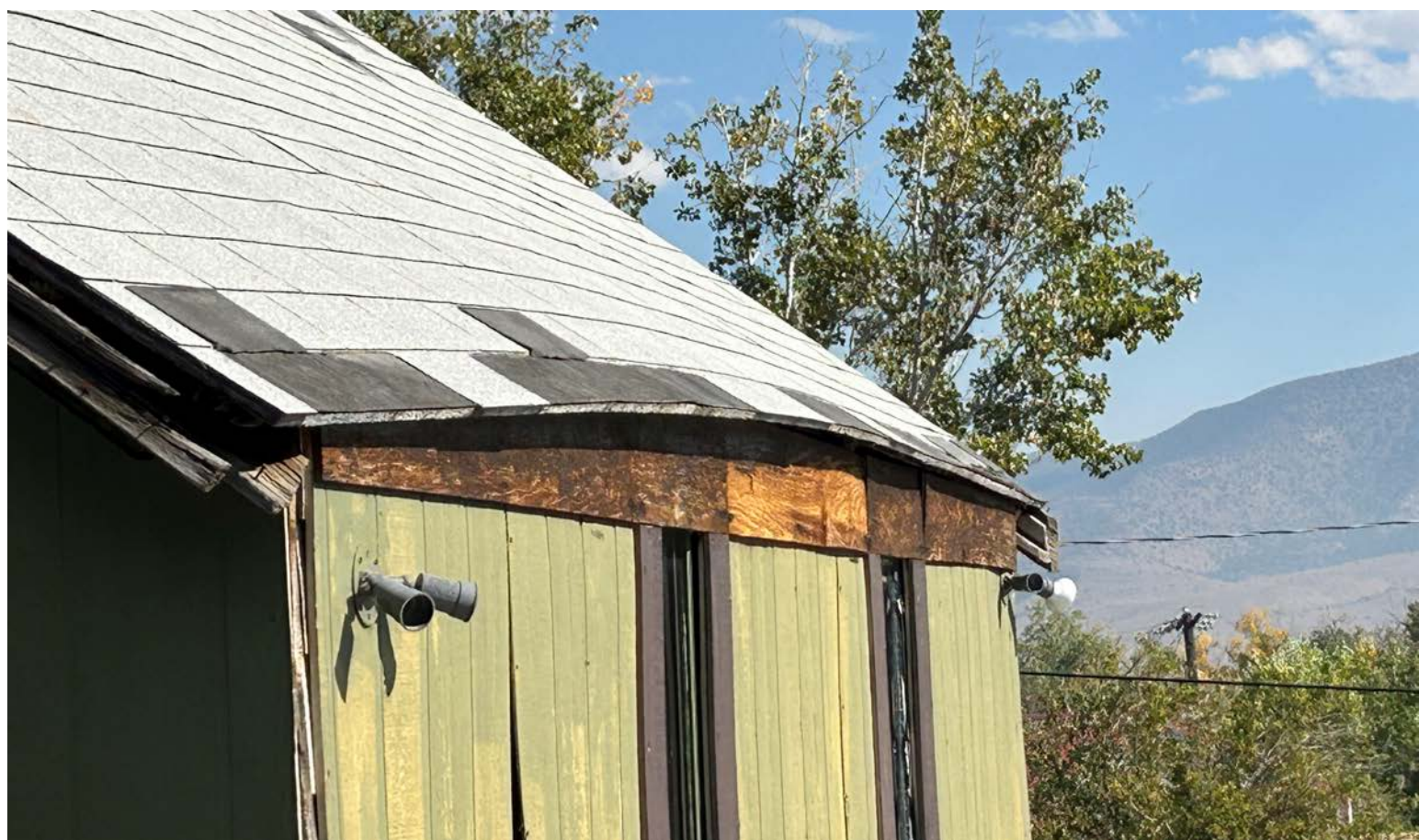
STRUCTURAL ROOF FAILURES
