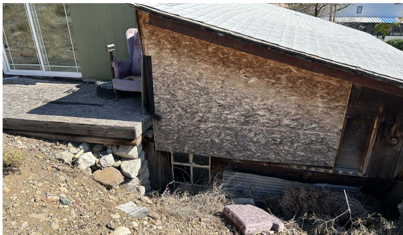
EXISTING COLLAPSED REAR SLOPE ONTO BUILDING
