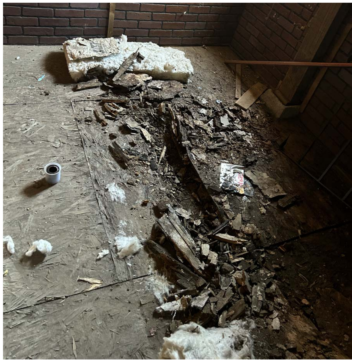
SUBFLOOR DIRECTLY ON DIRT
