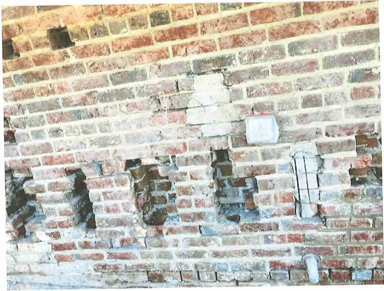
Open Holes where beams connected to old building
