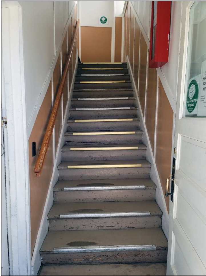
This is the staircase to the second floor of the Transportation Building. The staircase was installed in 1910 and has developed list away from the wall. This is the only access to the second floor of the building.
