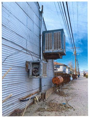
This is one of the swamp coolers hanging off the side of the building currently. These will be replaced with new and working systems.
