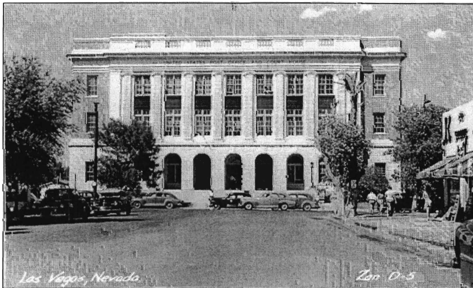
Figure 2: View of USPOCH from Third Street c. 1940.
