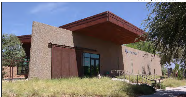
Figure 15: Visitor Center facing northwest.
