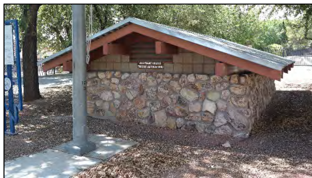
Figure 11: Modern pumphouse building facing south.
