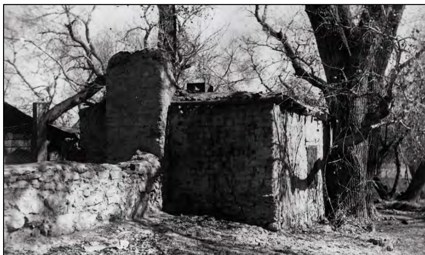
Figure 28: Fort remnant with chimney pictured in 1929.
