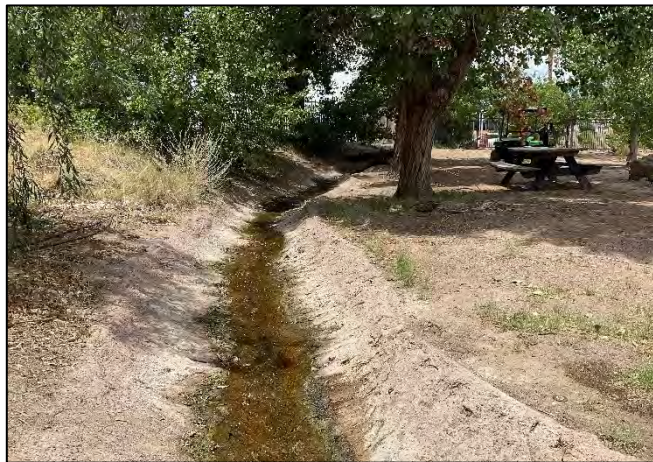
Figure 17: Creek reconstruction facing west.
