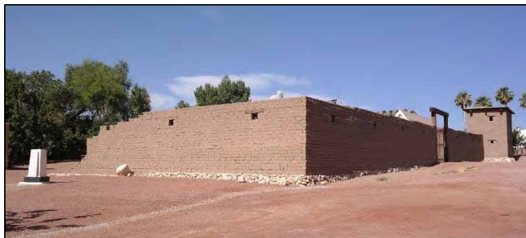
Figure 7: Overview of fort reconstruction looking southwest.
