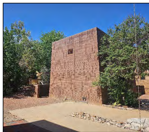
Figure 12: Restroom Building 1 facing southwest.
