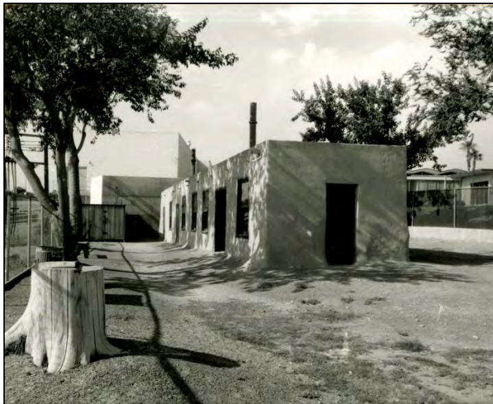
Figure 36: Adobe building with new mud plaster pictured in 1992 (Old Las Vegas Mormon Fort State Park).
