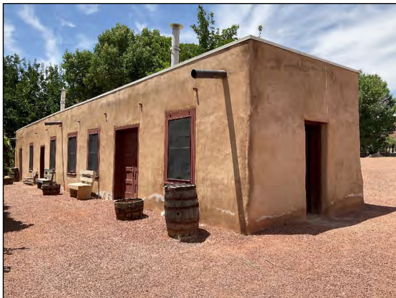
Figure 4: East and north elevations of adobe building.
