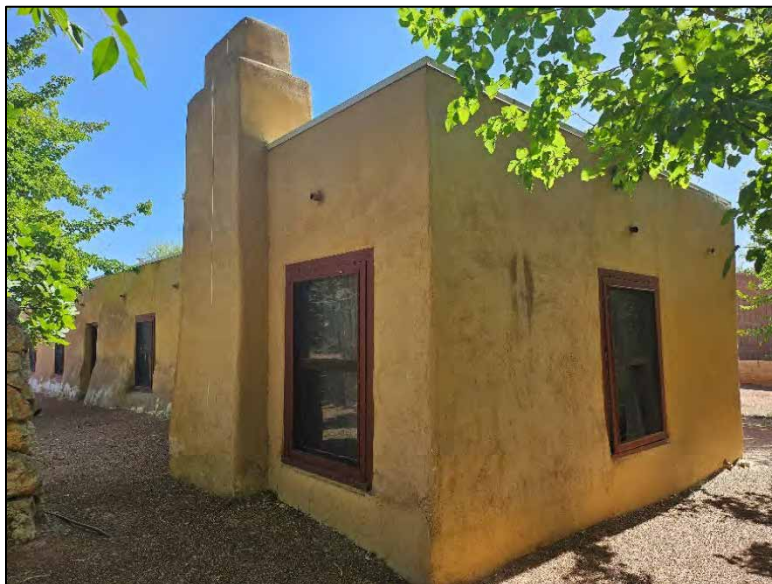
Figure 5: West and south elevations of adobe building.
