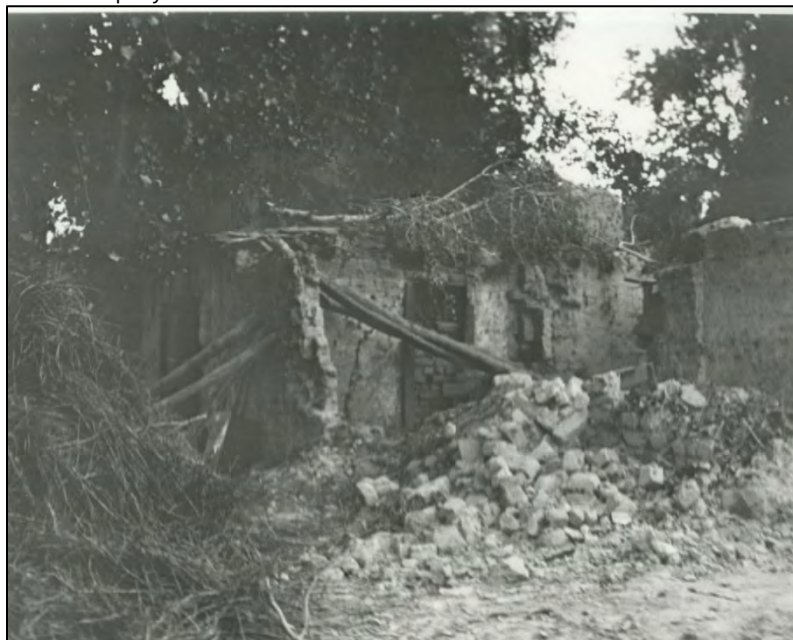
Figure 29: Braced adobe remnant in 1929 with rubble of east wall in foreground (Old Las Vegas Mormon Fort State Park).
