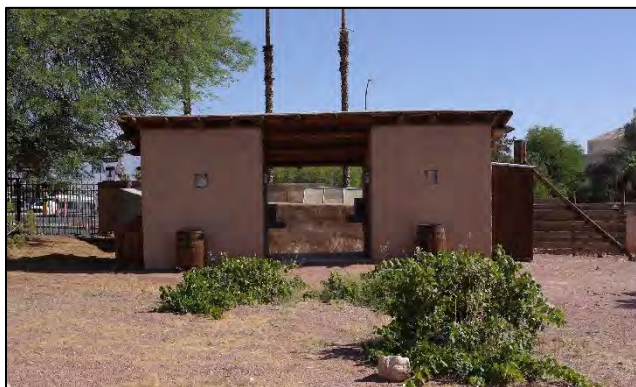
Figure 13: Restroom Building 2 facing north.
