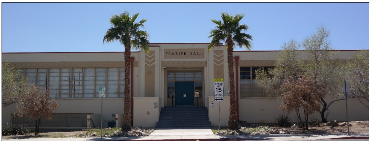
Figure 8: North Elevation of Frazier Hall.
