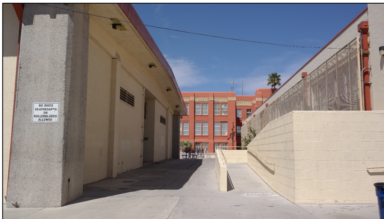
Figure 17: Northeast elevation of Cafeteria at left. Frazier Hall is at right; Main Academic Building is in the background.
