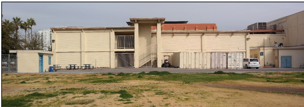
Figure 24: South elevation of Knapp Hall, viewed from the Athletic Field.
