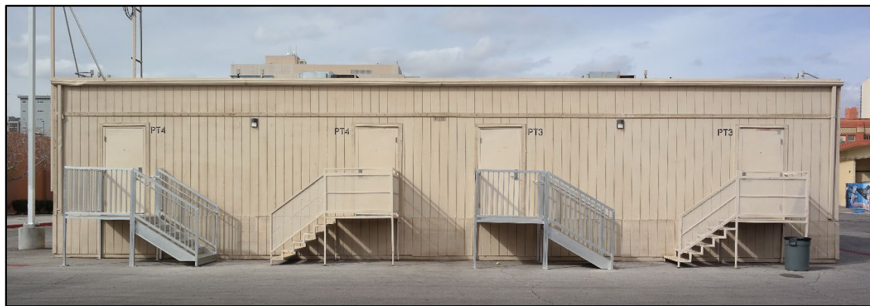
Figure 27: East Elevation of East Portable Building.
