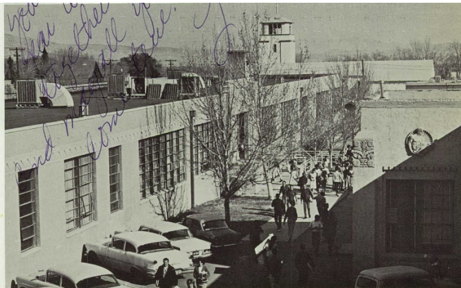
Figure 44: North elevation of Frazier Hall (left) and original shop building (right) in 1963 (Las Vegas High School Wildcat Echo).
