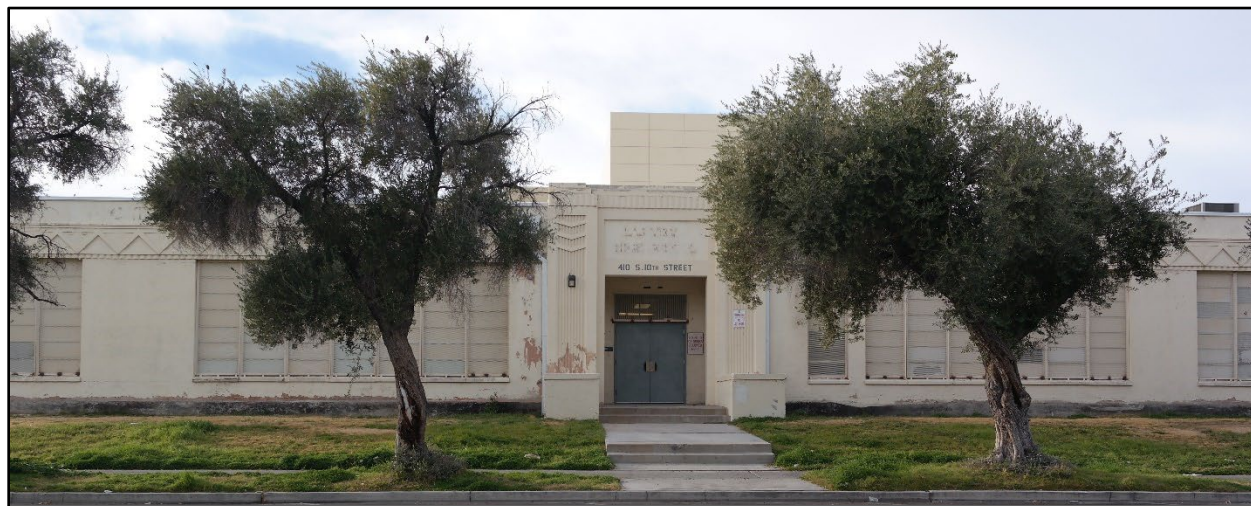
Figure 10: East Elevation of Original Vocational and Industrial Arts Building.
