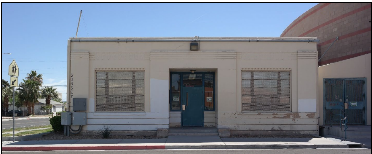
Figure 6: West Elevation of Public Schools Administration Building.
