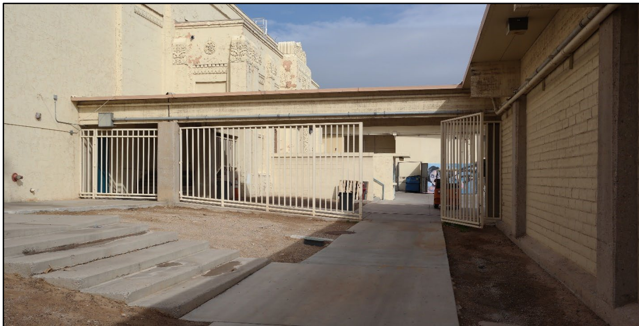
Figure 21: Breezeway between Gymnasium (left) and Locker Rooms (right).
