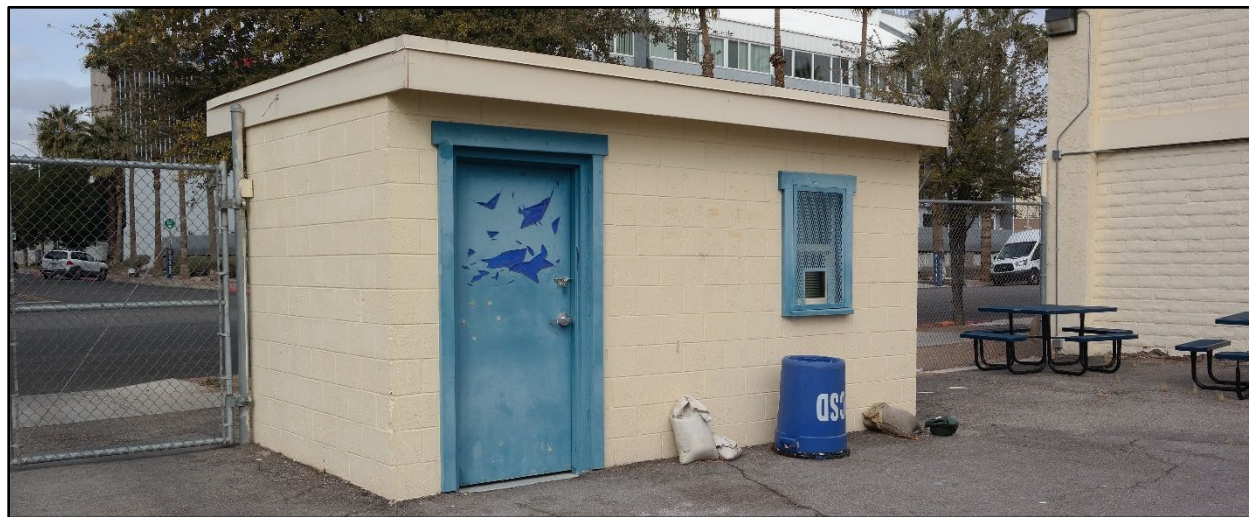
Figure 25: South and East Elevations of Ticket Office.
