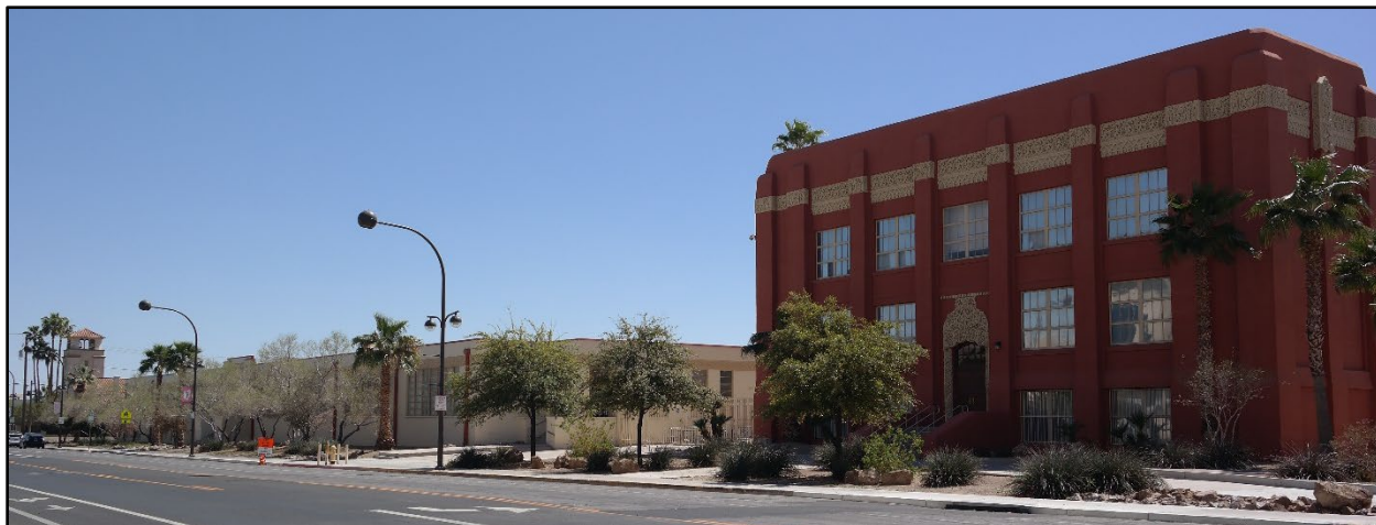
Figure 2: North elevation of Main Academic Building, looking southeast toward Frazier Hall.
