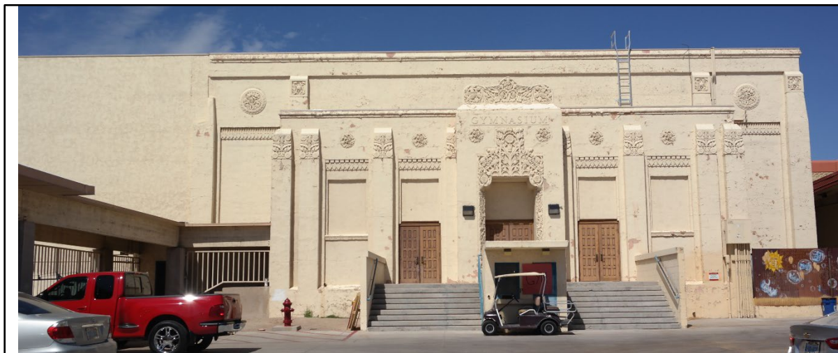
Figure 3: East Elevation of Gymnasium. Note addition at left.
