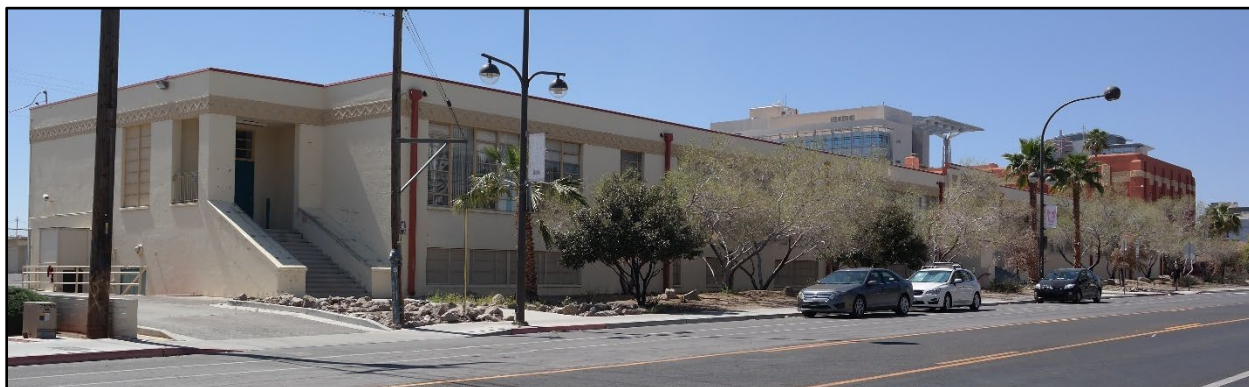
Figure 9: North elevation of Frazier Hall, looking southwest toward Main Academic Building.
