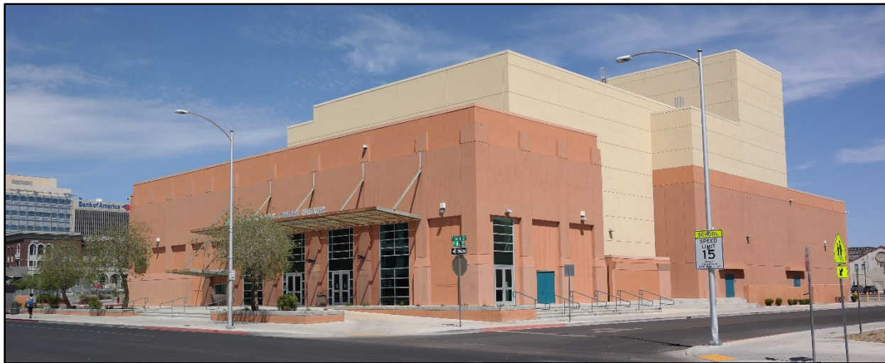
Figure 31: South and East Elevations of Lowden Theater.
