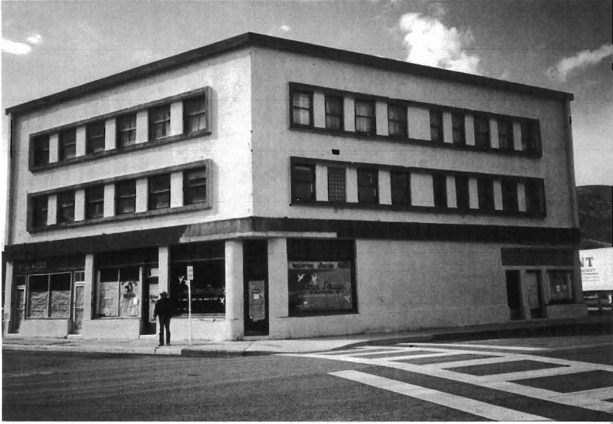
Smith-Cornelius Hotel South and East sides of building
