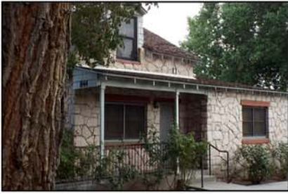
The north side and front entrance to the Wungnema House.
