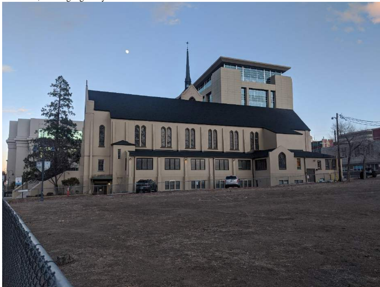
Figure 5: West elevation of Trinity Cathedral, view to east. Photo by ZoAnn Campana, January 2020.
