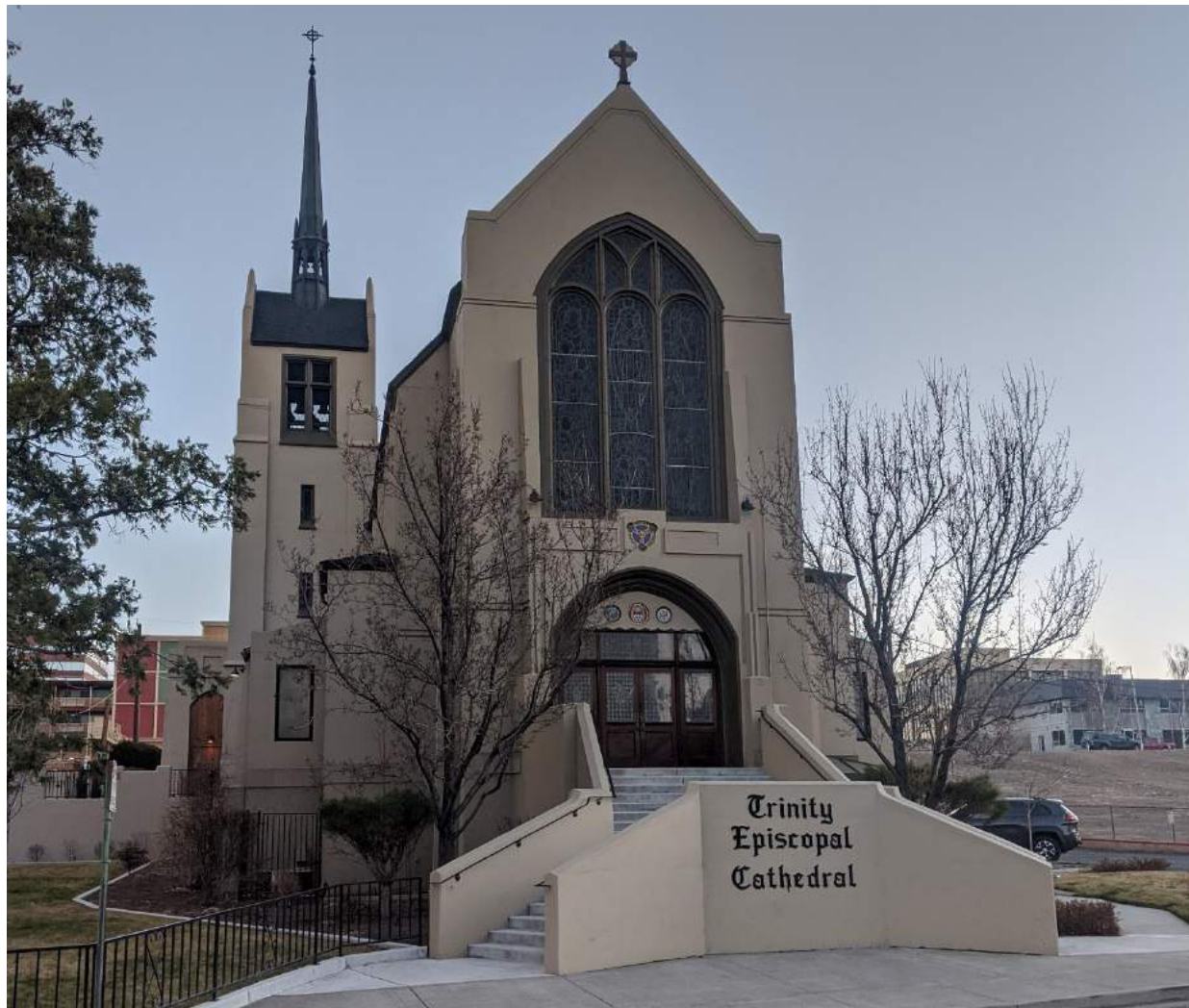
Figure 2: North elevation of Trinity Episcopal Cathedral, view to south. Photo by ZoAnn Campana, January 2020.
