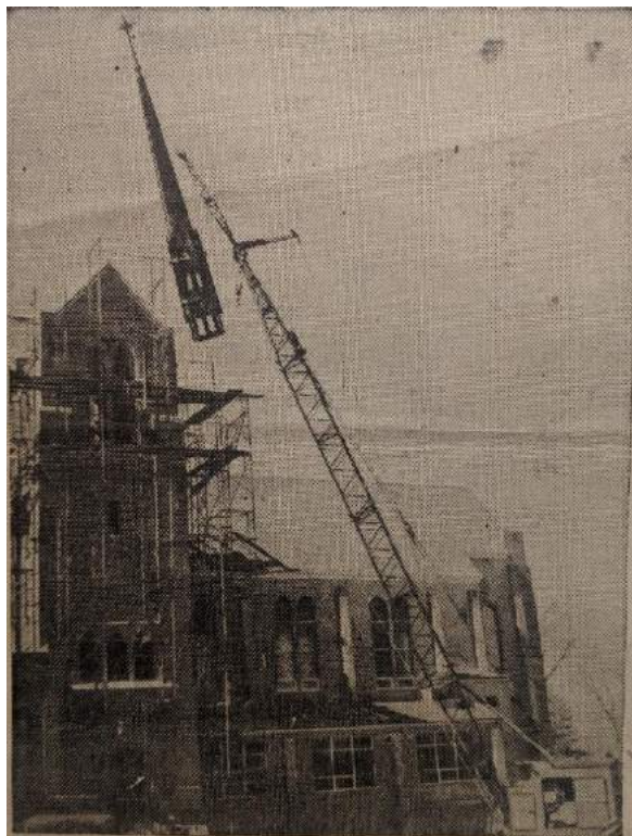
HIGHEST LIFT ever made in Reno. Hoisting into position the spire of Trinity Episcopal Church, Reno, Nevada. The operation was believed to be the highest hoist ever made in Reno. Distance from the ground to the steel beams in the tower on which the fleche rests is 60 feet. The spire itself, from base to top is 45 feet, so the distance from ground level to top is 105 feet. The fleche weighs 3,300 pounds, and its length presented problems for the crew handling the lifting operation.
