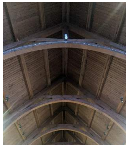
Figure 13: Trinity's trussed roof structure. Photo by ZoAnn Campana, December 2019.
