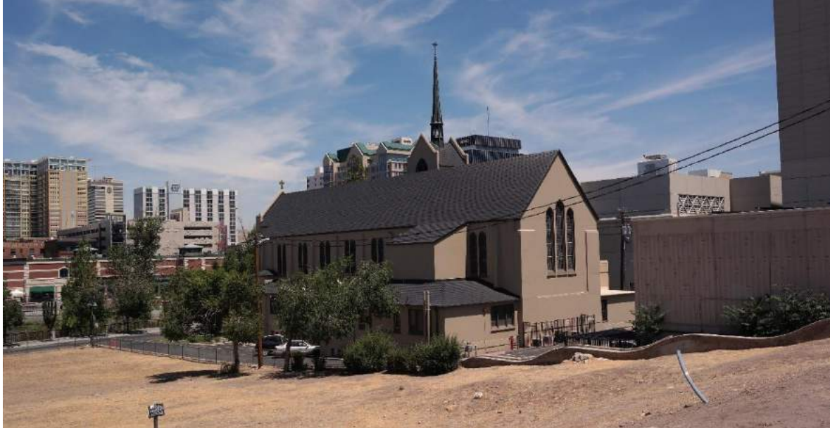
Figure 7: South and west elevations, view to northeast. Photo by ZoAnn Campana, July 2019.
