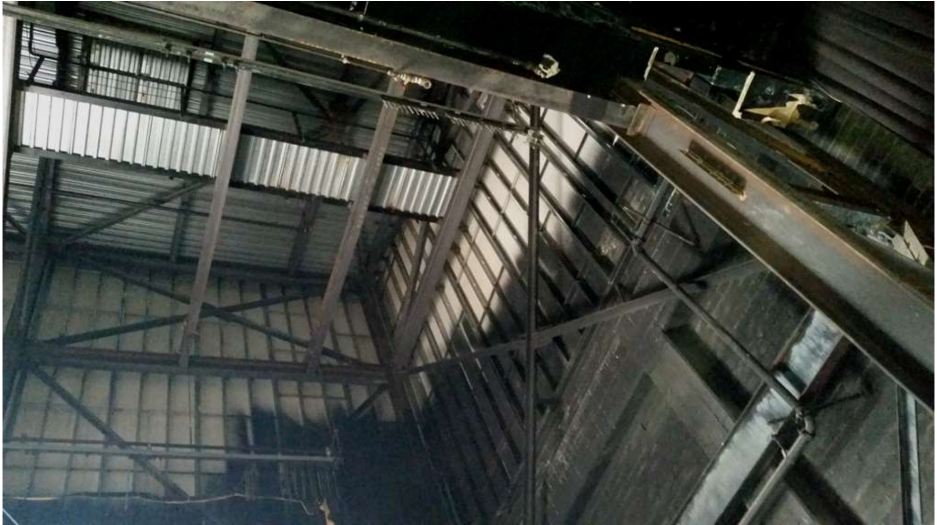
View of Fly Loft and Ceiling in Auditorium, Both Funded with CCA grants
