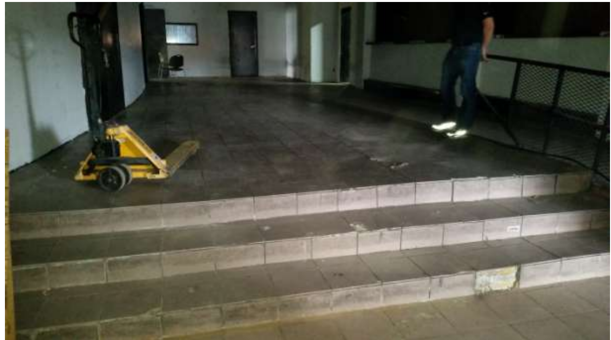
Visible in photo are broken tiles on lobby floor and stairs
