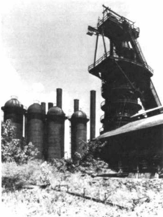
Important industrial and engineering structures should be included in the survey. In addition to their intrinsic value in the history of American industry and engineering, such structures are often associated with the economic development of a community and with its prominent citizens. The Sloss Blast Furnace Site, Birmingham, Alabama, contributed to the development of that city as the iron and steel center of the South. The site has recently been developed into a local historical park. (Jack E. Boucher for Historic American Buildings Survey/Historic American Engineering Record)
