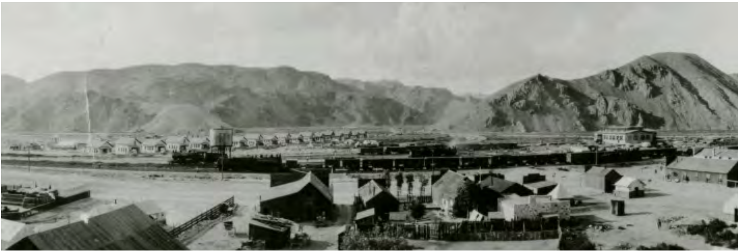
View of Caliente with row houses in background (1900-1925)
