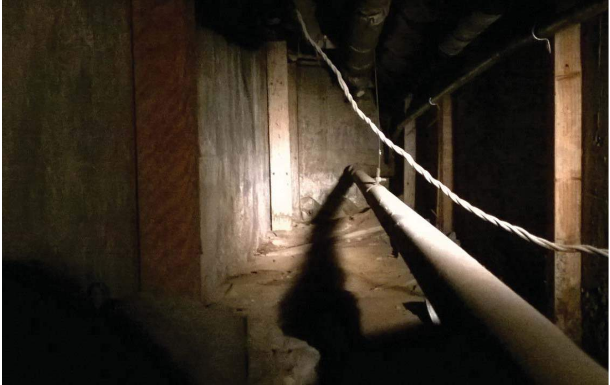
Utility line in crawlspace .
