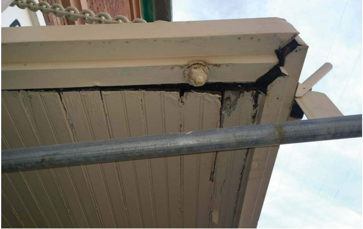
Damage to the entrance of the building.
