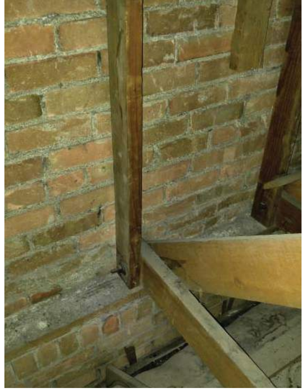
Wall to structure connection in attic space.
