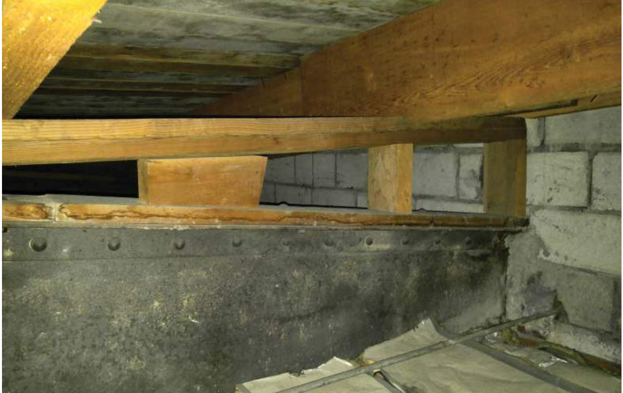
Structural truss above the firestation garage.
