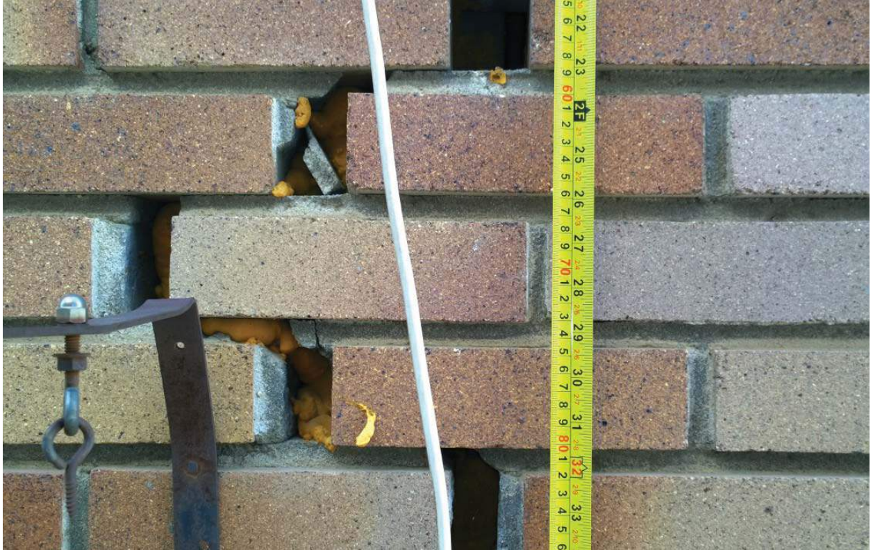
Large crack in North facade.
