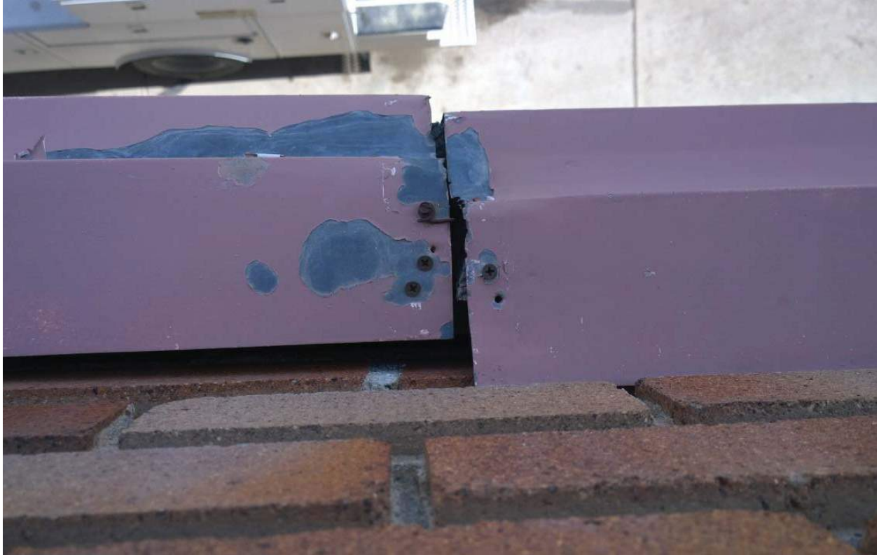
Damage to the cornice.
