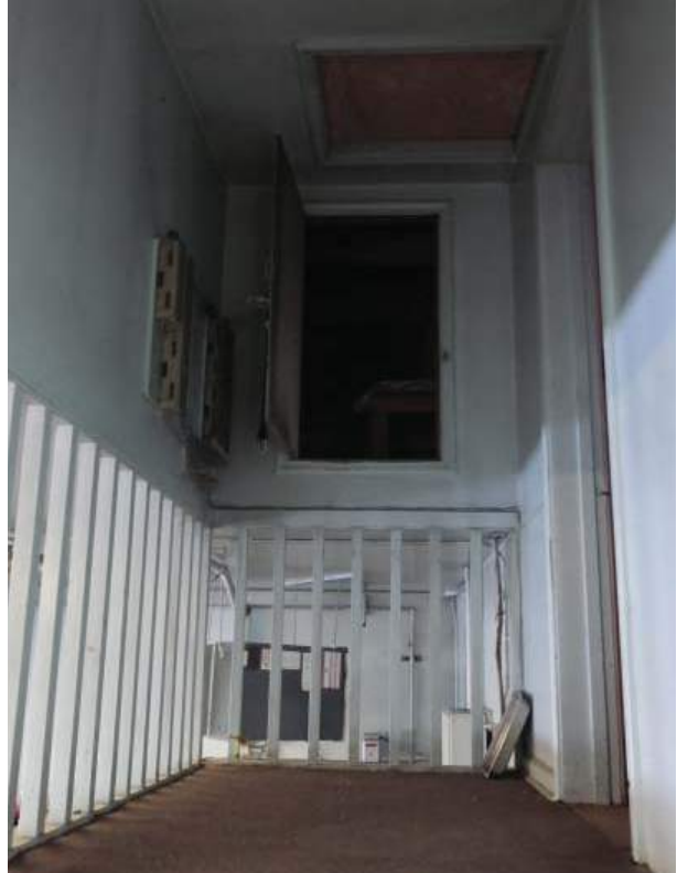
Ceiling access above firestation.
