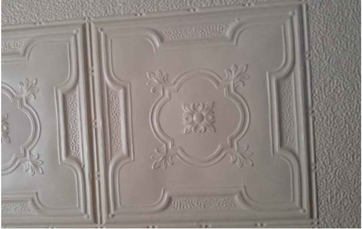
Original tin ceiling pattern detail.
