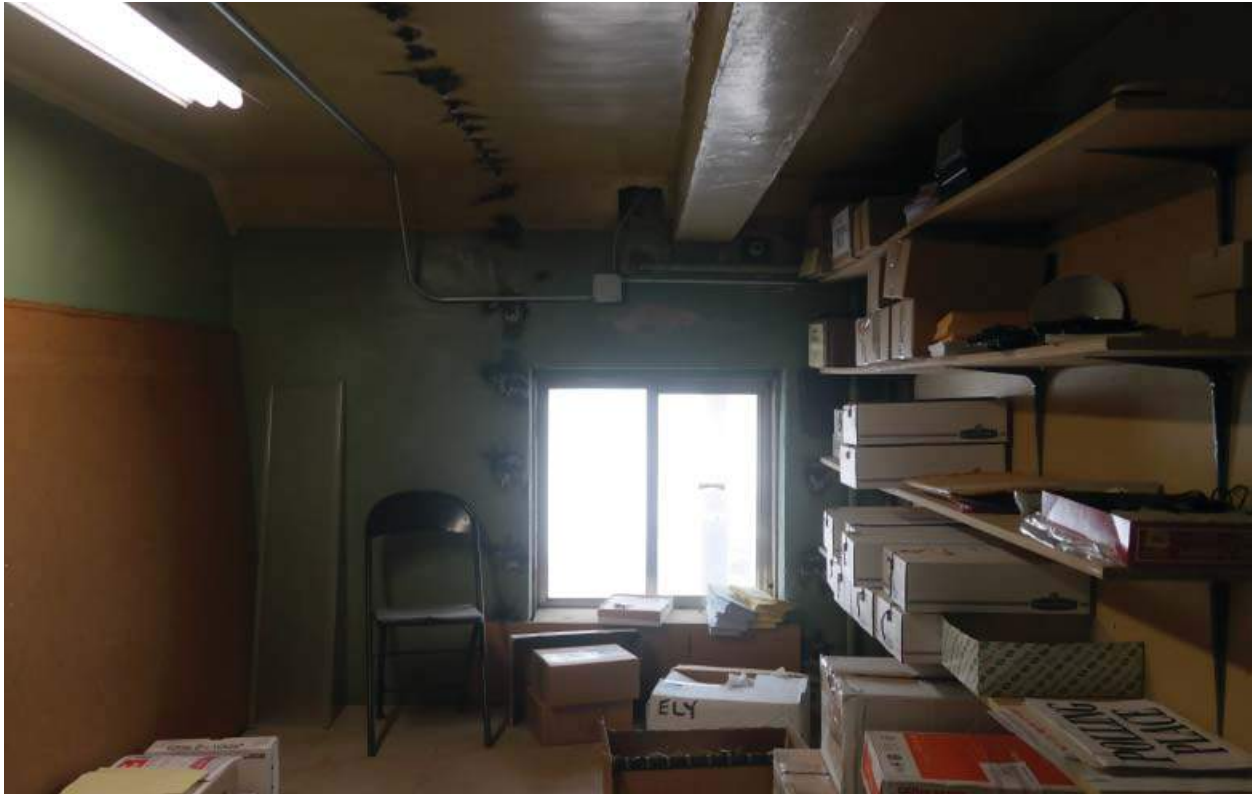
Storage on messanine level.
