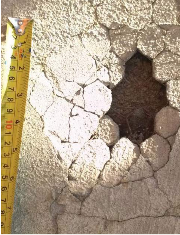
Damage to basement entry.
