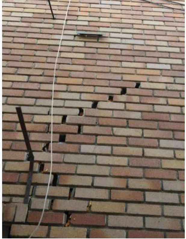
Large crack in the North facade.
