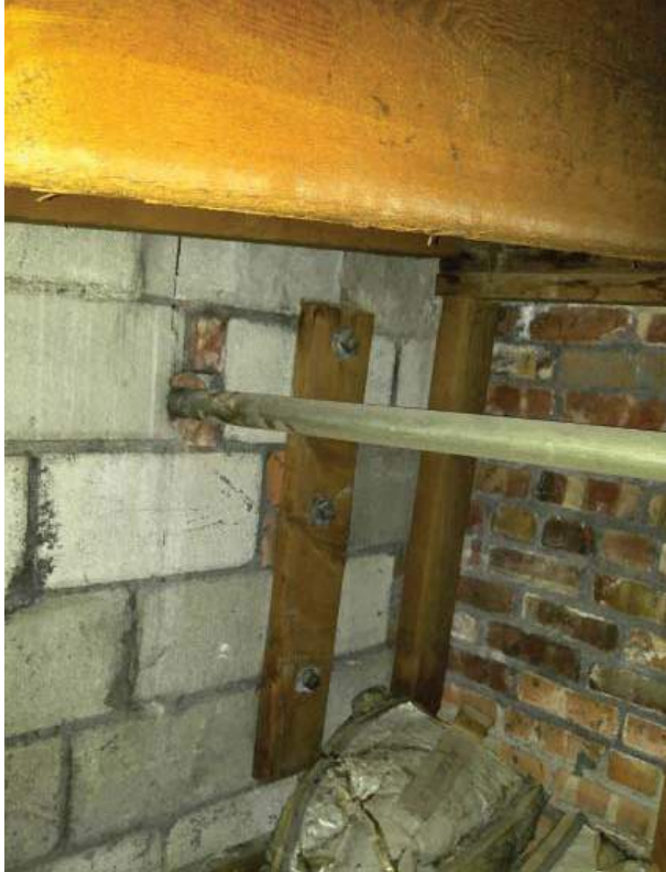
Masonry infill from previous renovation.
