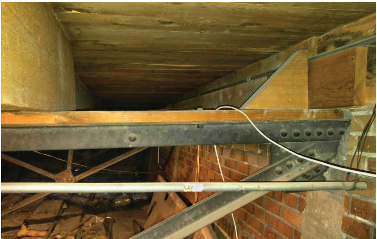
Structural truss above the firestation garage.
