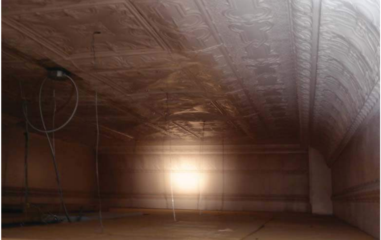
Space oin ceiling between tin ceiling and dropped ceiling.
