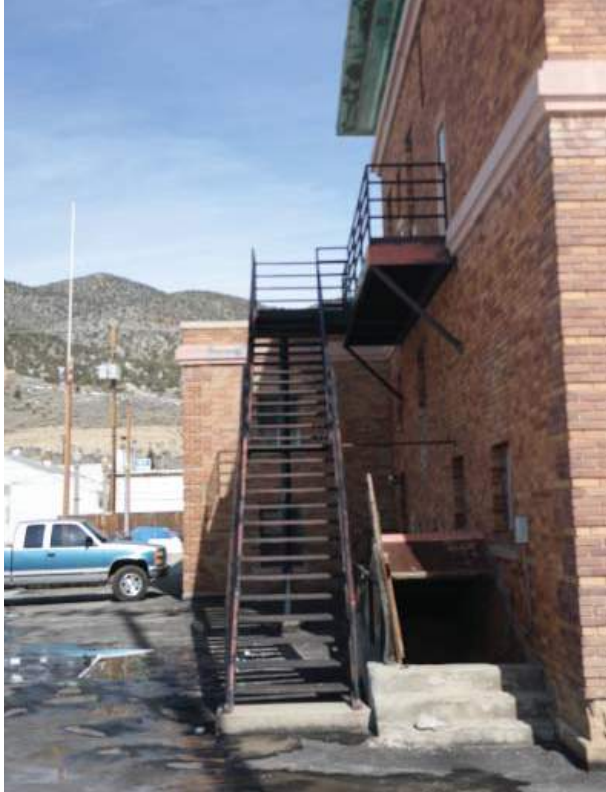
Emergency stairway behind building.
