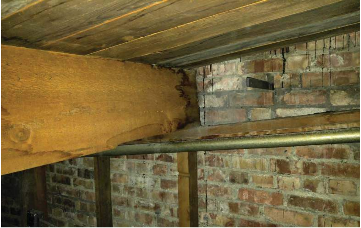
Roof to beam to truss connection.
