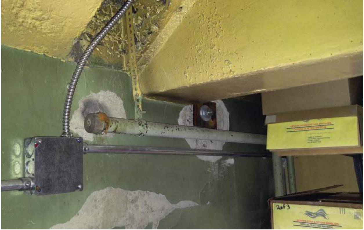
Electrical work in messanine level.
