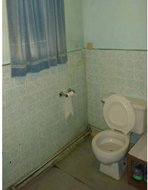
Lower bathroom in the firestation.
