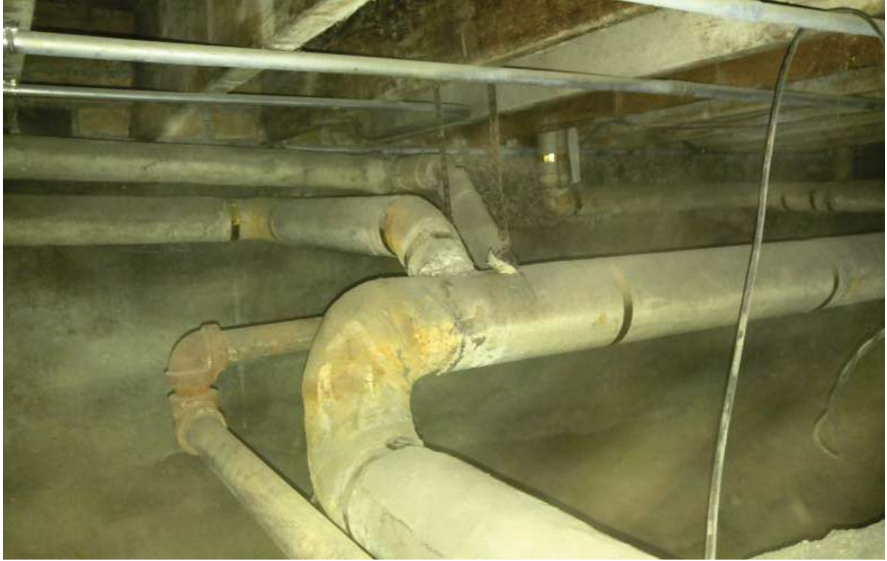
Utilities in the crawlspace.
