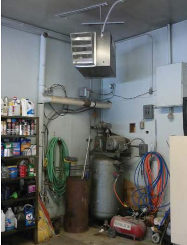
HVAC unit in firestation.
