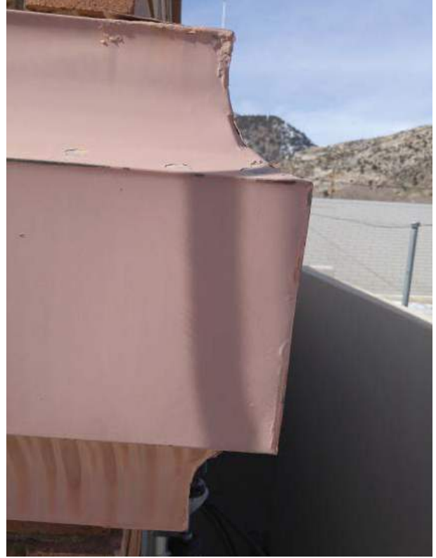
Lower cornice on the firestation.
