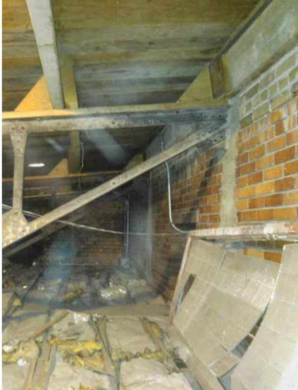
Masonry infill from previous renovation above the current firestation garage.
