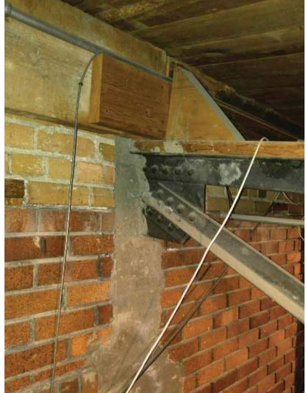
Structure to wall connection above firestation garage.
