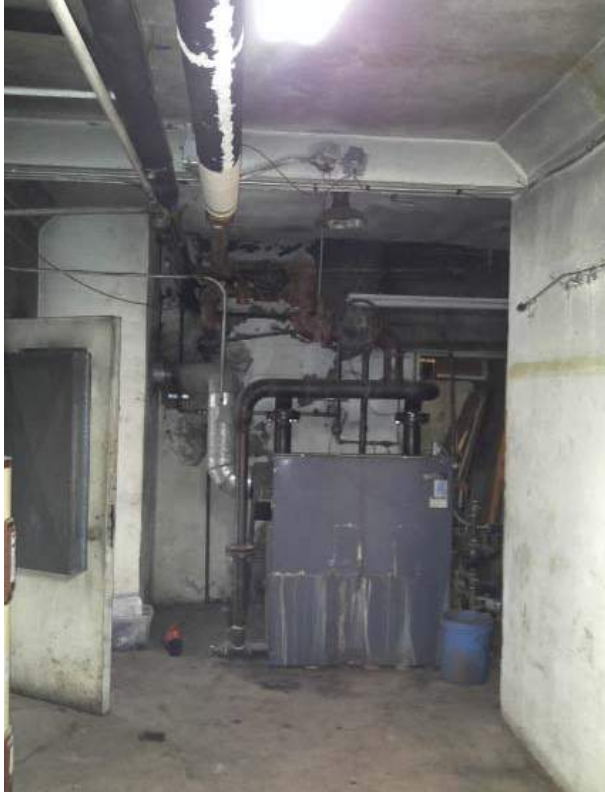
Utilities in the basement.
