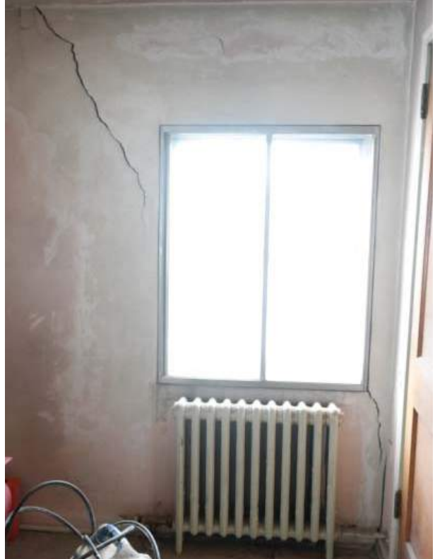
Large crack on North facade.
