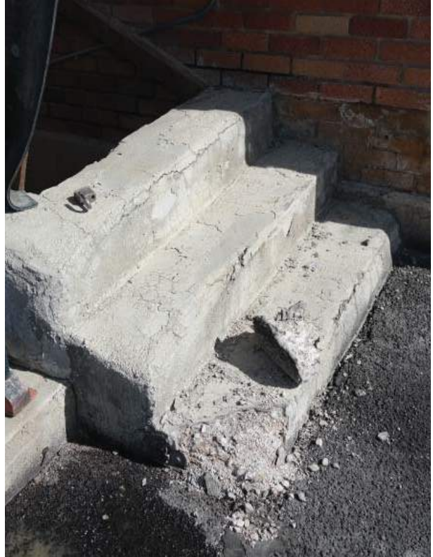
Damaged stairs to the basement.
