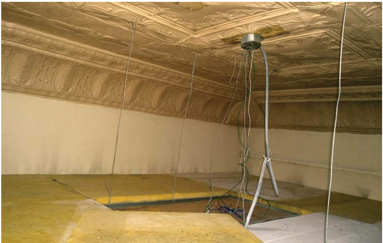
Electrical wires haging through the ceiling.
