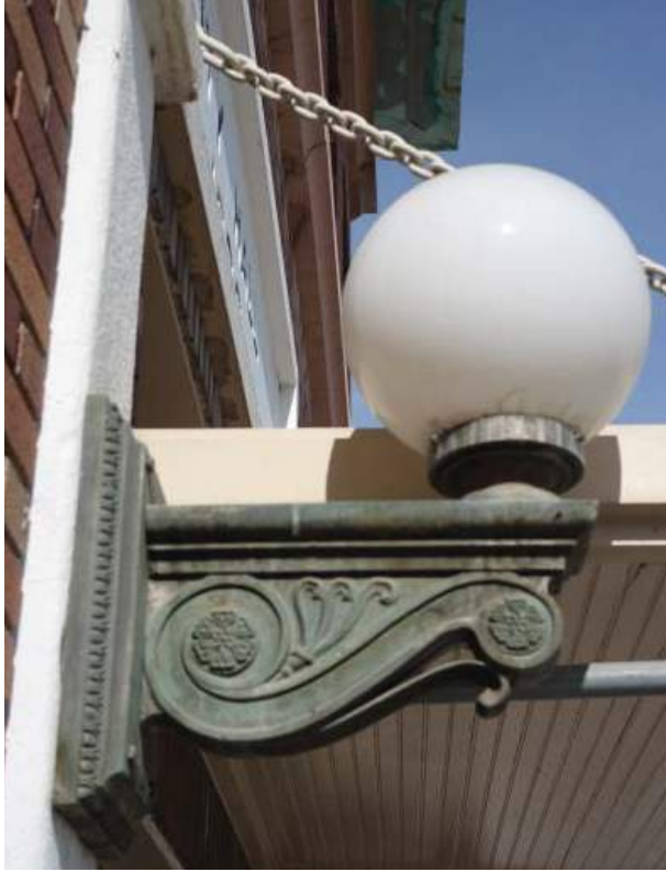
Corbel detail at entrance.
