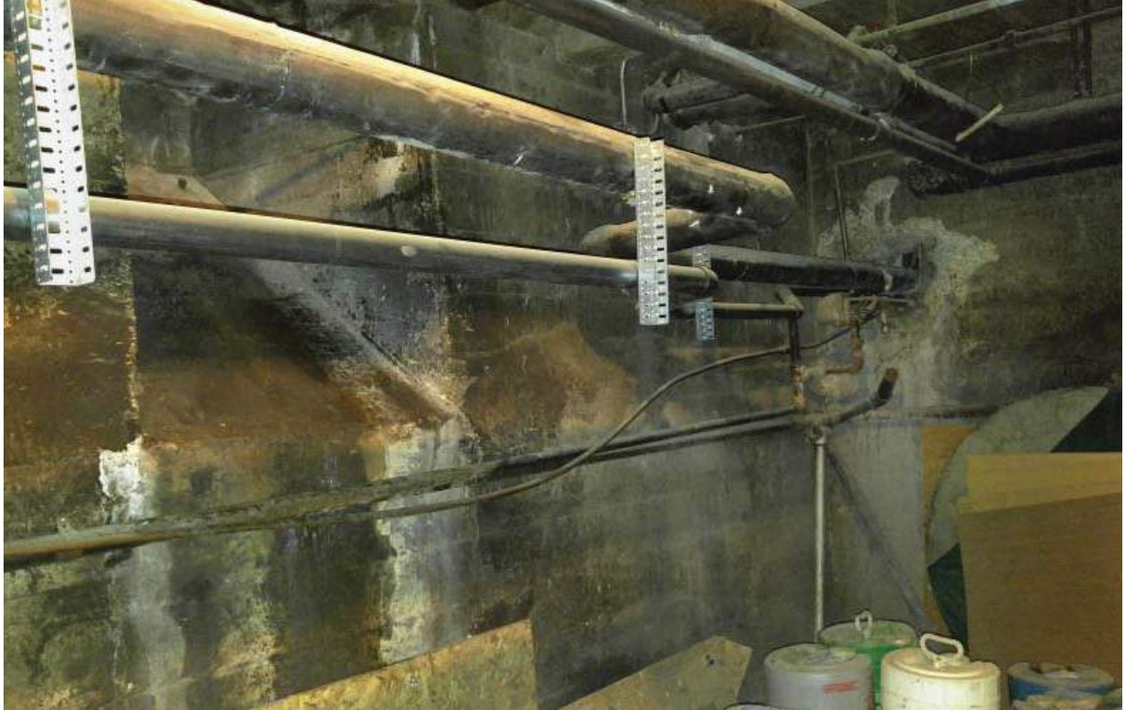
Utilities and storage in basement.
