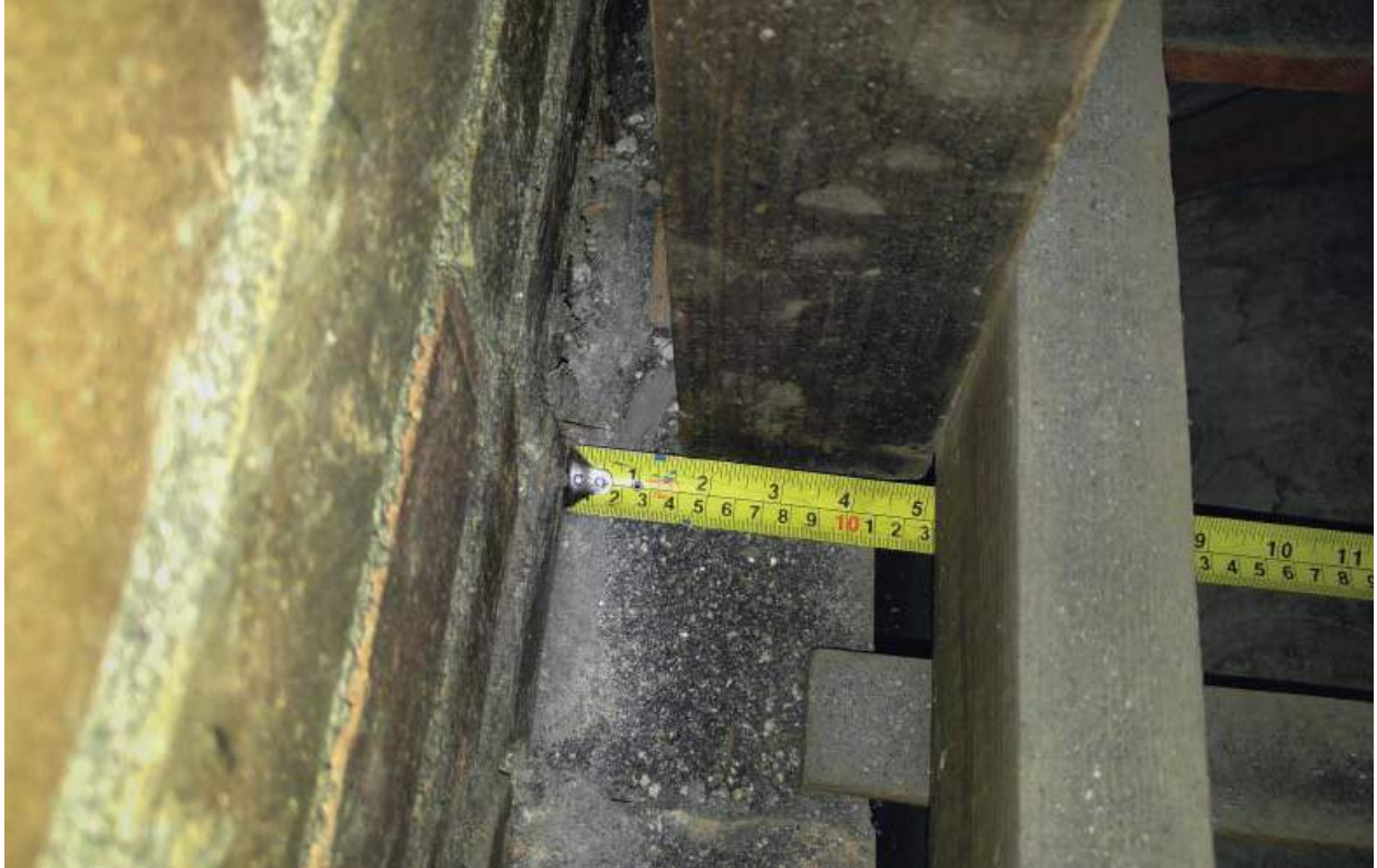
Wall to structure connection in attic space.
