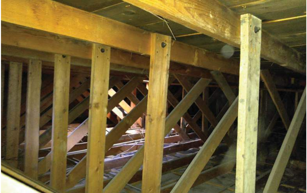
Wooden structure in the attic.
