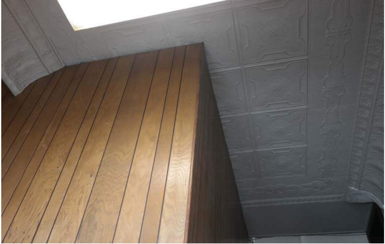
Original ceiling pattern.
