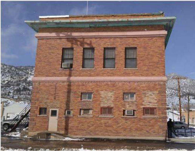
South Elevation (Notice Changes in Brick Color at Alterations)
