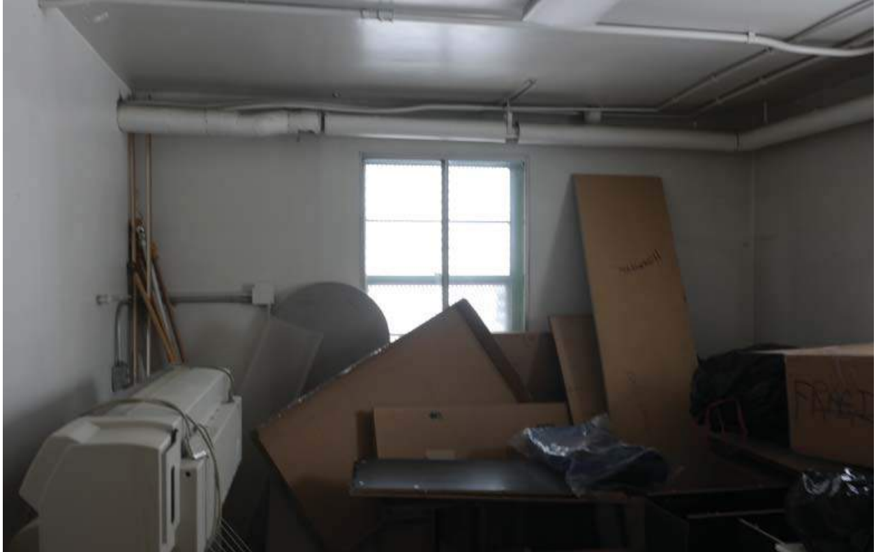
Storage are in the firestation.
