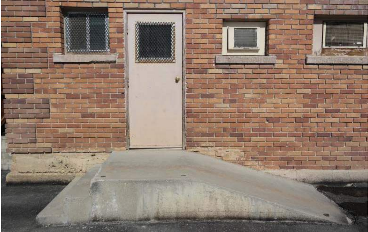
Entrance along the south elevation.
