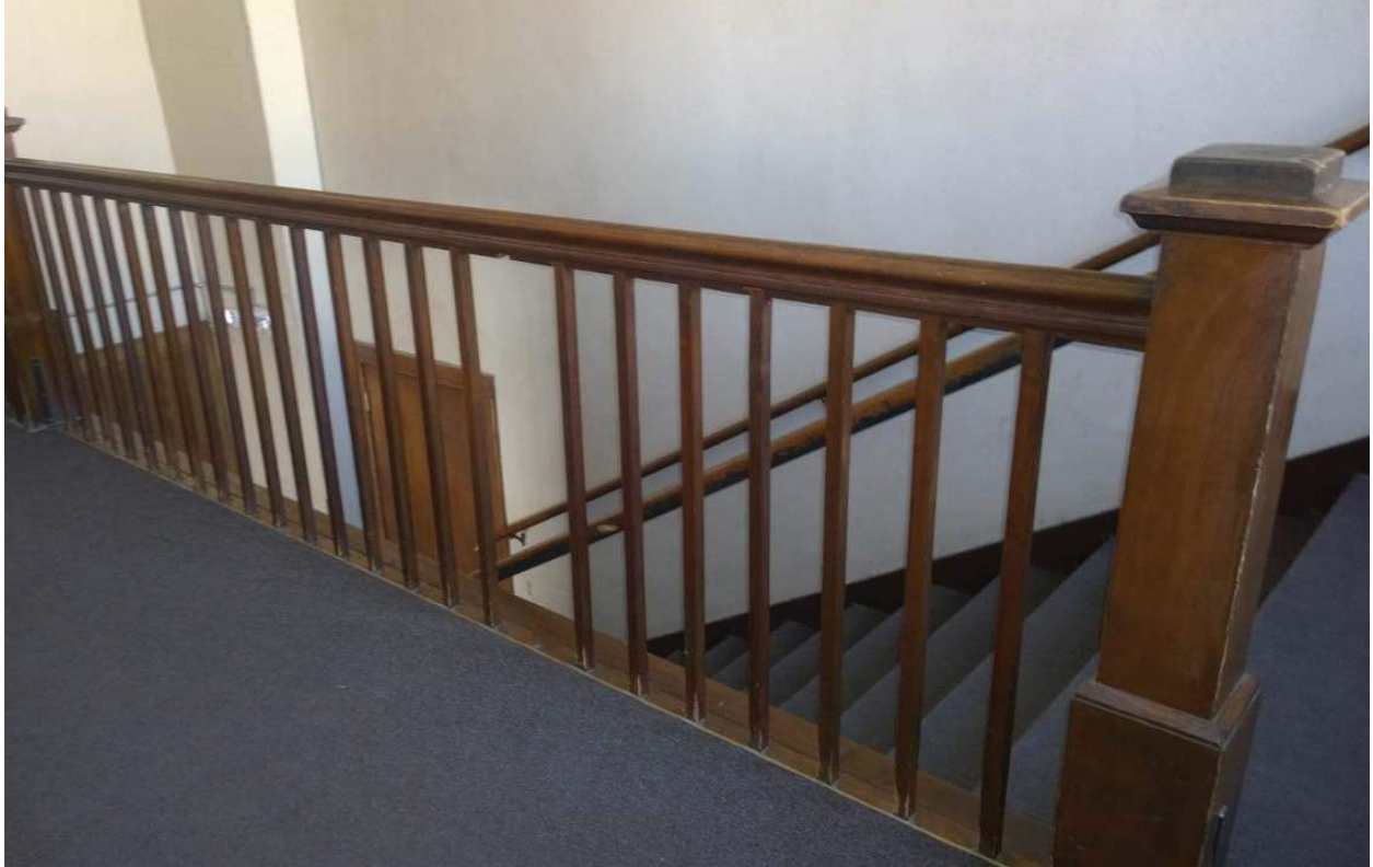
Railing on the second floor.
