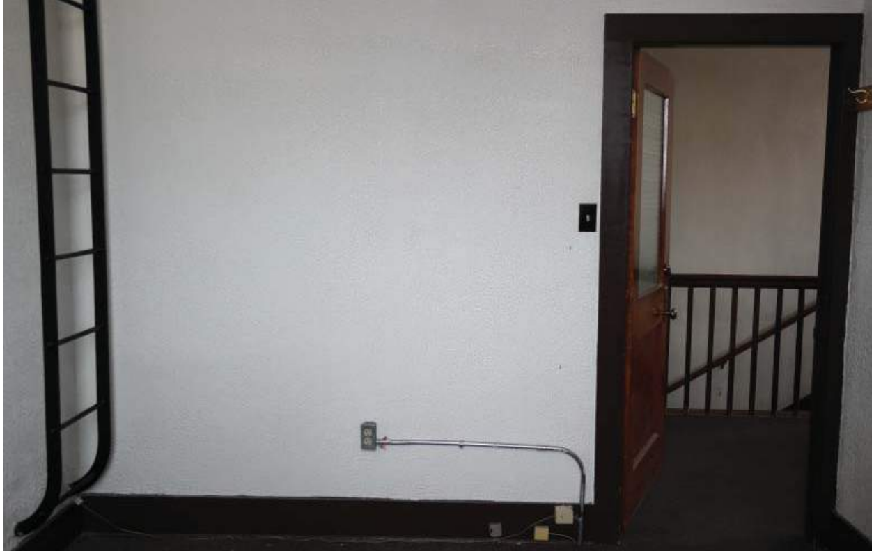
Roof access ladder on the second level.
