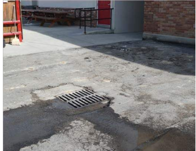
Detail of West Drain in Parking/Drive Area
