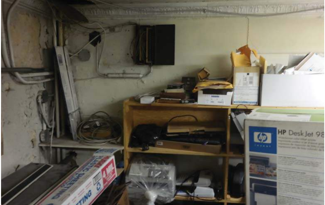
Electrical box on messanine level.
