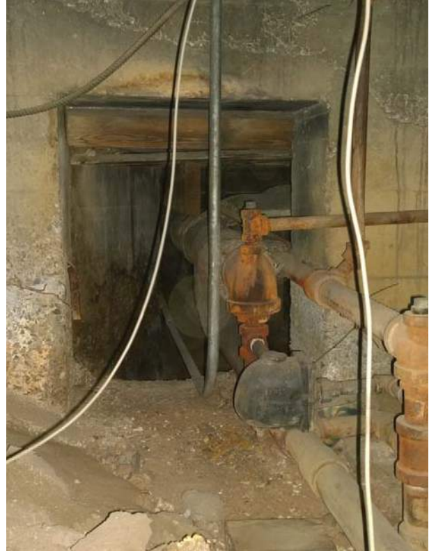
Utilities in the crawspace.
