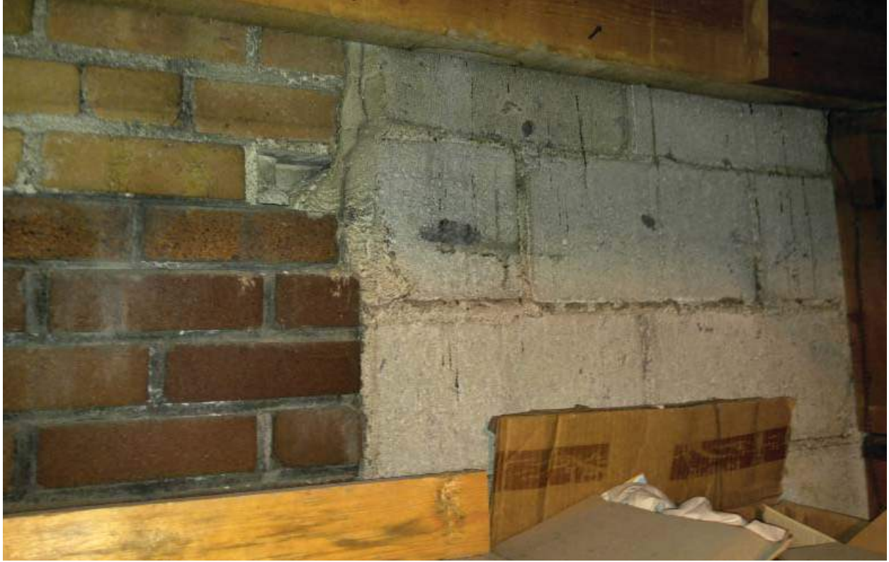
Masonry infill from previous renovation above the current firestation garage.
