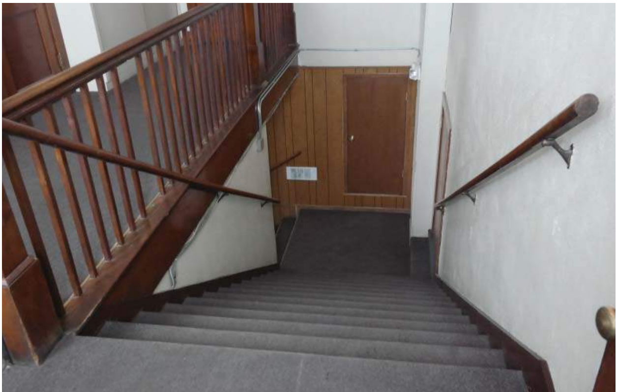
Central stairwell of the building.
