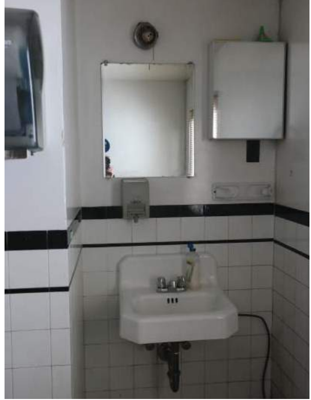
Upper bathroom in the firestation.
