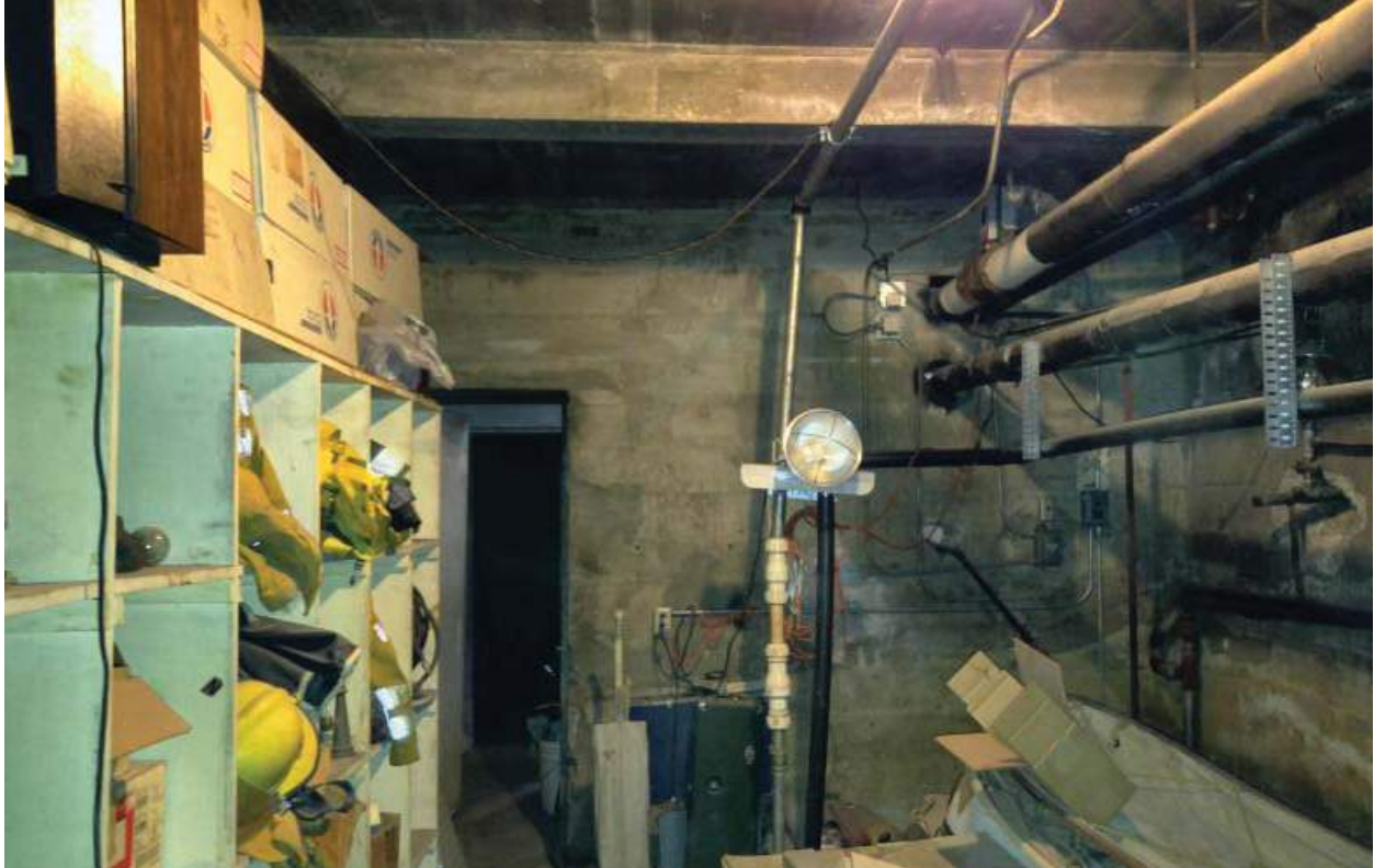
Storage and overflow pump in basement.
