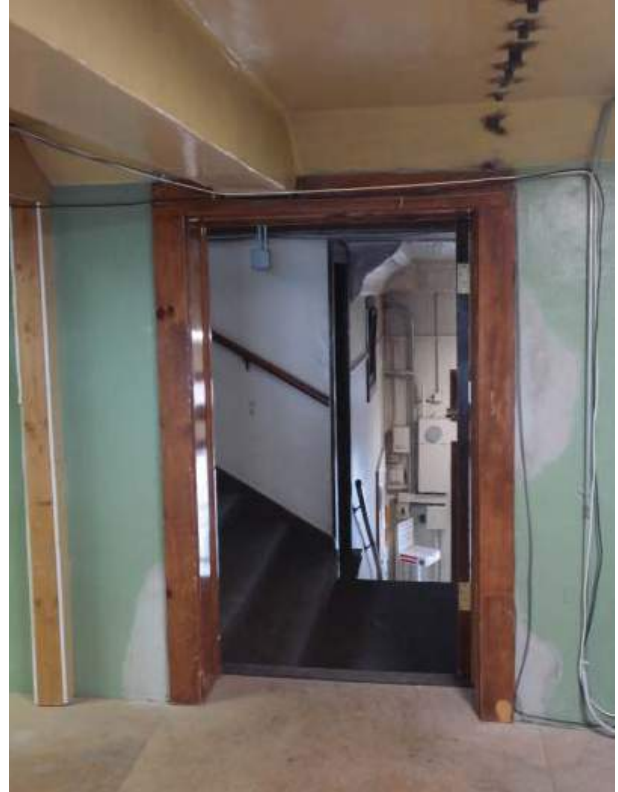
Entrance to room on messanine level.
